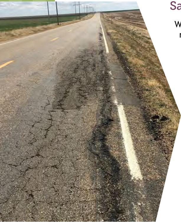
Pavement damage on US 385 in Cheyenne County
