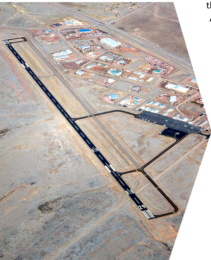
Aerial view of Fremont County airport.
