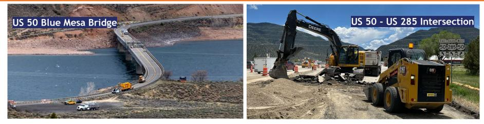
The US 50 Blue Mesa Bridge was closed between Mile Point 136 and MP 140 in April 2024 due safety reasons stemming from a crack in the high-strength steel. Repairs were conducted in phases.
