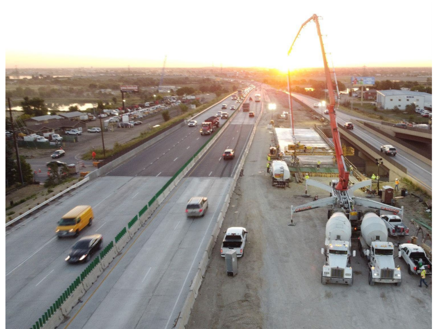
I-76 From York to Dahlia: Bridge Replacement and Concrete Pavement Reconstruction
