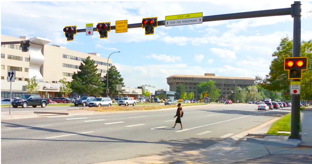
A pedestrian crosses a busy street at mid-block on Union in Lakewood west of the Federal Center with the help of a pedestrian-activated crosswalk signal.
