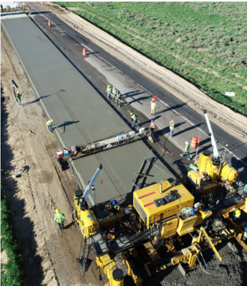
Construction on US 287 in Lamar.
