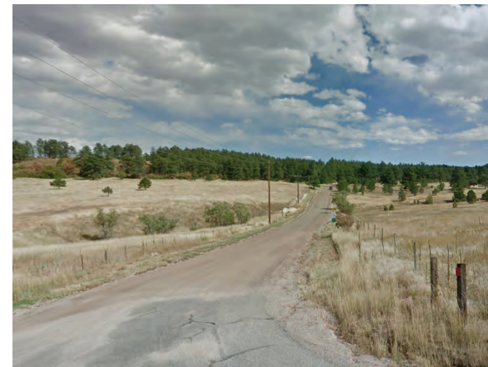
Local roads through Larkspur, like the unpaved Noe Road, are not designed to handle interstate or truck traffic. Town leaders report that cut-through traffic has increased substantially as travel delays on I-25 have worsened.
