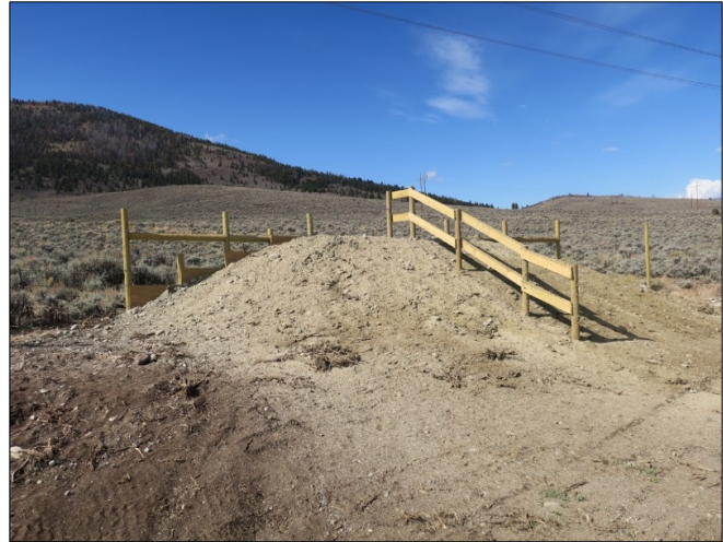
Figure 8. Standard CDOT Wildlife Escape Ramp
