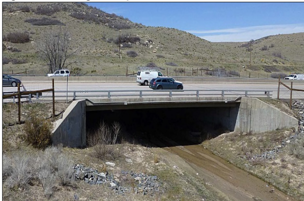
Figure 1. Existing Underpass at MP 191.1
