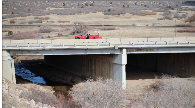
Figure 2. Existing East Plum Creek Bridge at MP 172.2
