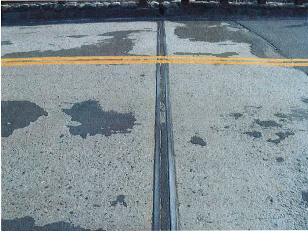
View Showing Joint at East Abutment Filled with Polymer Coating
