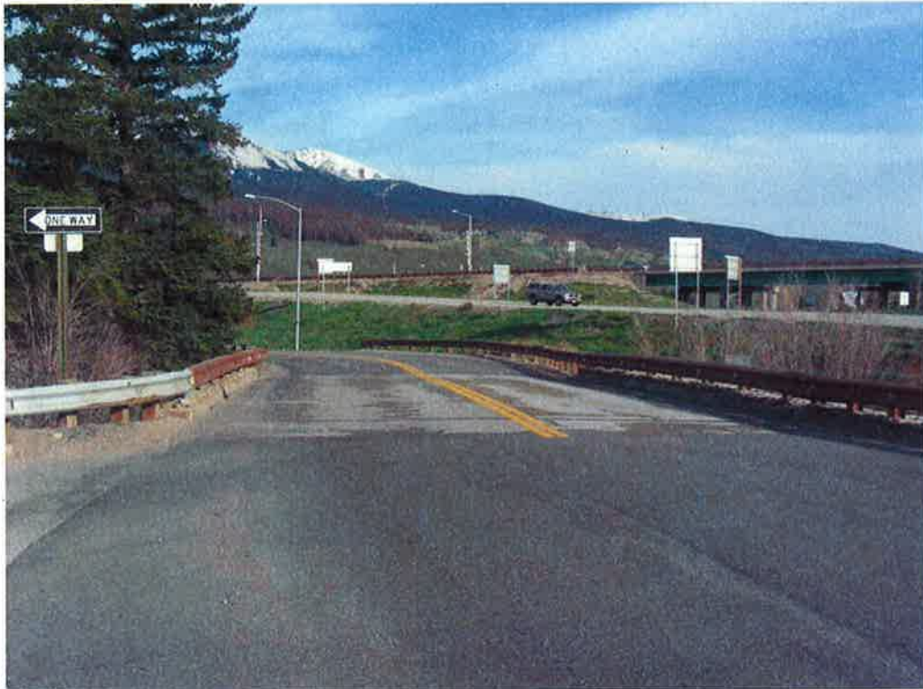
View Down Centerline Bridge Roadway Looking Upstation
