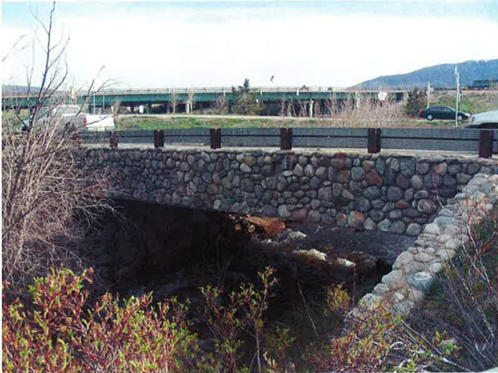
View of Bridge Side Elevation Looking Upstream
