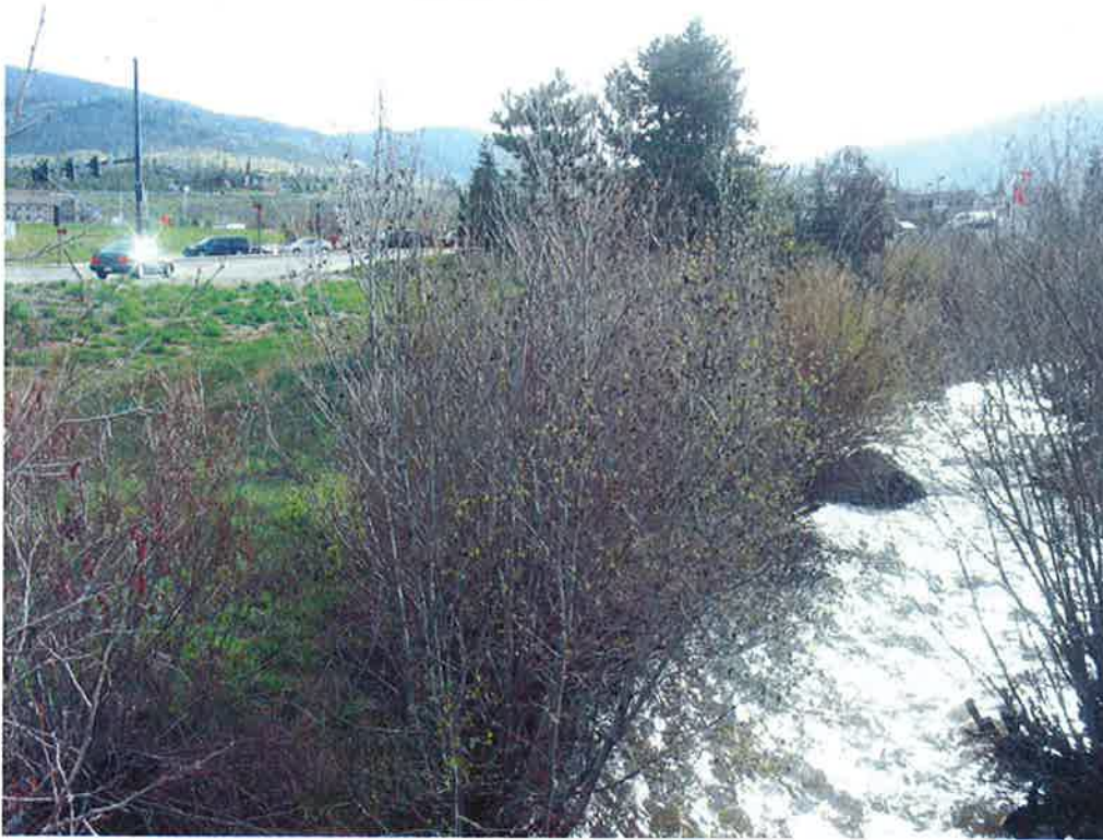
View Looking Upstream, Left Bank
