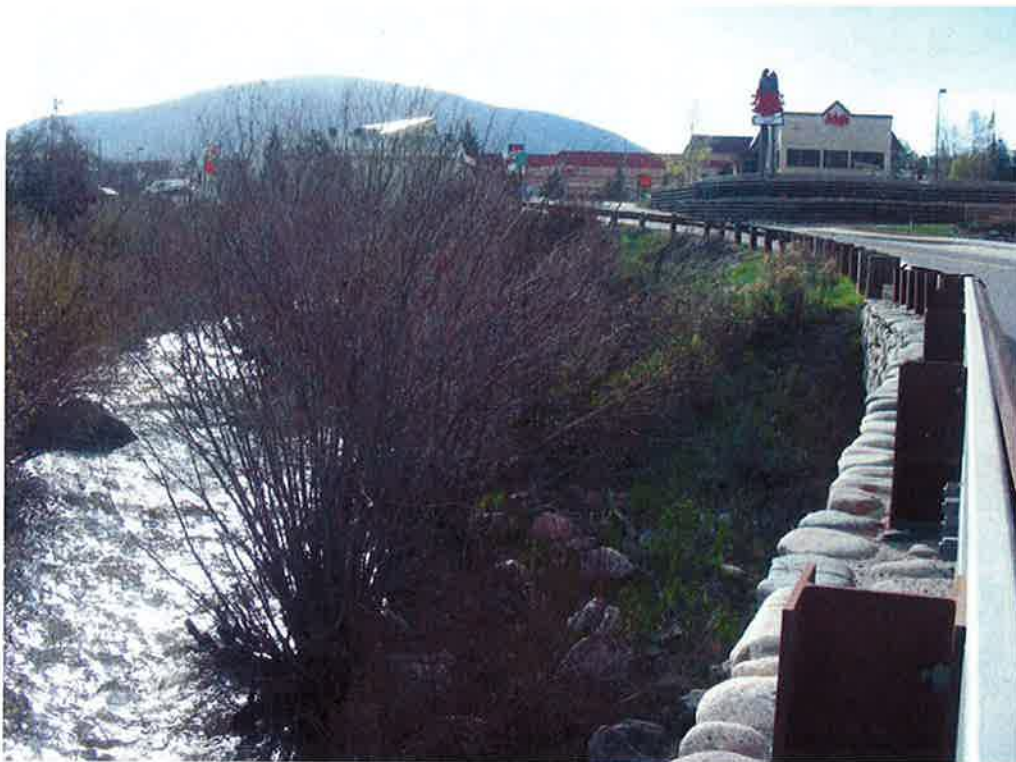
View Looking Upstream, Right Bank
