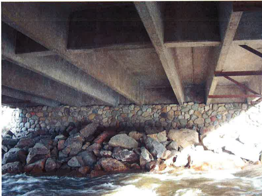
General View of Underside of Bridge Looking Downstation
