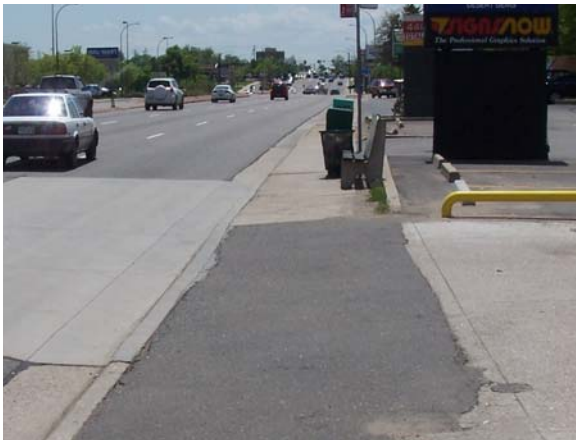
EXHIBIT 1-3: MISSING SIDEWALKS AND OBSTRUCTIONS NEAR 5TH AVENUE
