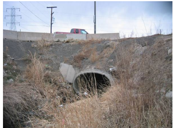
46 EXHIBIT 4-4: DRY GULCH CULVERT
