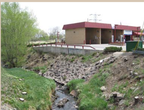
Drainages in the study area have been heavily modified by past development. While the US 6/Wadsworth project would destroy several small wetlands, proposed widening of gulches would improve conditions for new wetlands and natural riparian areas to establish.
