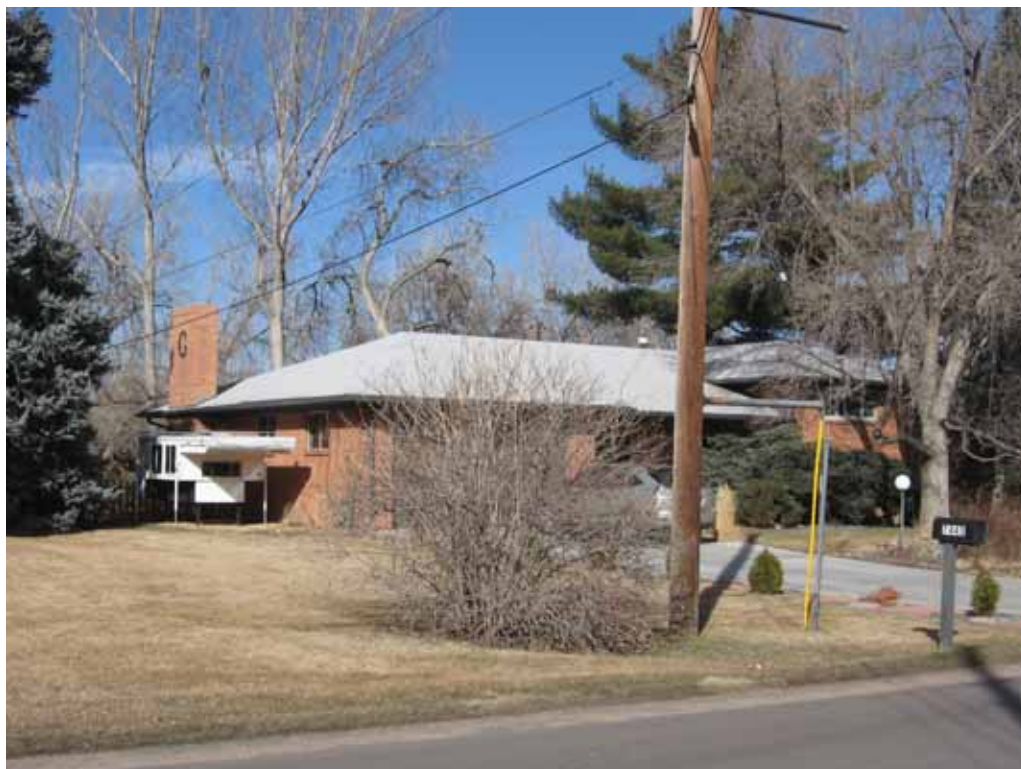
Photograph 2: South and West façades, view to the Northeast
