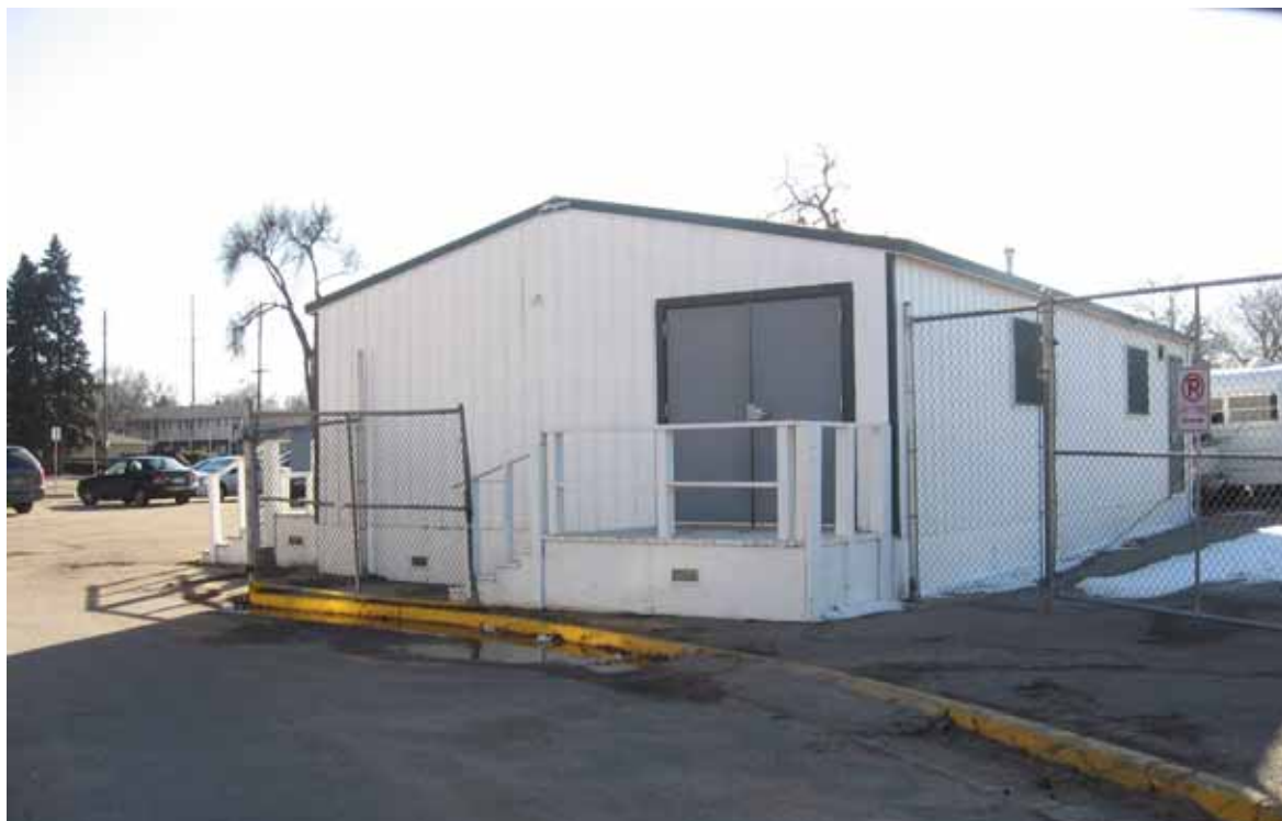
Photograph 40. Structure 15: Storage Outbuilding, east and north facades, view to the Southwest
