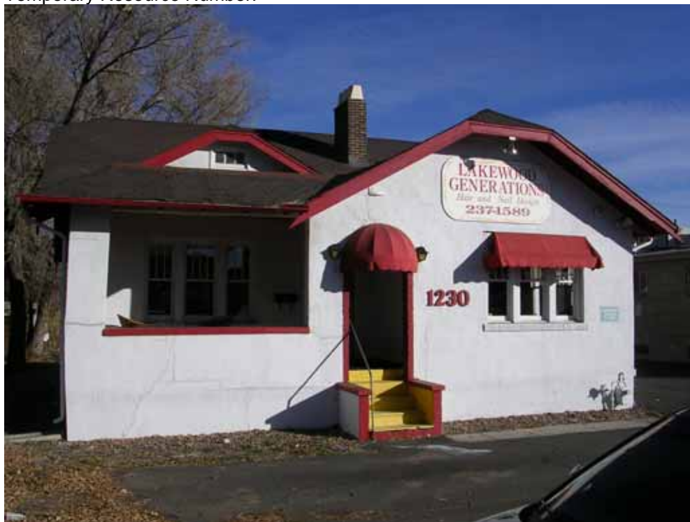
Photograph 1. West façade, view looking East
