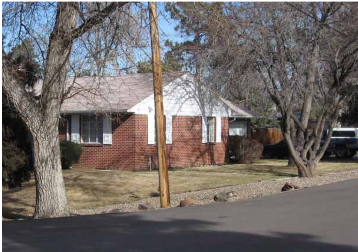
Photograph 3: West and south façades, view to the Northeast
