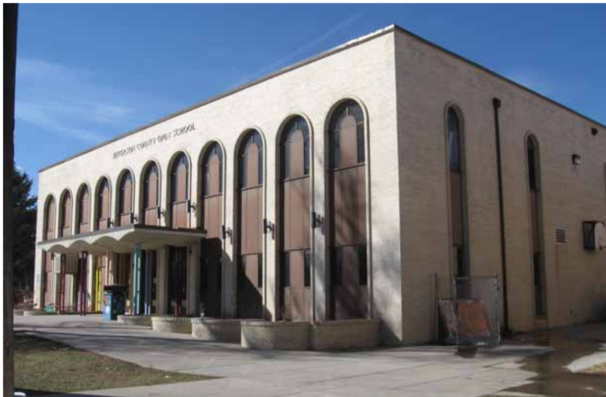
Photograph 17. Building 5: Administration and Arts Building, Jefferson County Open School, south and east façade, view to the Northwest
