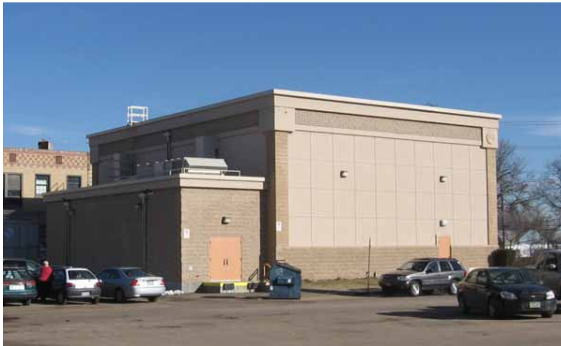
Photograph 27. Building 8: Theater, west and north facades, view to the Southeast
