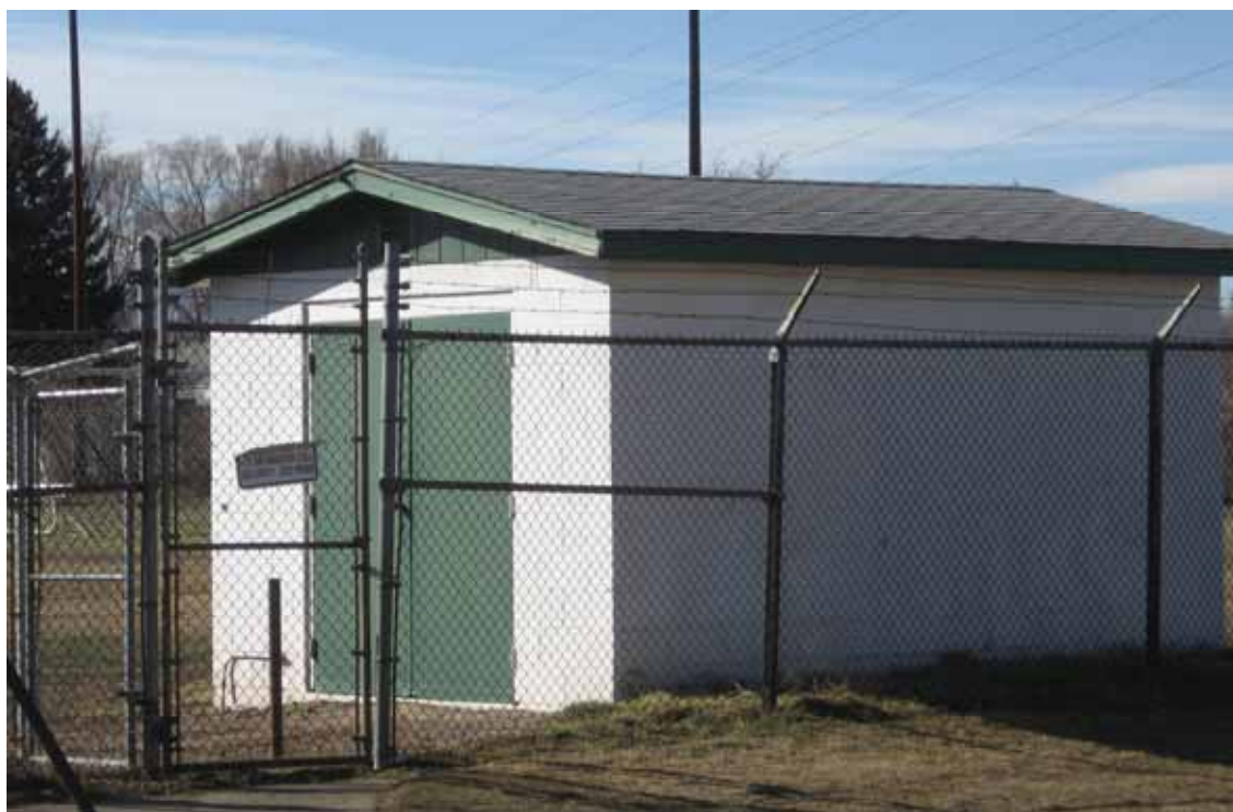
Photograph 34. Structure 12: Storage Outbuilding, Jefferson County Open School, south and east facades, view to the Northwest
