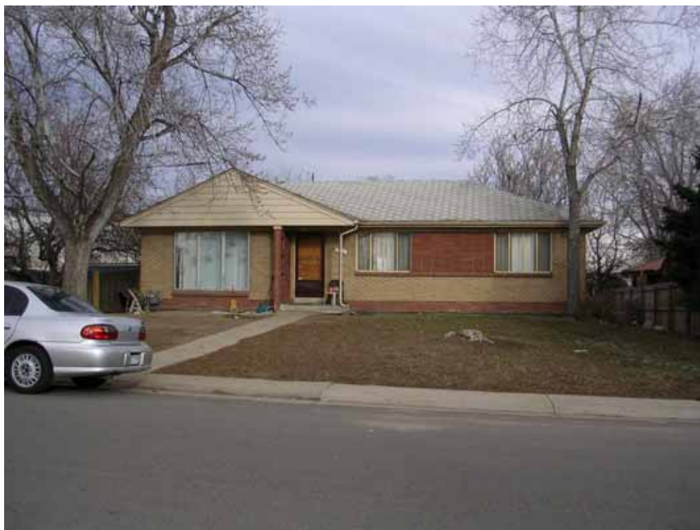
Photograph 2: West façade, view looking East
