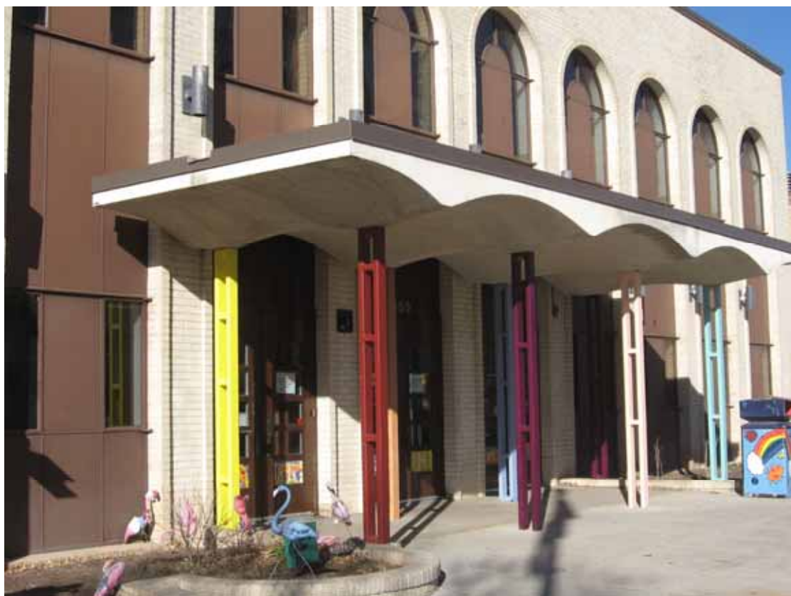
Photograph 20. Administration and Arts Building, entrance canopy
