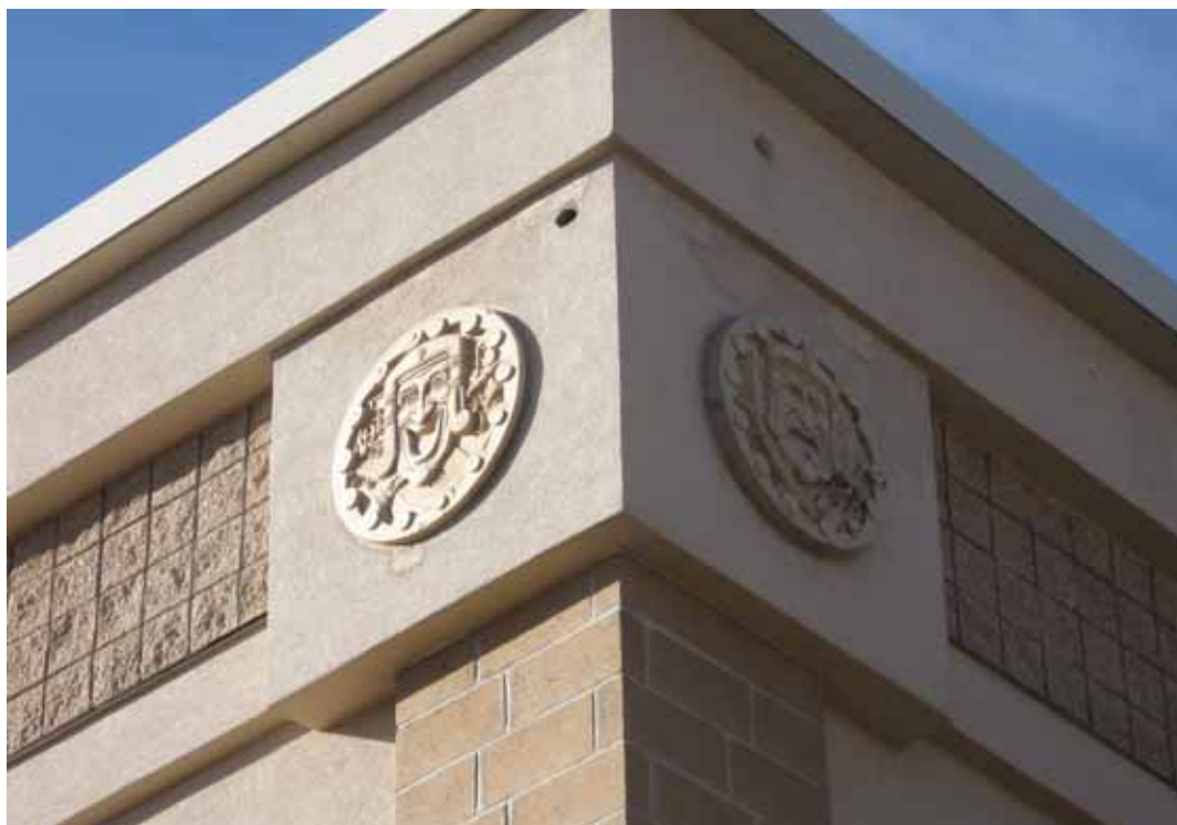
Photograph 28. Building 8: Theater, southeast corner medallions
