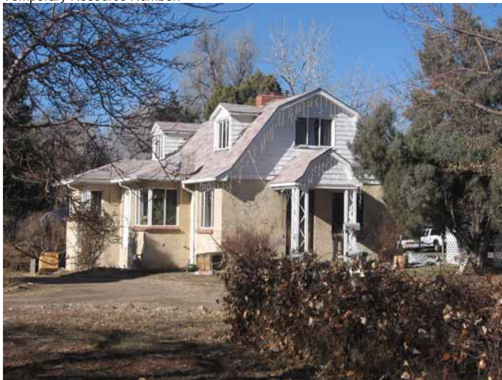
Photograph 1: East and South façades, view looking Northwest
