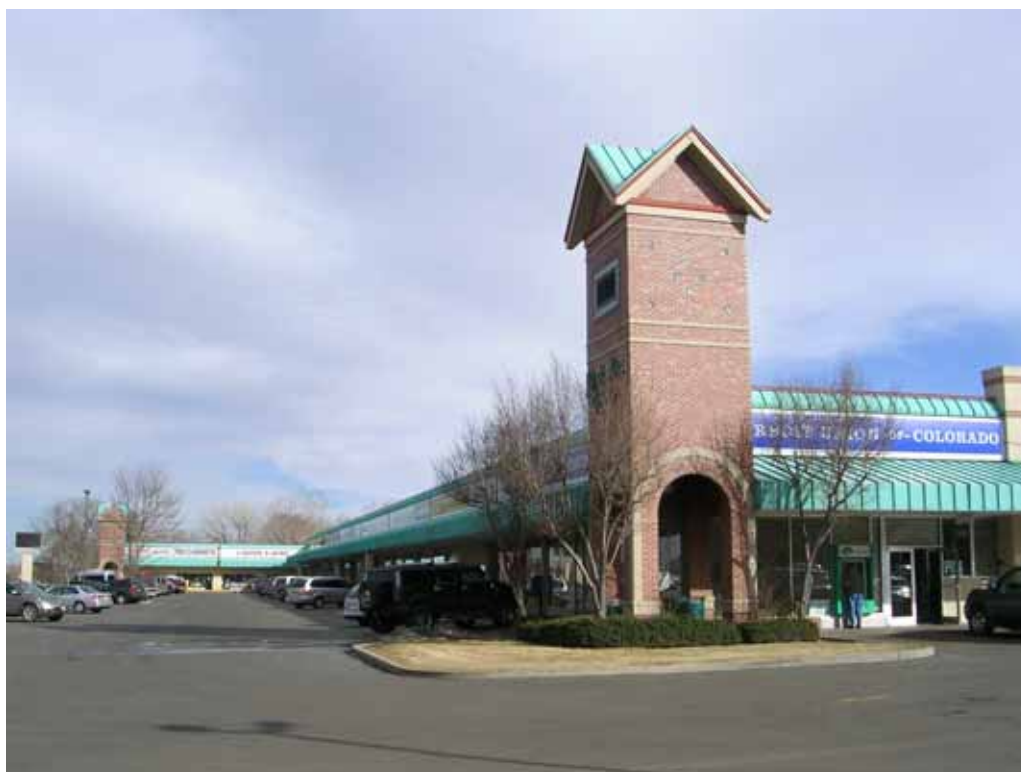
Photograph 2: North and West façades, view looking East
