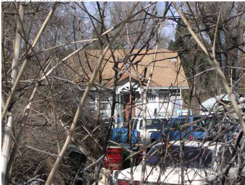
Photograph 1: South façade, view looking North
