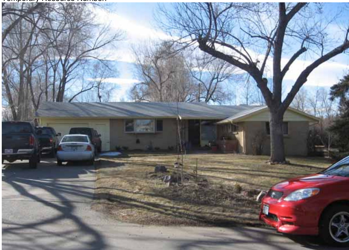
Photograph 1: East façade, view to the West
