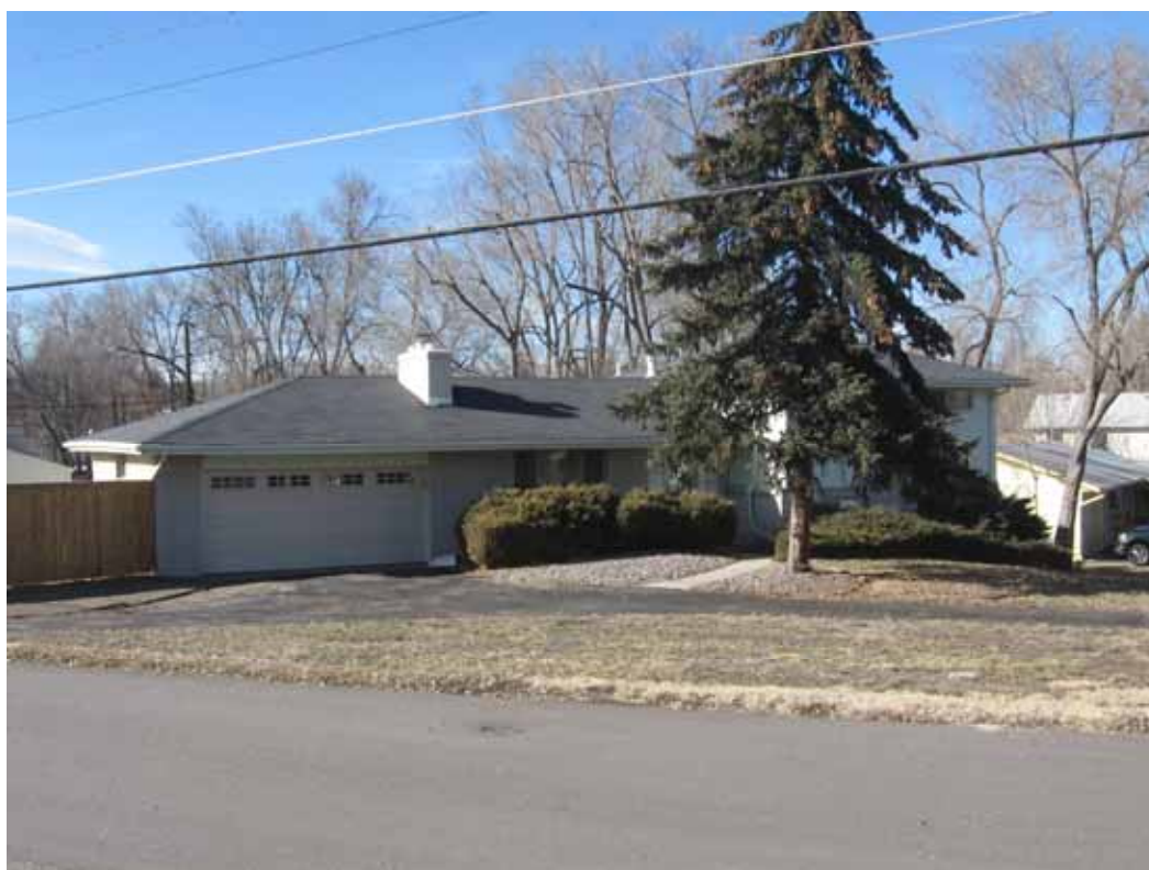
Photograph 2: East façade, view to the Northwest
