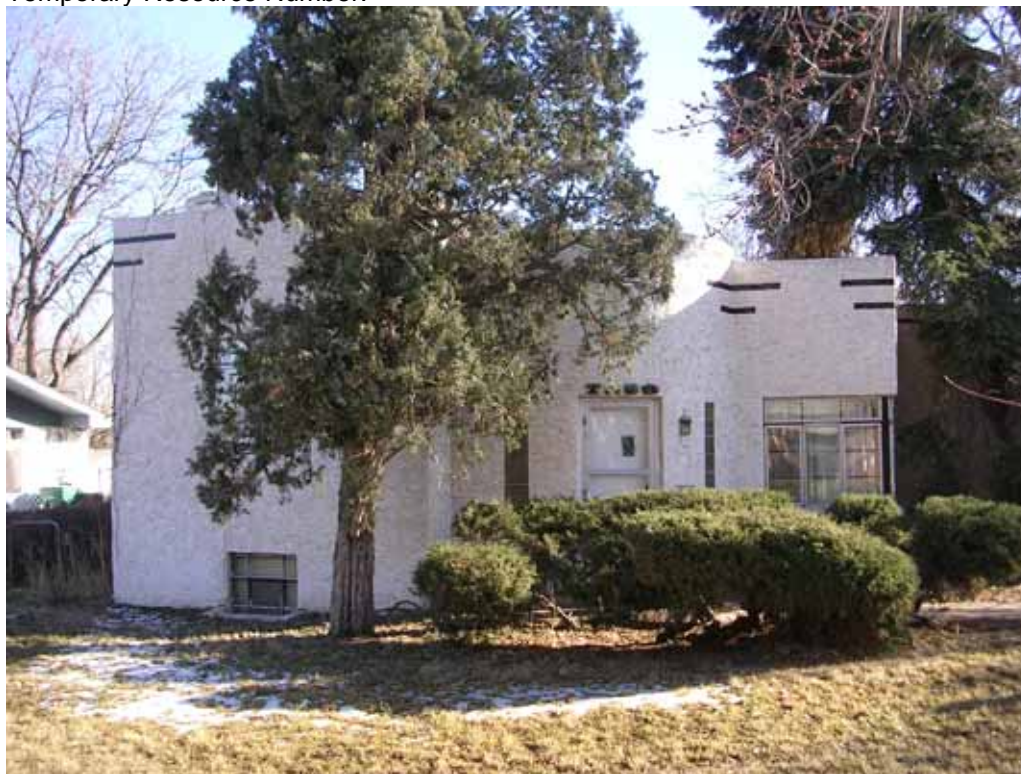
Photograph 1: North façade, view looking Southeast
