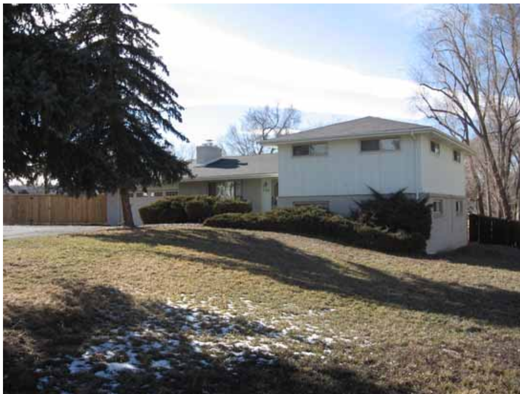
Photograph 1: East and North facades, view to the Southwest
