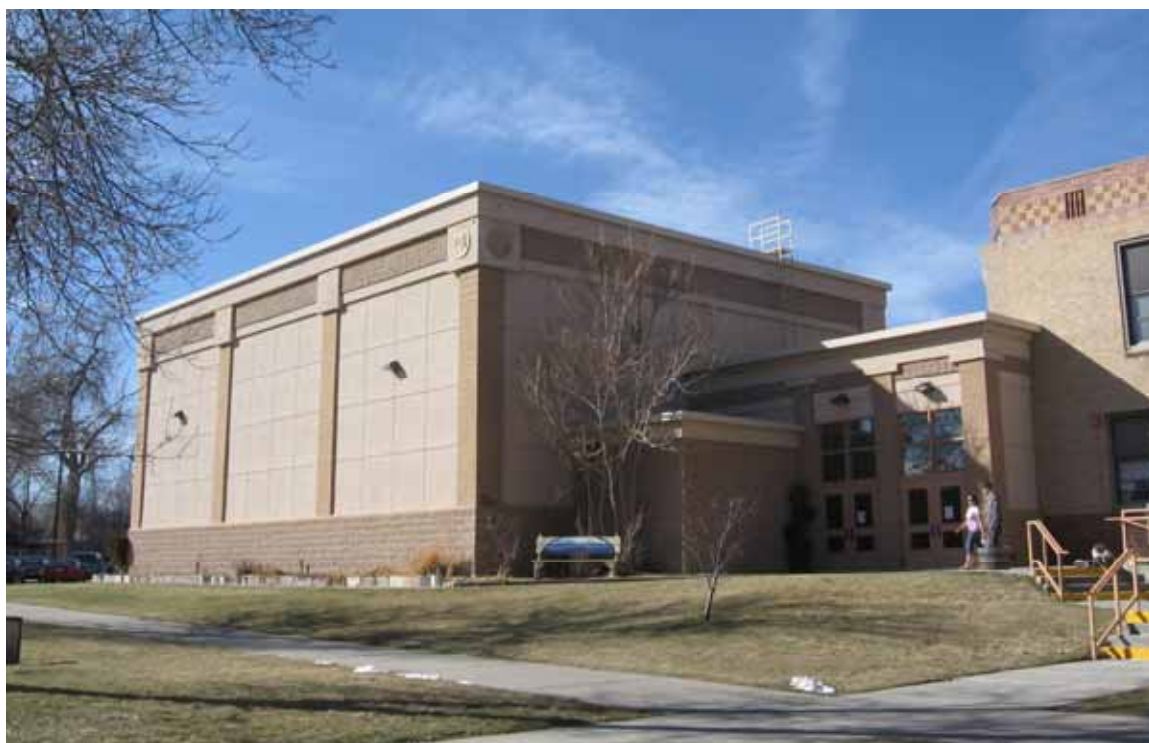
Photograph 26. Building 8: Theater, Jefferson County Open School, south and east facades, view to the Northwest
