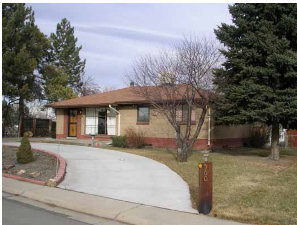
Photograph 2: West and South façades, view looking Northeast
