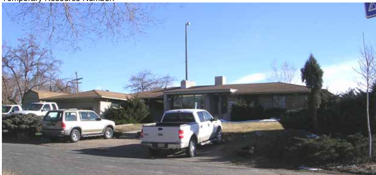
Photograph 1: North façade, view to the Southeast
