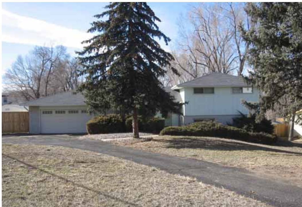
Photograph 3: East façade, view to the West
