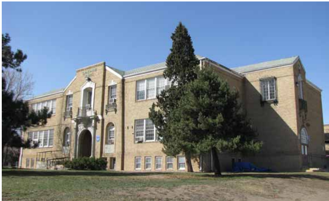
Photograph 1. New America School (Building 1), view to the Southwest
