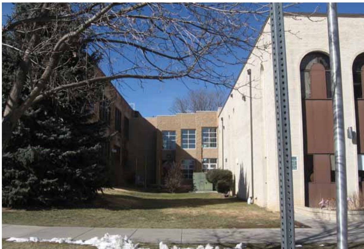
Photograph 22. Connecting Building, west end, south façade, view to the North
