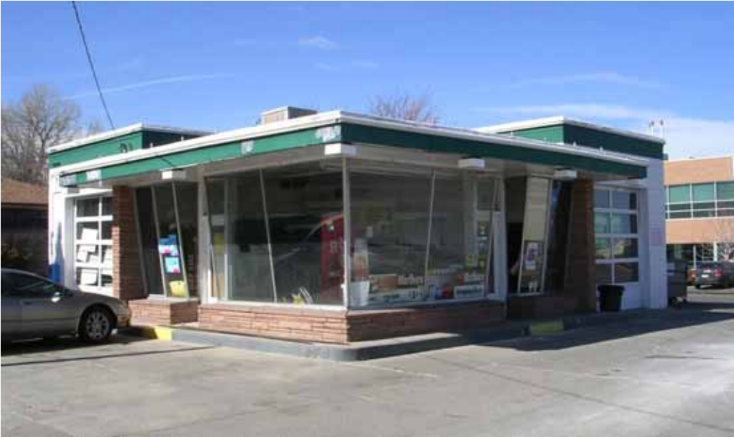
Photograph 1: East and South façades, view looking Northwest
