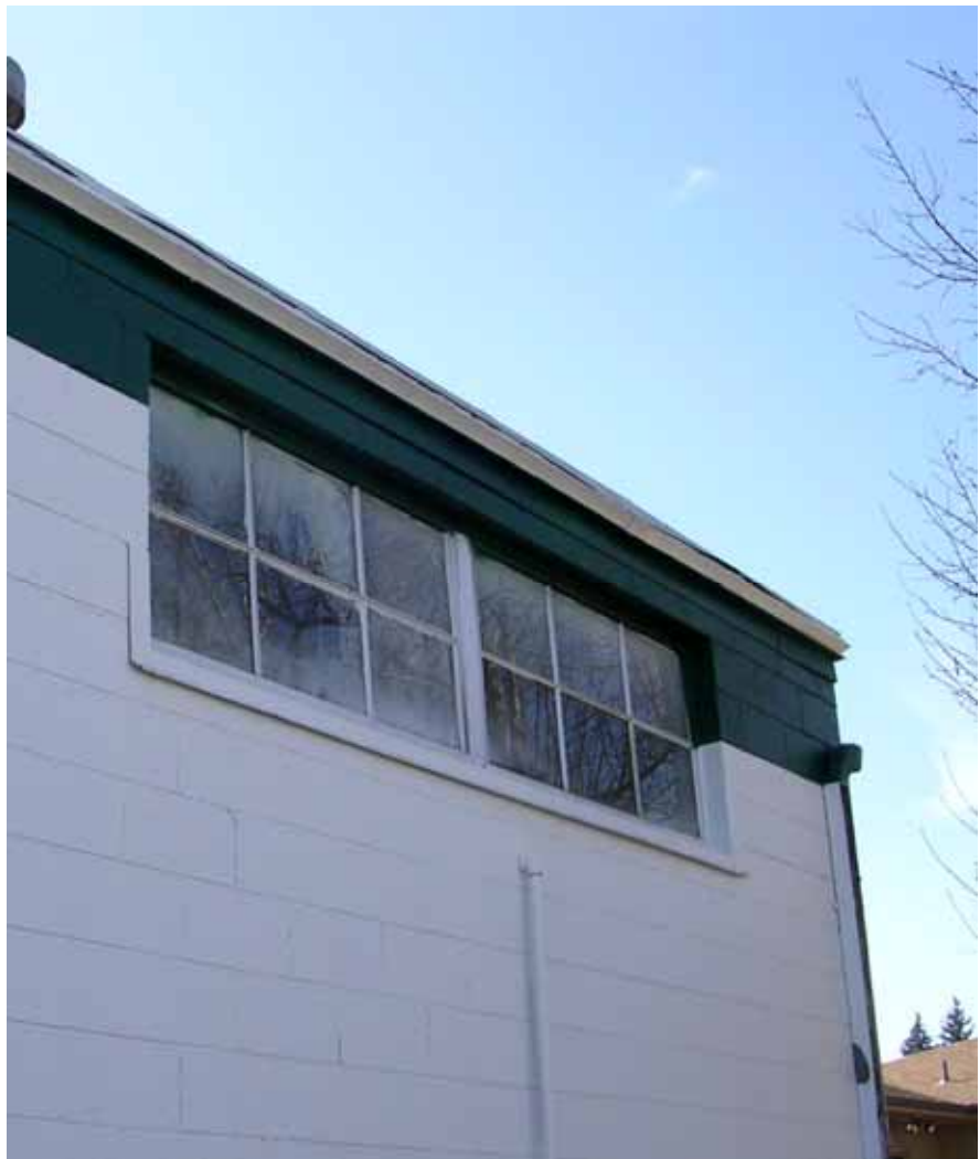
Photograph 5: North façade, awning window detail, view to the Southwest
