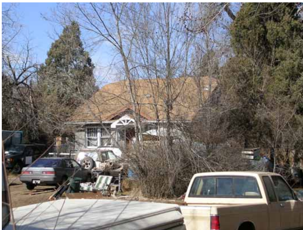
Photograph 2: South façade, view looking Northwest
