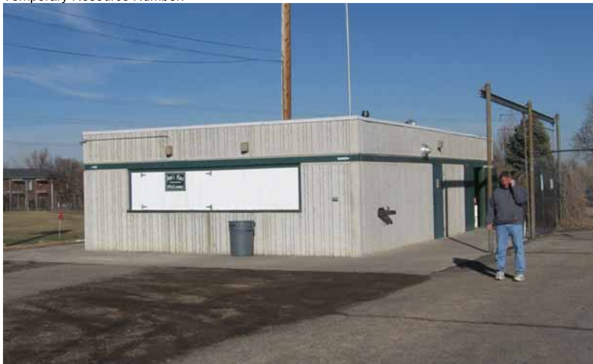
Photograph 37. Structure 14: Concessions Building, Jefferson County Open School, south and east facades, view to the North, Northwest
