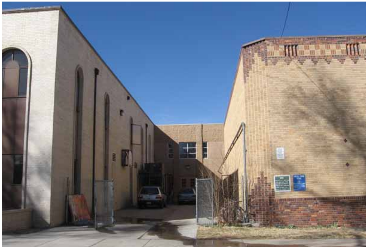
Photograph 21. Building 6: Connecting Building, Jefferson County Open School, east end, south façade, view to the North
