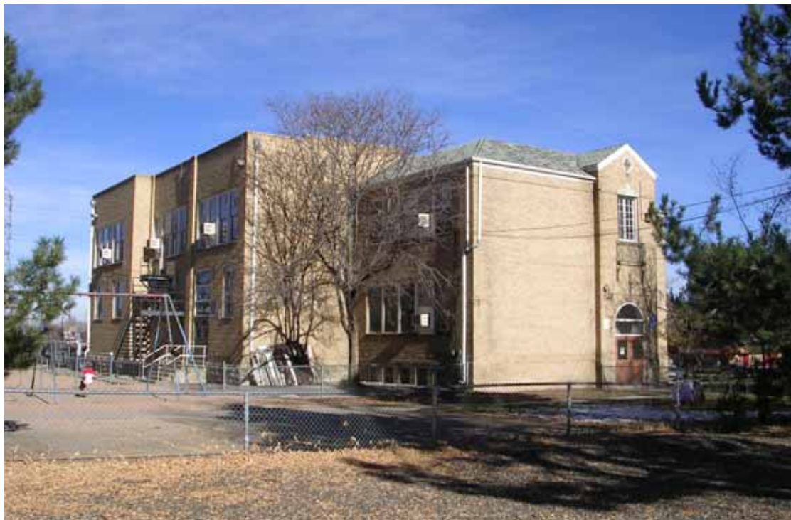
Photograph 5. New America School, west and south façade, view to the Northeast
