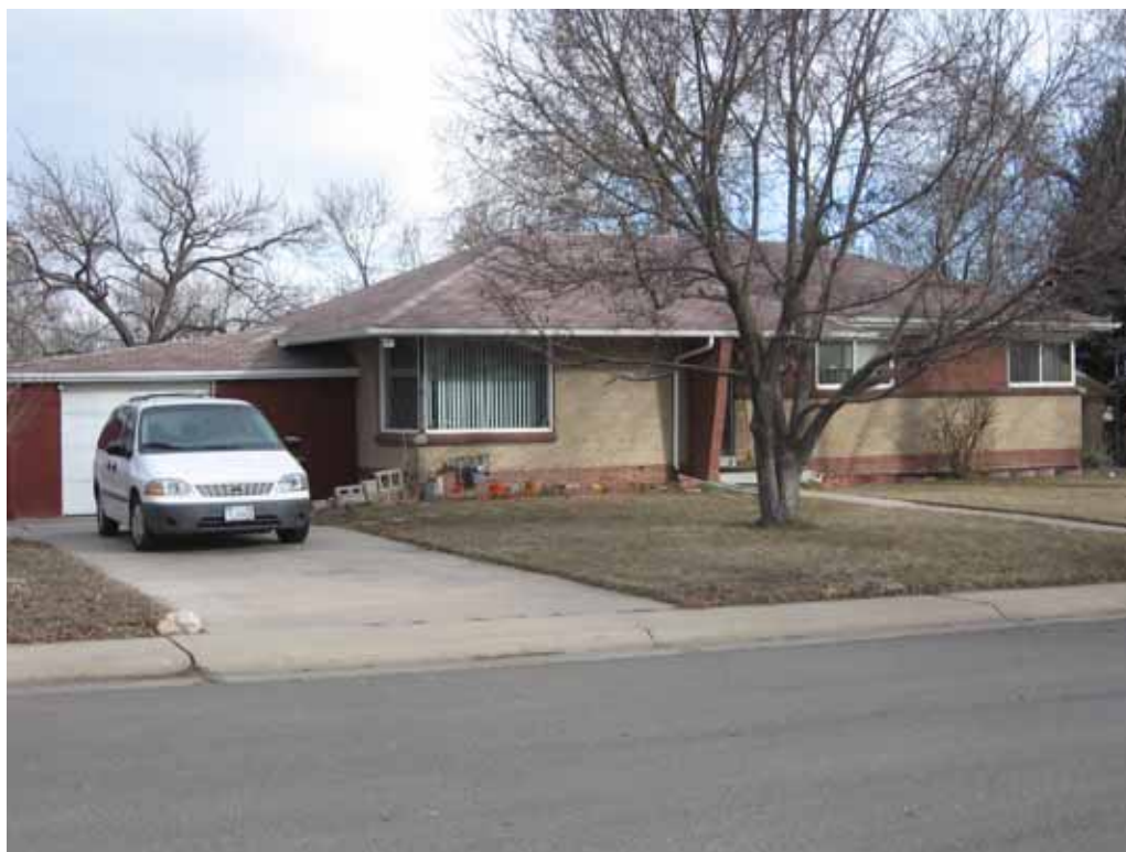
Photograph 2: West façade, view to the Southeast
