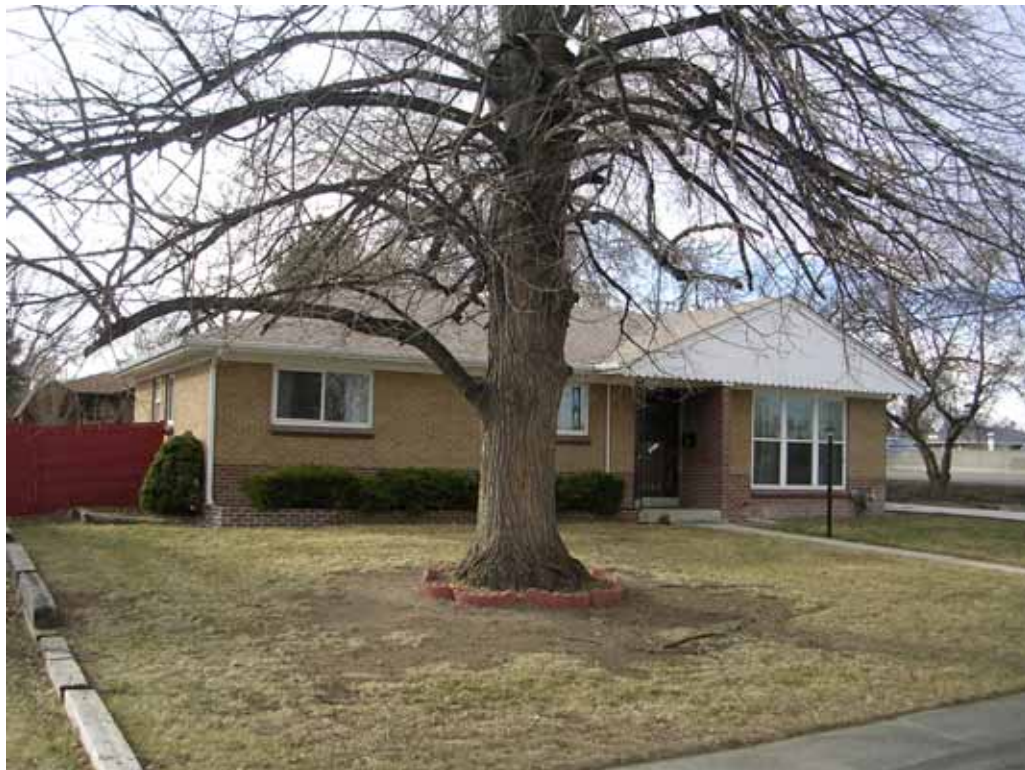
Photograph 1: East and South façades, view looking Northwest
