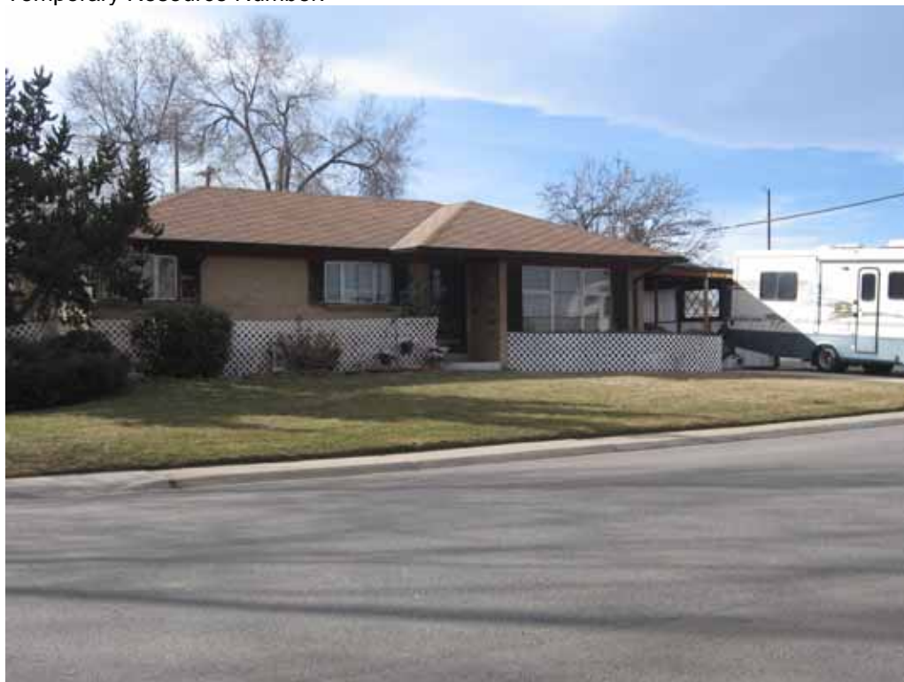
Photograph 1: East façade, view to the Northwest
