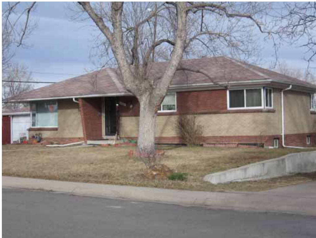
Photograph 1: West façade, view to the Northeast
