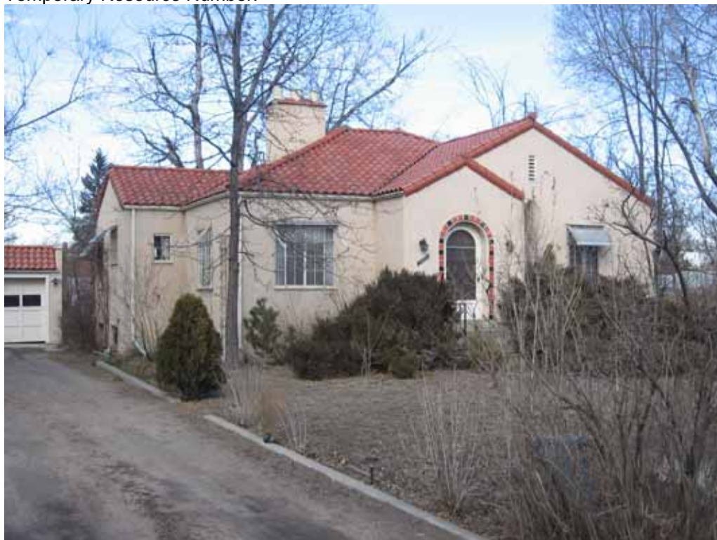
Photograph 1: South and West façades, view to the Northeast
