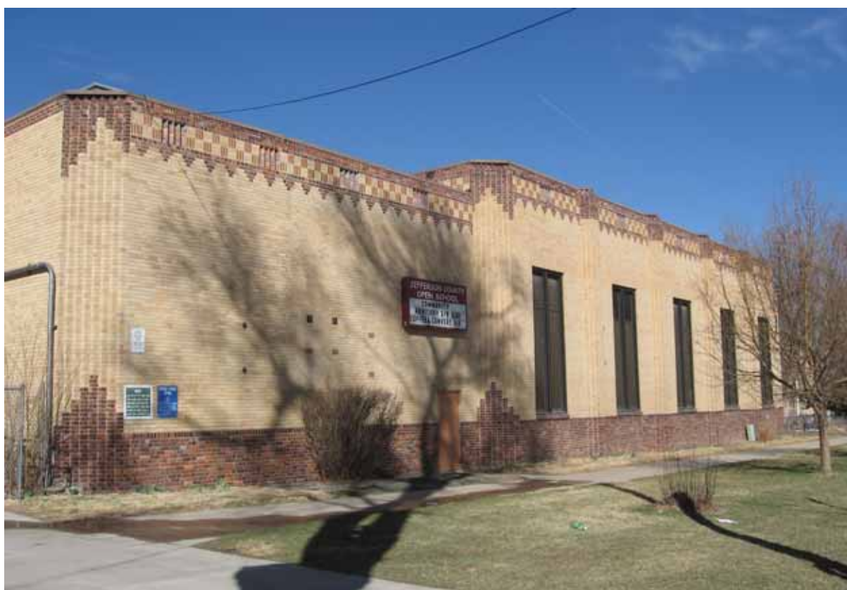
Photograph 14. Building 3: Gymnasium, south façade, view to the Northeast
