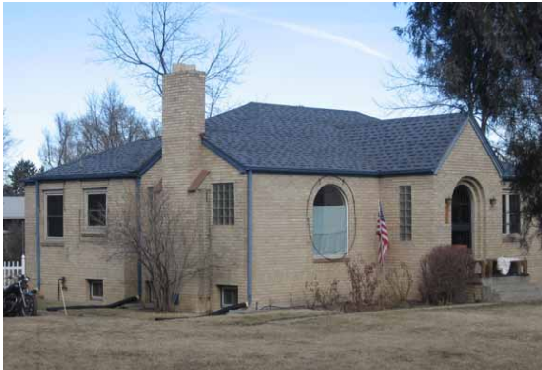
Photograph 1: West and South façades, view to the Northeast
