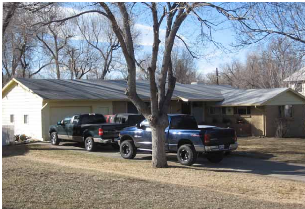
Photograph 2: East and South facades, view to the Northwest
