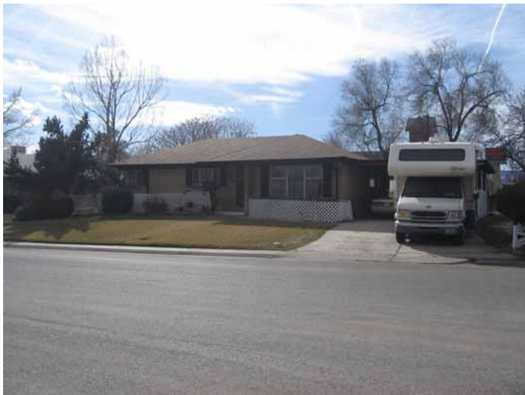
Photograph 2: East façade, view to the Southwest
