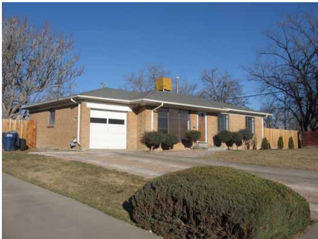
Photograph 1: East and South façades, view to the Northwest
