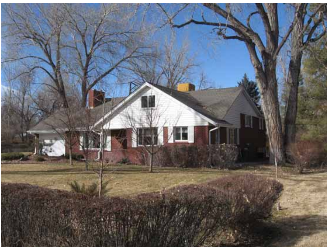
Photograph 2: South and East façades, view to the Northwest
