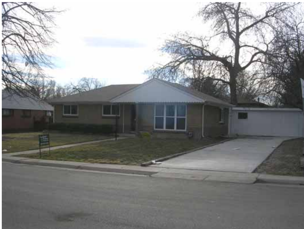
Photograph 2: East and North façades, view looking Southwest
