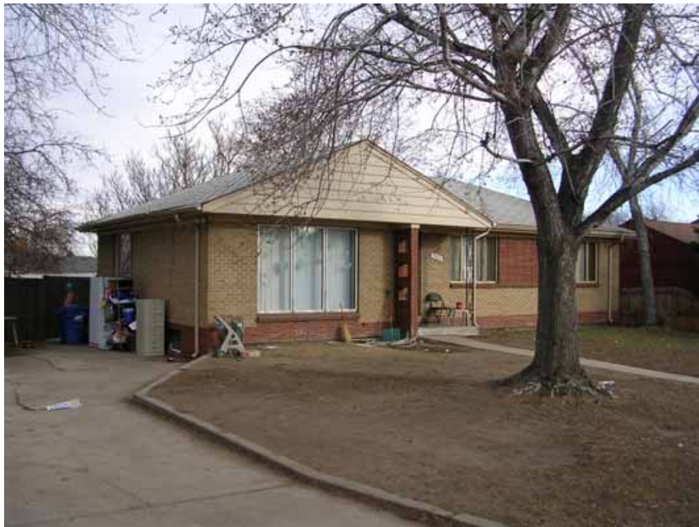
Photograph 1: West and North façades, view looking Southeast
