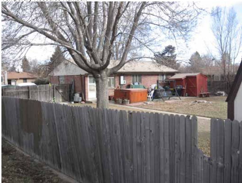
Photograph 3: West façade, view to the Southeast
