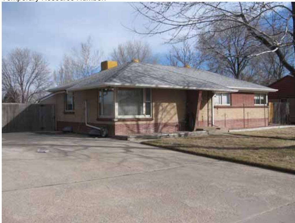
Photograph 1: West Façade, view to the SE
