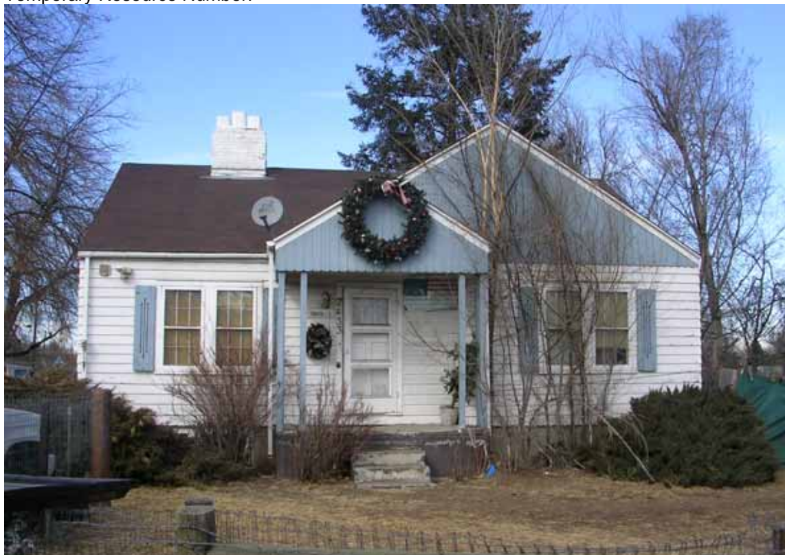
Photograph 1. South façade, view looking North
