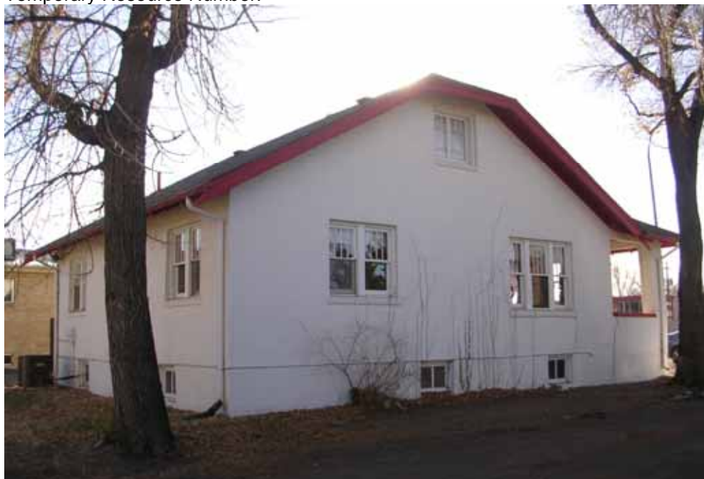
Photograph 3. East and North façades, view looking Southwest
