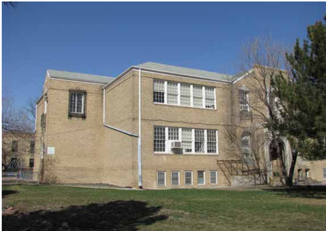
Photograph 3: New America School East façade, view to the Northwest
