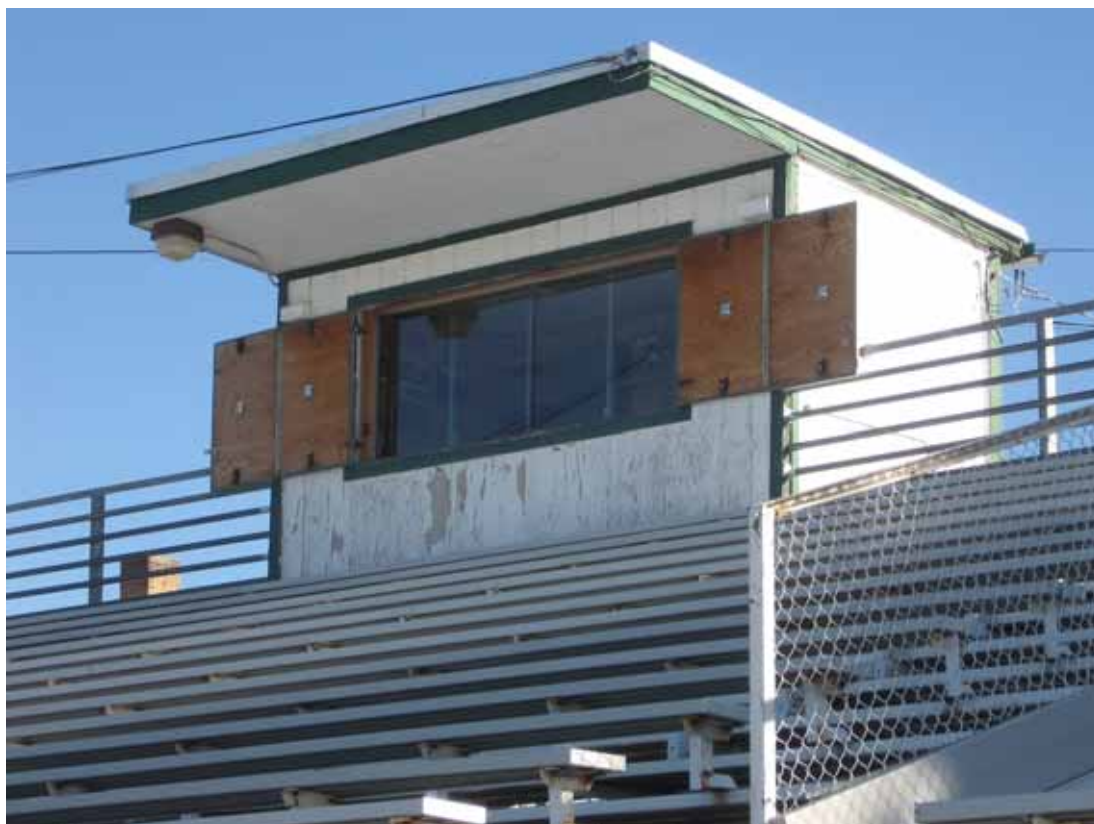
Photograph 42. Structure 16: Bleachers, Announcer's Box, view to the South, Southeast
