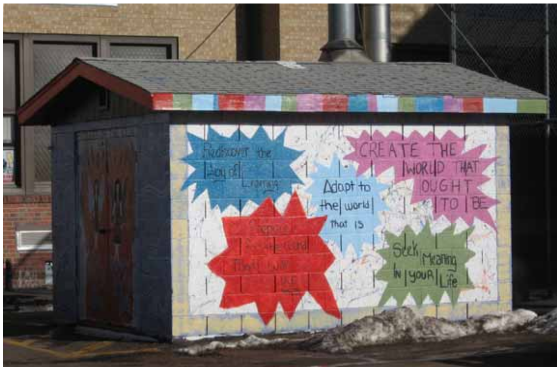
Photograph 29. Structure 9: Outbuilding, Jefferson County Open School, north and west facades, view to the Southeast
