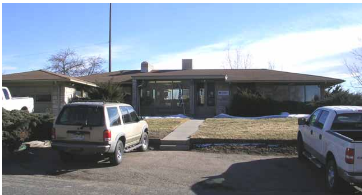
Photograph 2: North façade, view to the South
