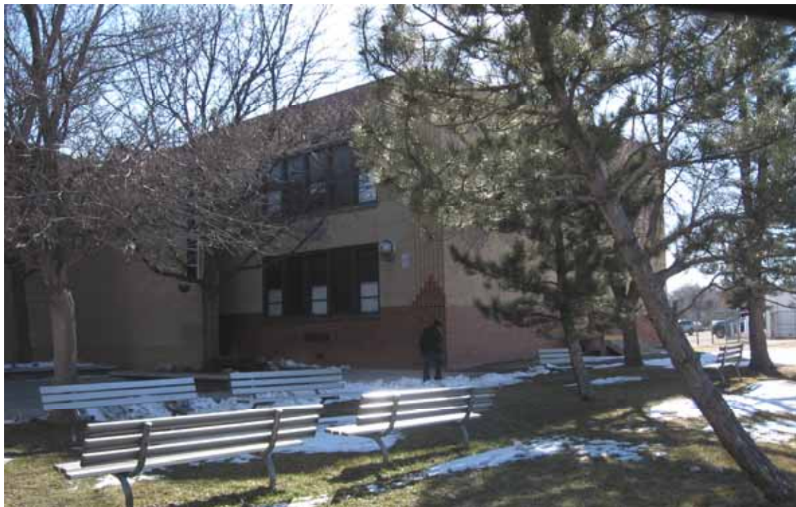
Photograph 25. Building 7: Junior High School, east and north facades, view to the southwest
