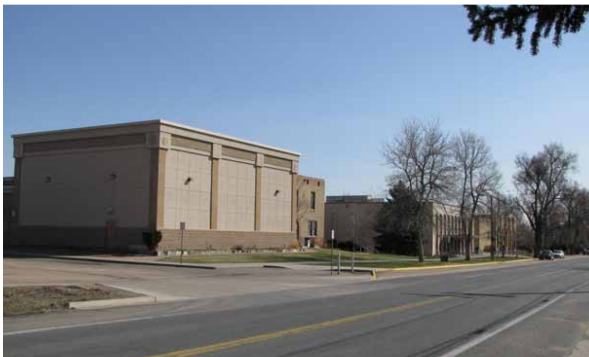
Photograph 56. View of the Jefferson County Open School along W. 10 th Avenue, view to the Northeast
