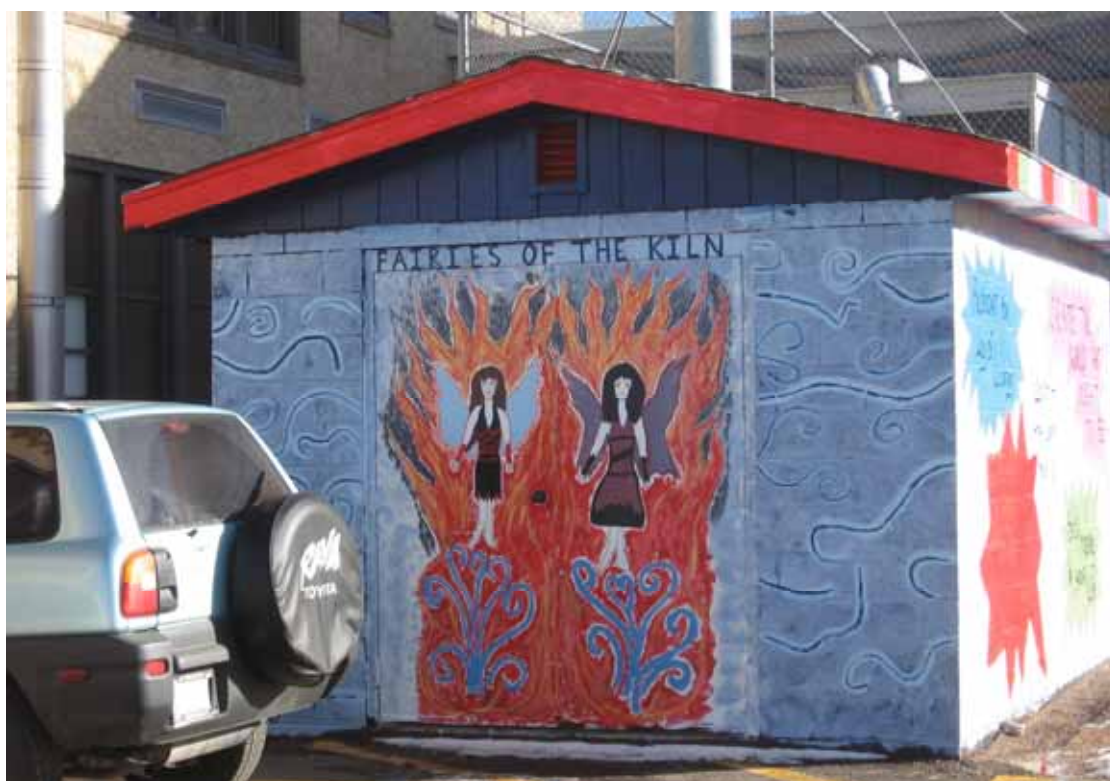
Photograph 30. Structure 9, north façade, view to the South, Southeast
