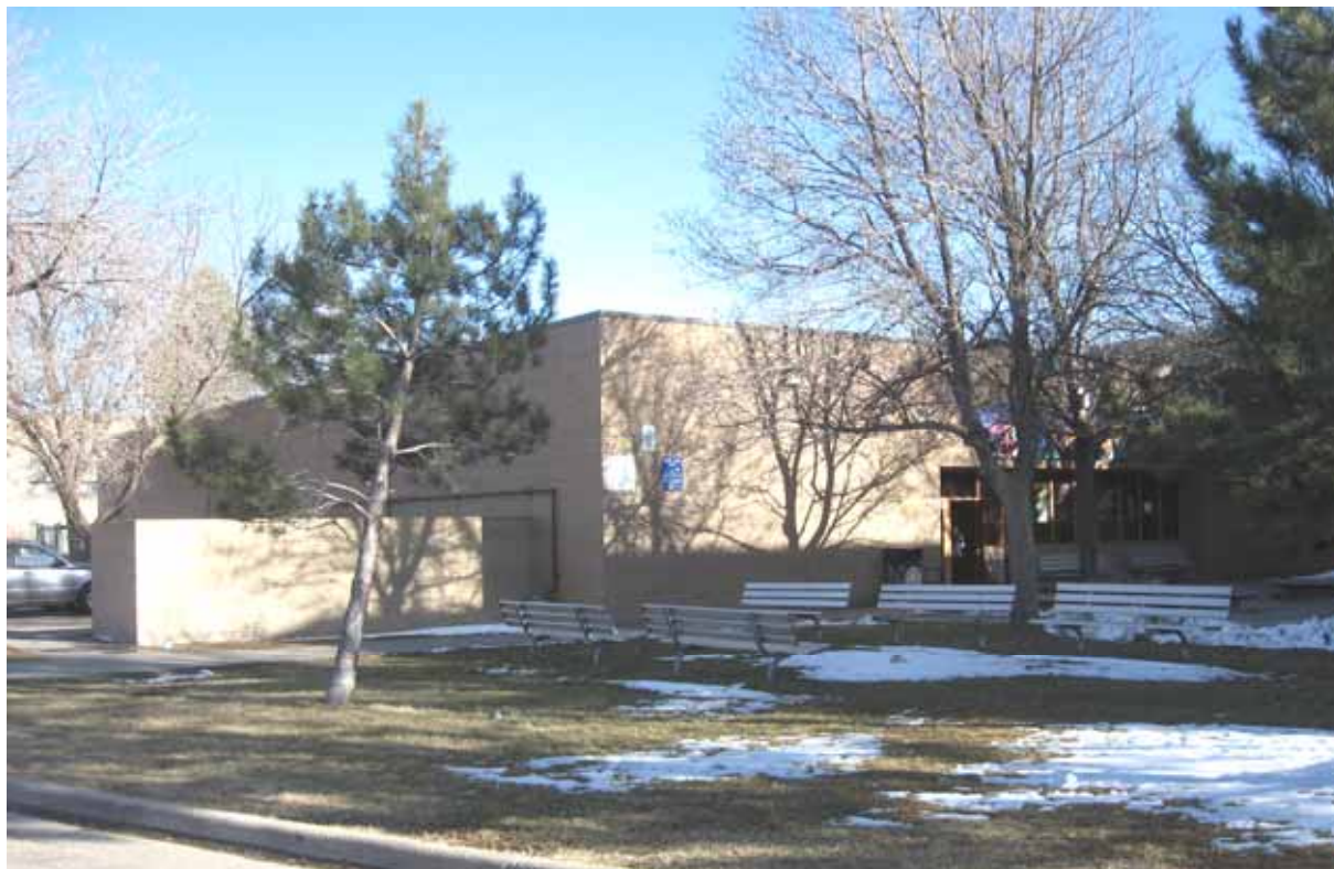
Photograph 15. Building 4: Cafeteria and Library, Jefferson County Open School, north and west facades, view to the Southeast
