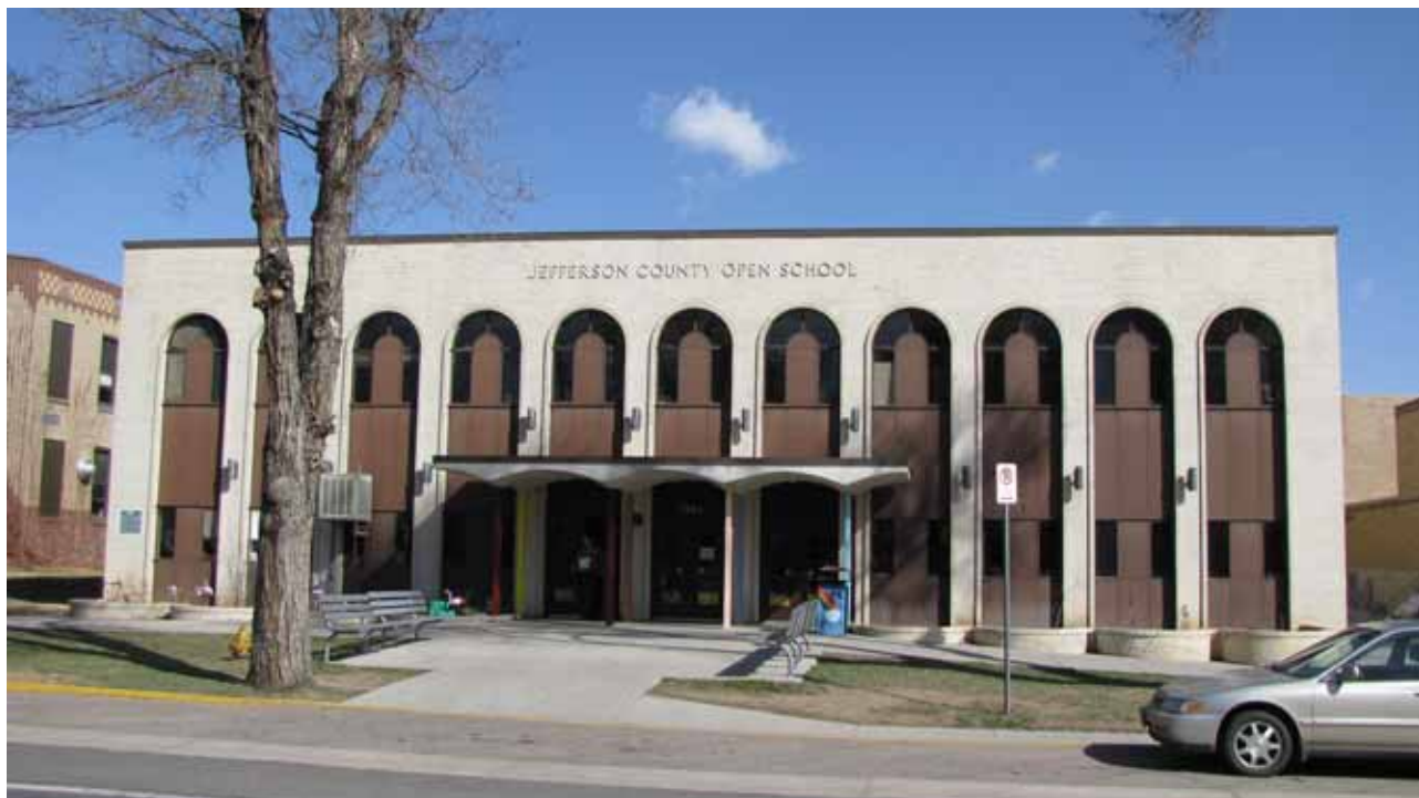
Photograph 19. Administration and Arts Building, south façade, view looking North
