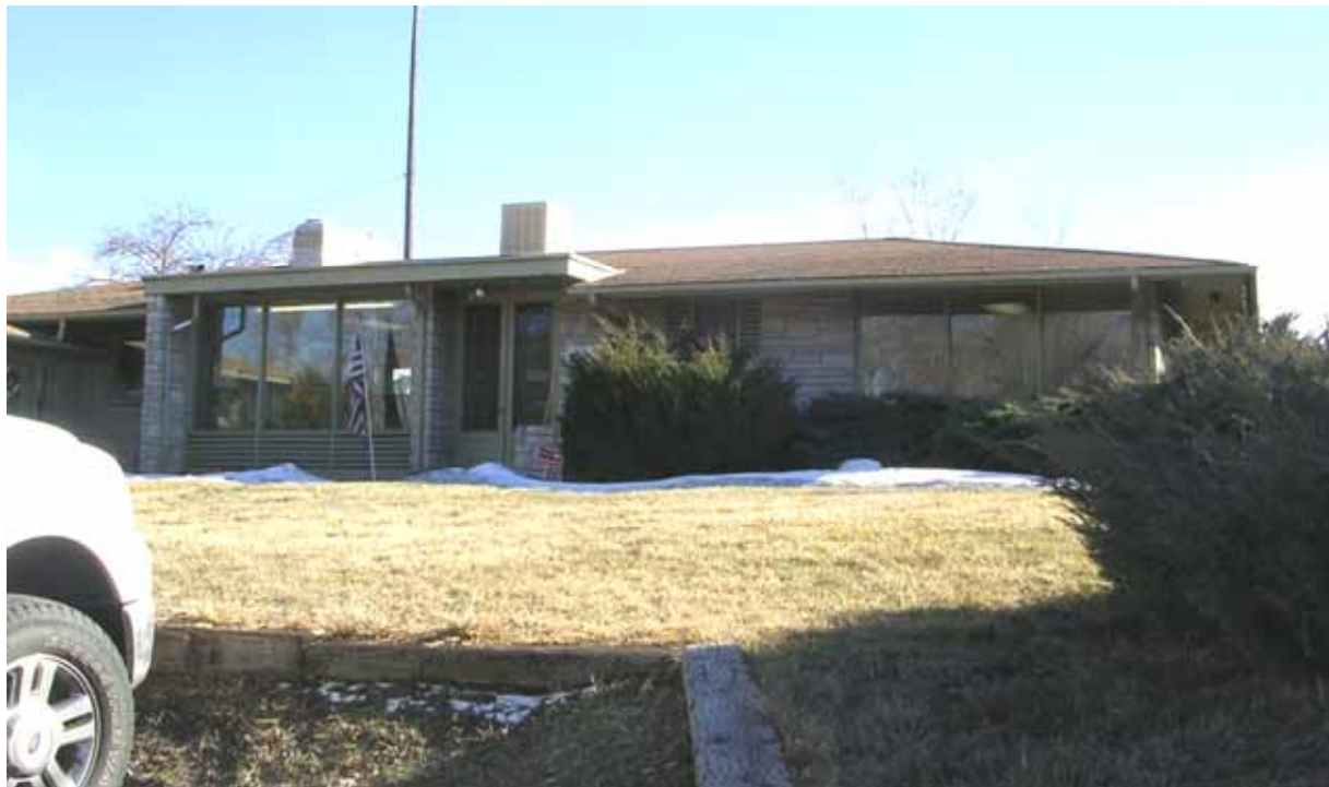
Photograph 3: North façade, view to the South-Southeast
