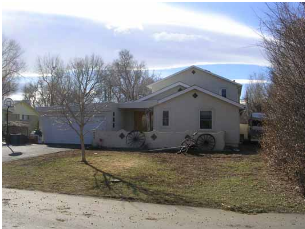
Photograph 2: East façade, view looking Southwest
