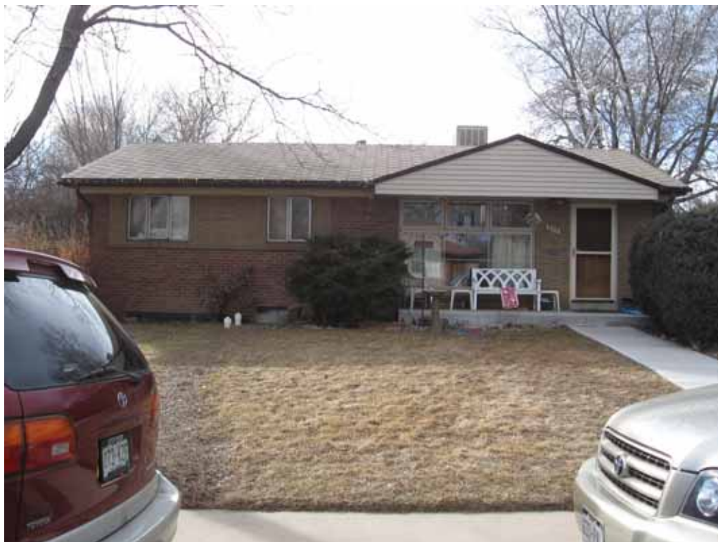
Photograph 2: East façade, view to the West
