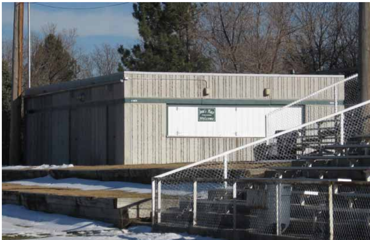
Photograph 38. Structure 14: Concessions Building, north and west facades, view to the Southeast
