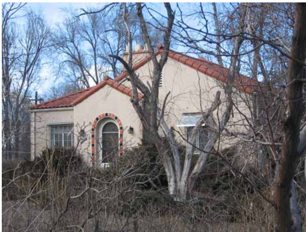
Photograph 2: South façade, view to the Northwest
