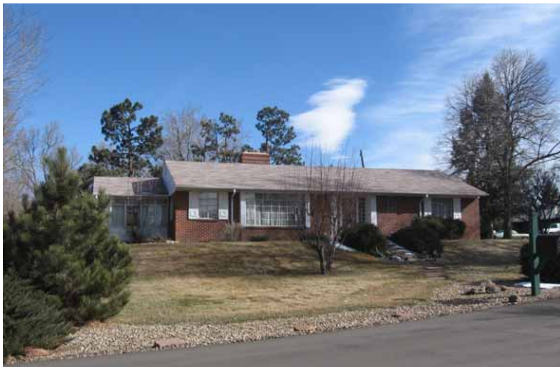
Photograph 1: West façade, view to the East, Southeast
