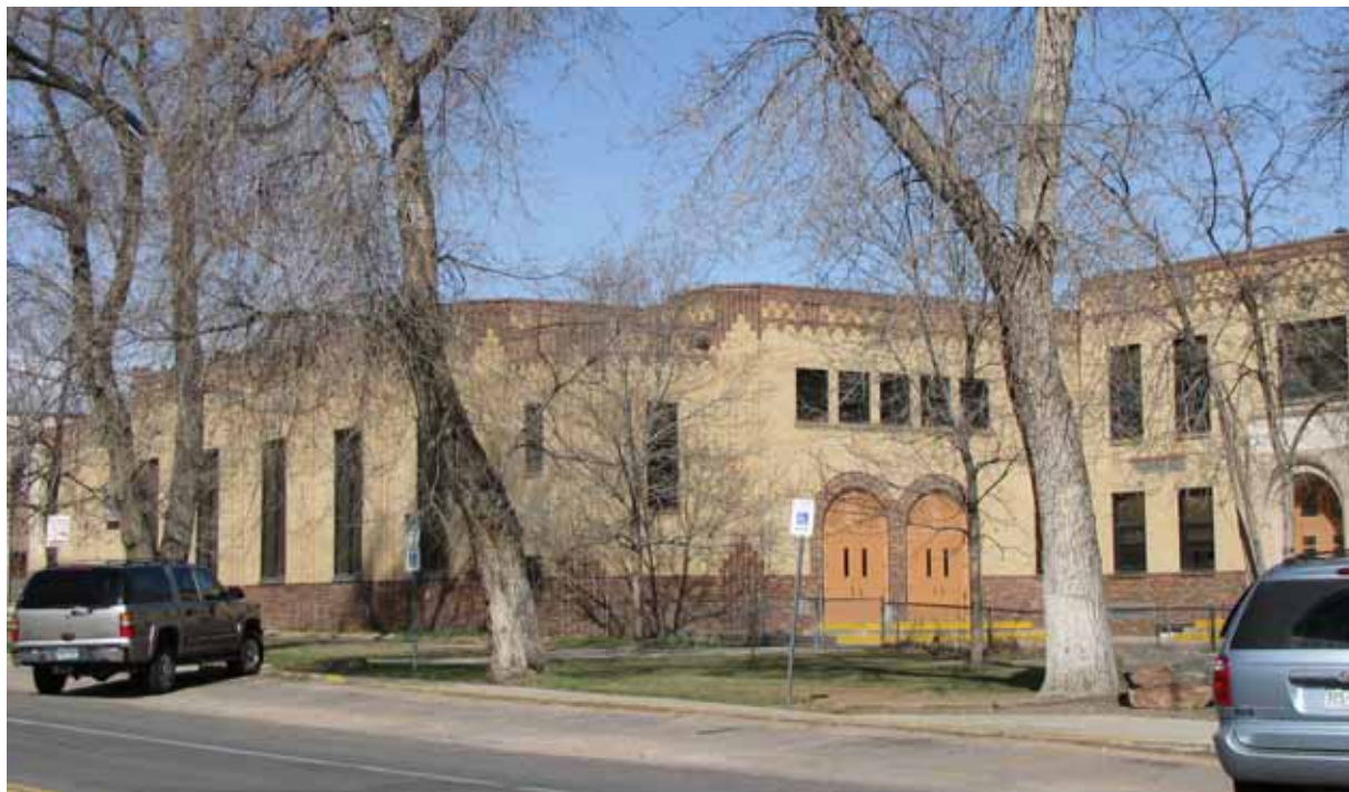
Photograph 13. Building 3: Gymnasium, south and east façade, view to the Northwest
