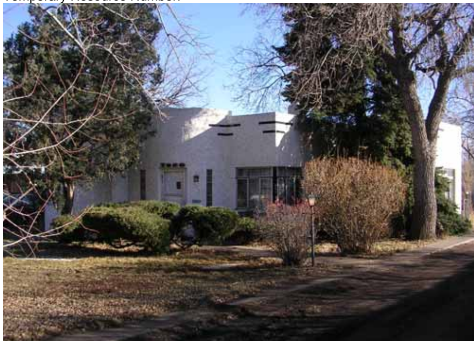
Photograph 3: North and West façades, view looking Southeast
