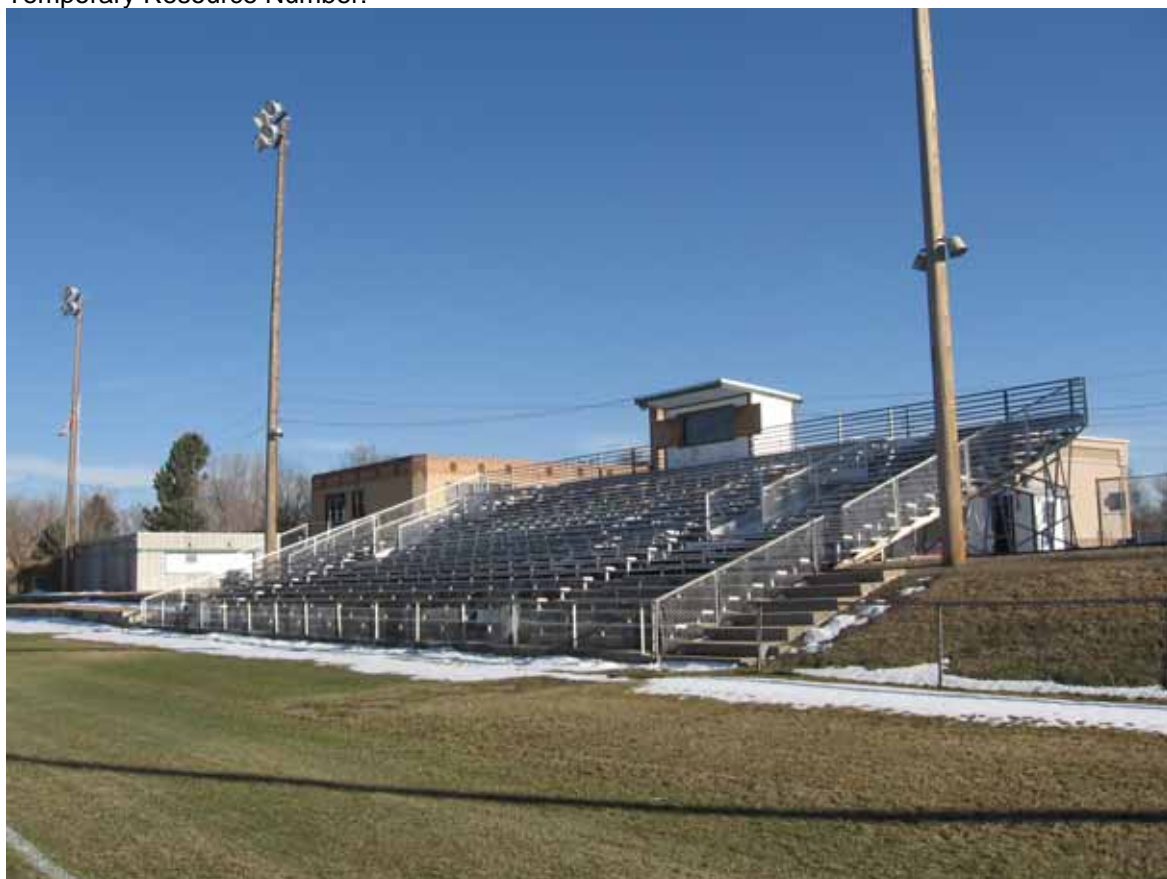
Photograph 41. Structure 16: Bleachers, Jefferson County Open School, view to the Southeast
