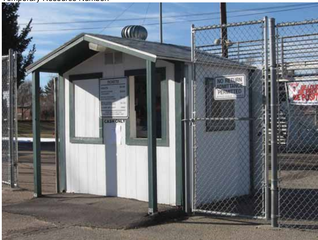
Photograph 45. Structure 17: Ticket Booth, south and east facades, view to the Northwest
