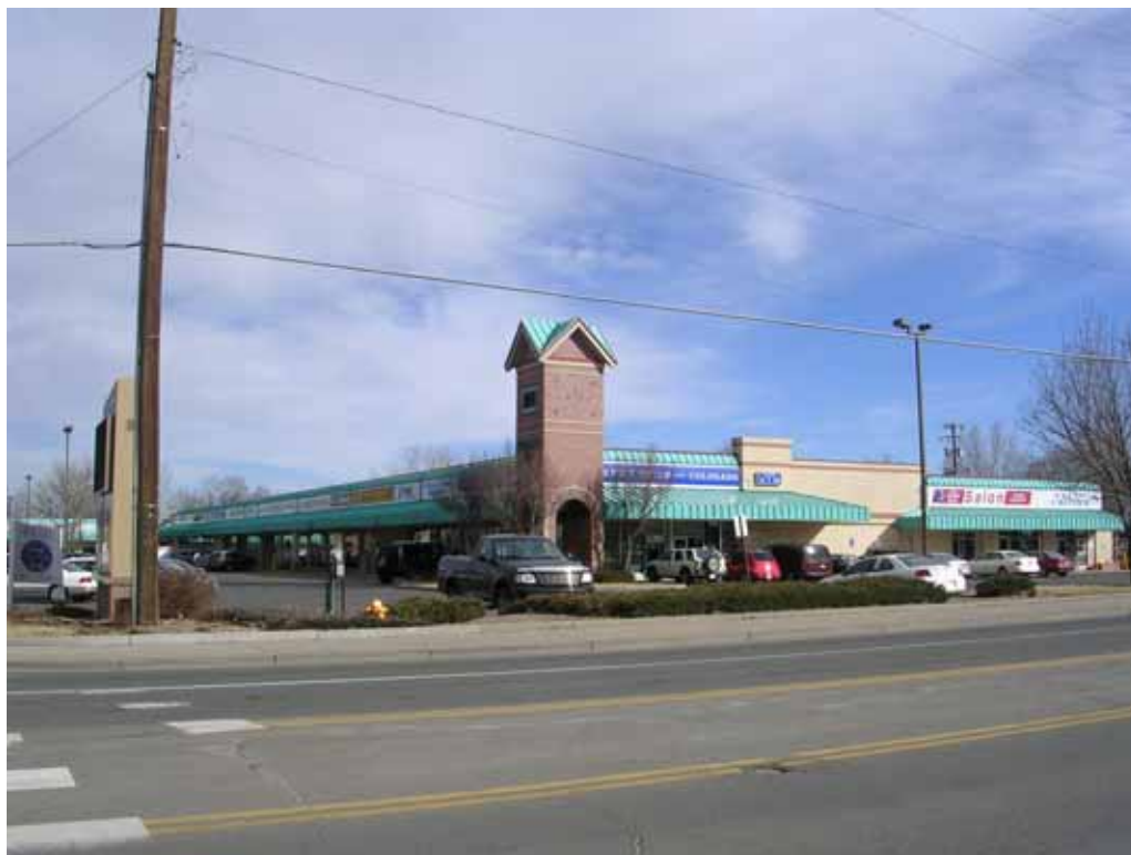
Photograph 1: North and West façades, view looking Southeast
