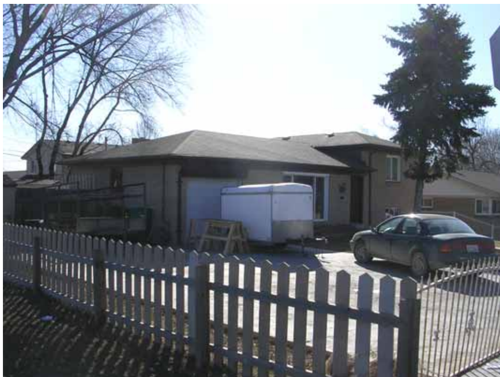
Photograph 2: West and North façades, view looking Southeast
