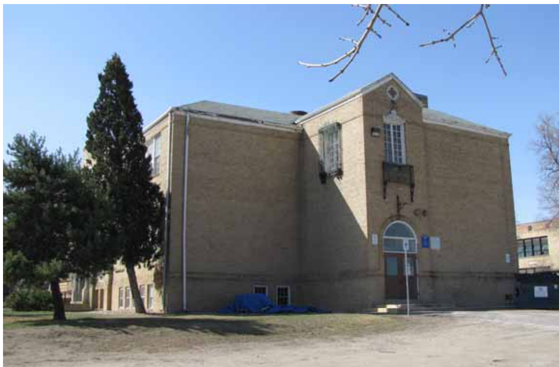
Photograph 4: New America School north façade, view to the Southwest
