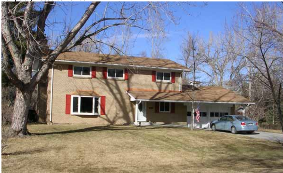
Photograph 1. South Façade, view looking North-Northeast
