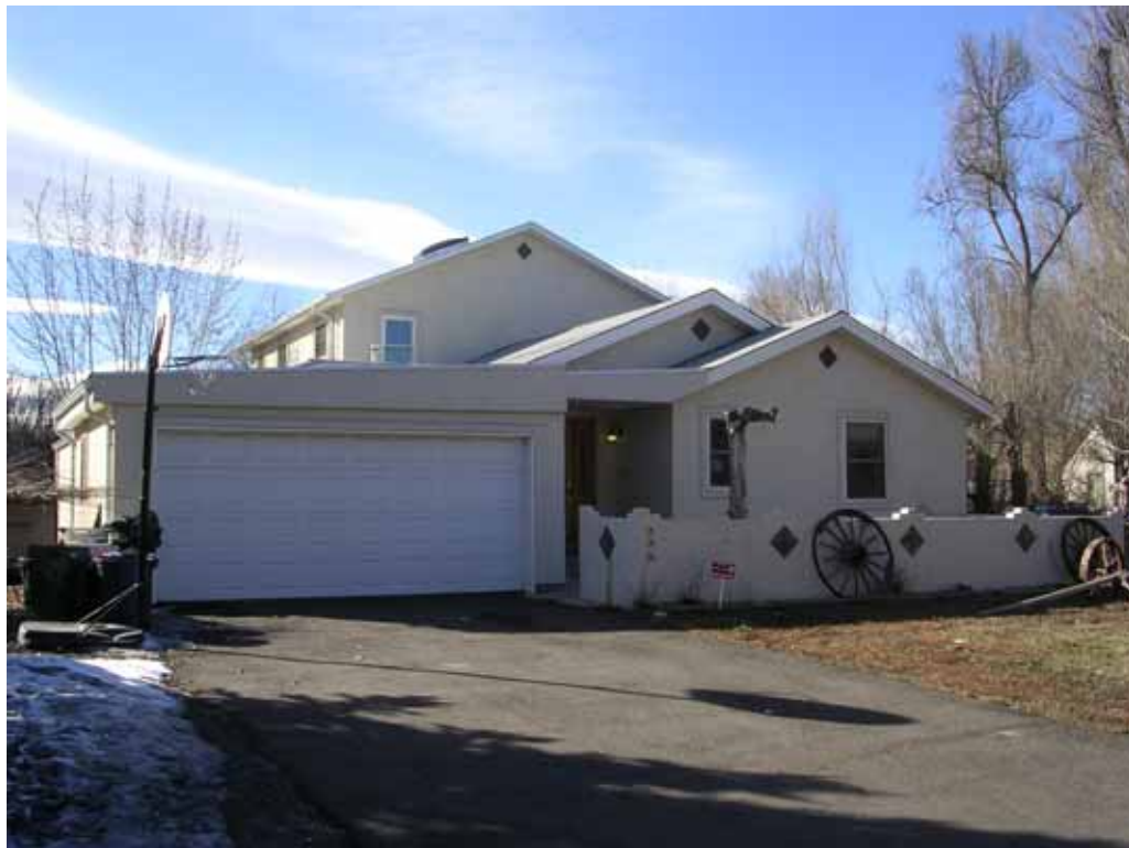
Photograph 1: East façade, view looking West, Northwest
