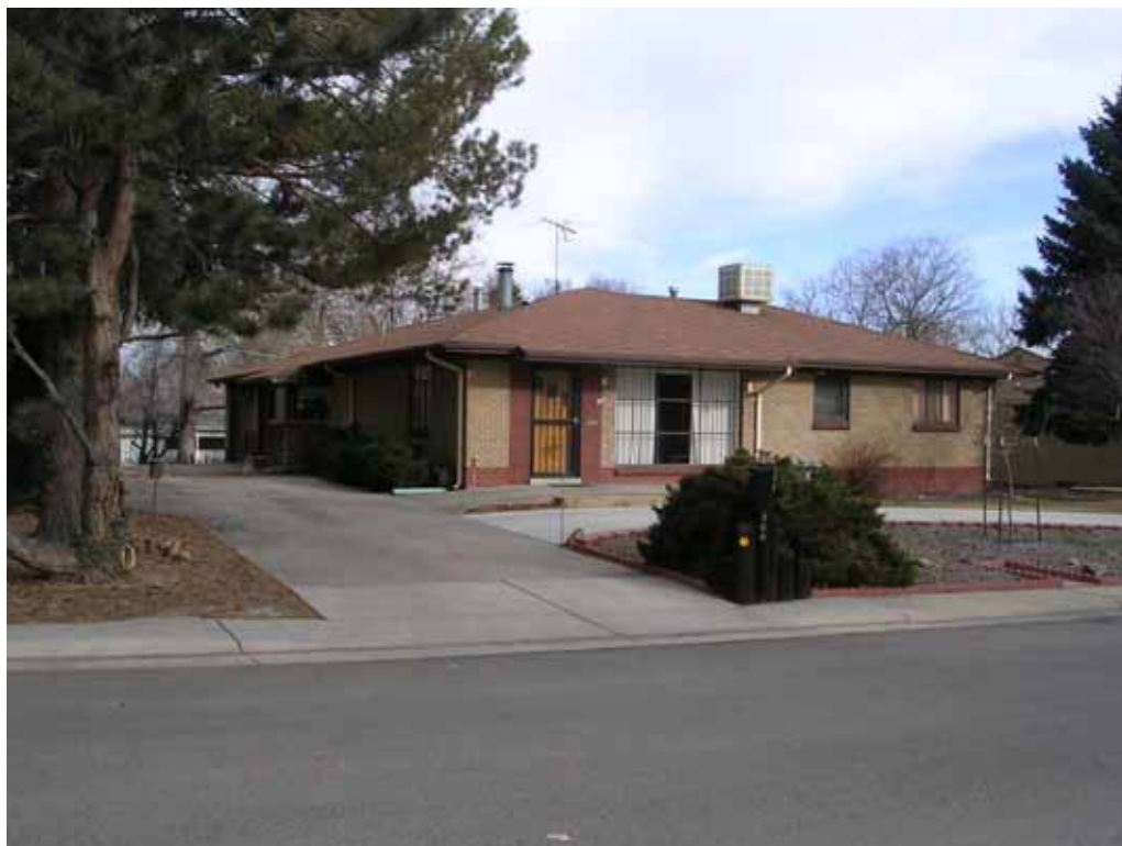
Photograph 1: West and North façades, view looking Southeast
