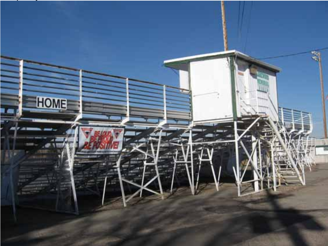
Photograph 43. Structure 16: Bleachers, view to the Northeast
