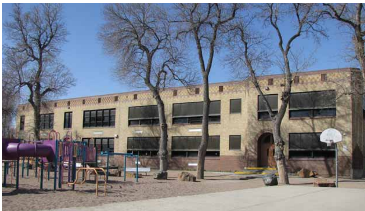
Photograph 8. Building 2: Elementary School, east façade, view to the Southwest
