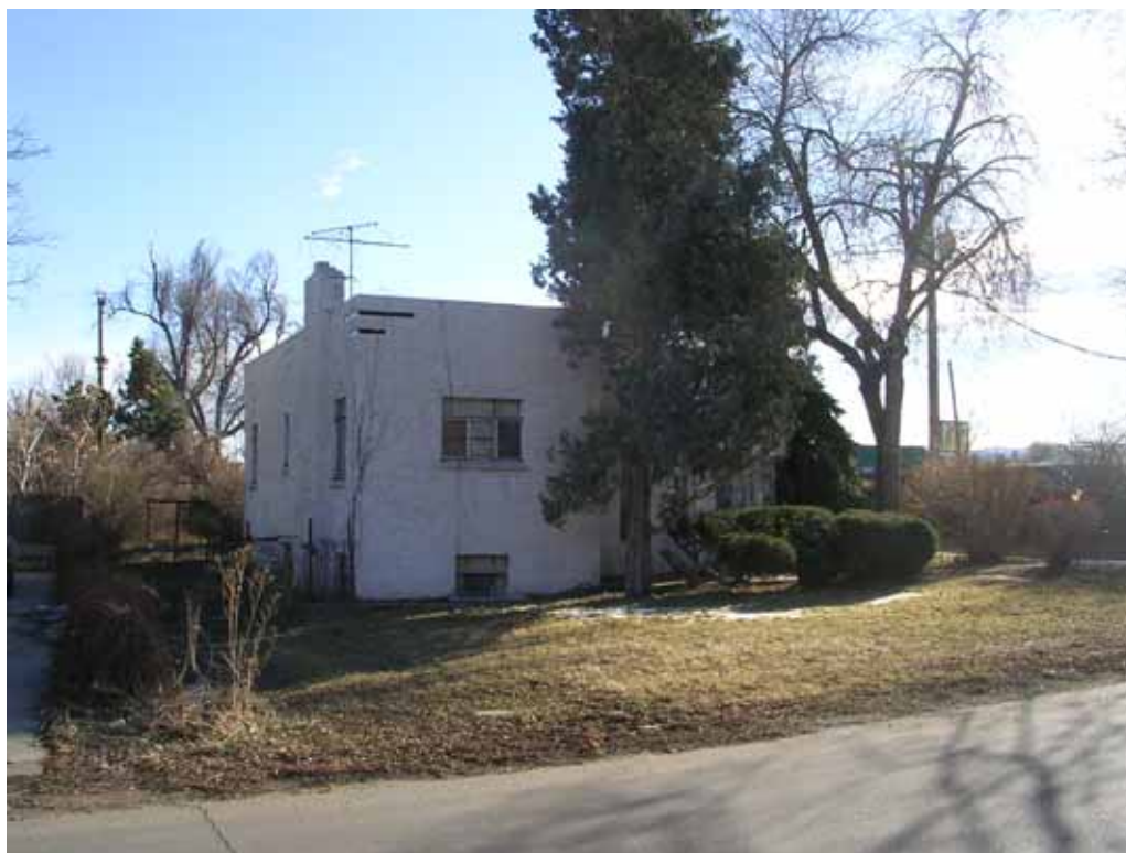
Photograph 2: North and East façades, view looking Southwest
