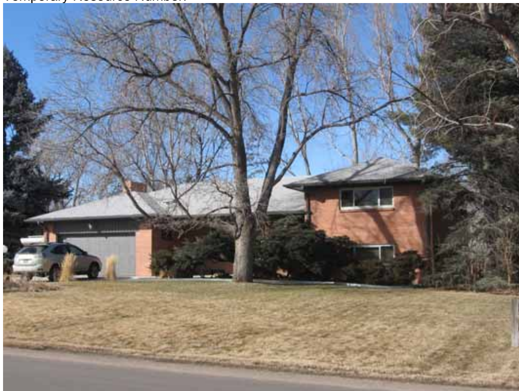
Photograph 1: South façade, view to the Northwest
