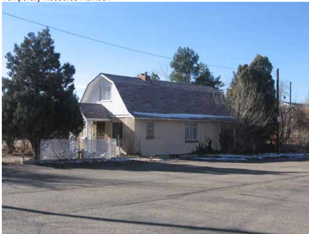
Photograph 3: North façade, view looking Southwest
