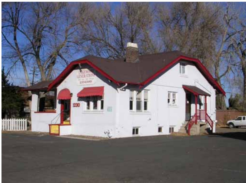
Photograph 2. West and South façades, view looking Northeast
