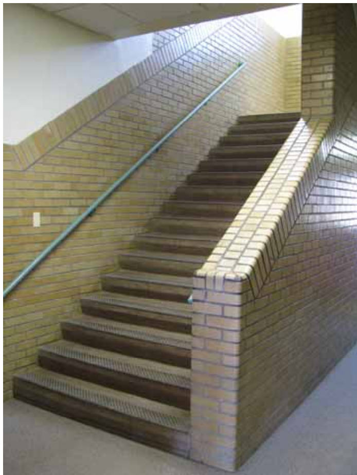
Photograph 11. Building 2: Elementary School, north stairwell
