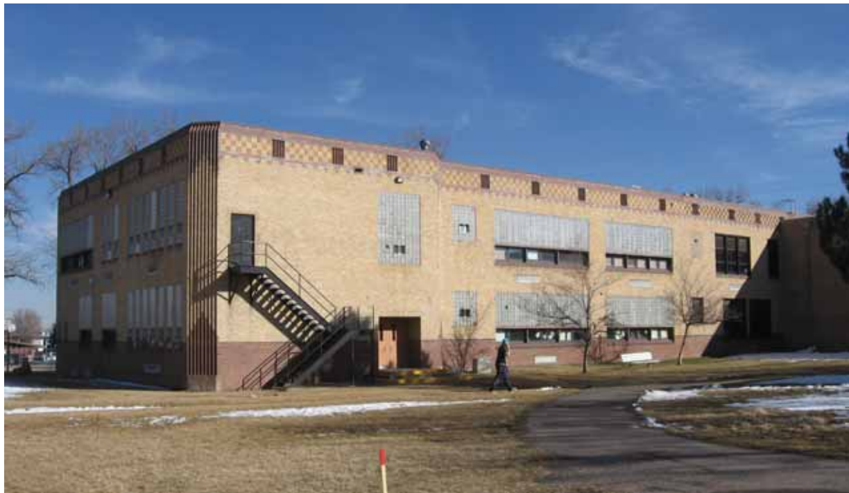
Photograph 9. Building 2: Elementary School, north and west façade, view to the Southeast
