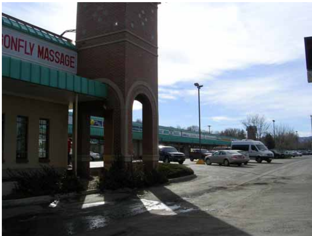
Photograph 3: North façade, view looking Southwest
