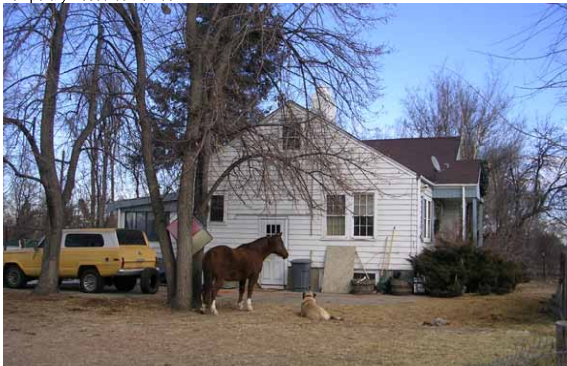
Photograph 3. West façade, view looking East
