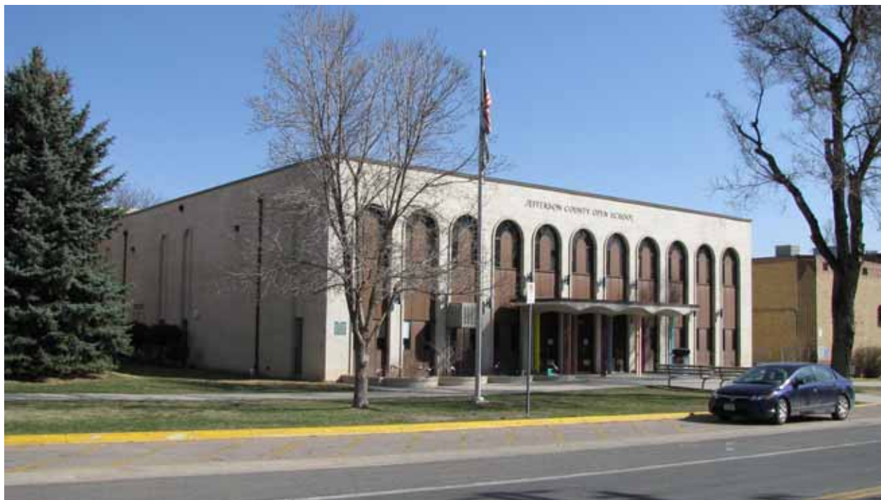
Photograph 18. Building 5: Administration and Arts Building, south and west façade, view to the Northeast
