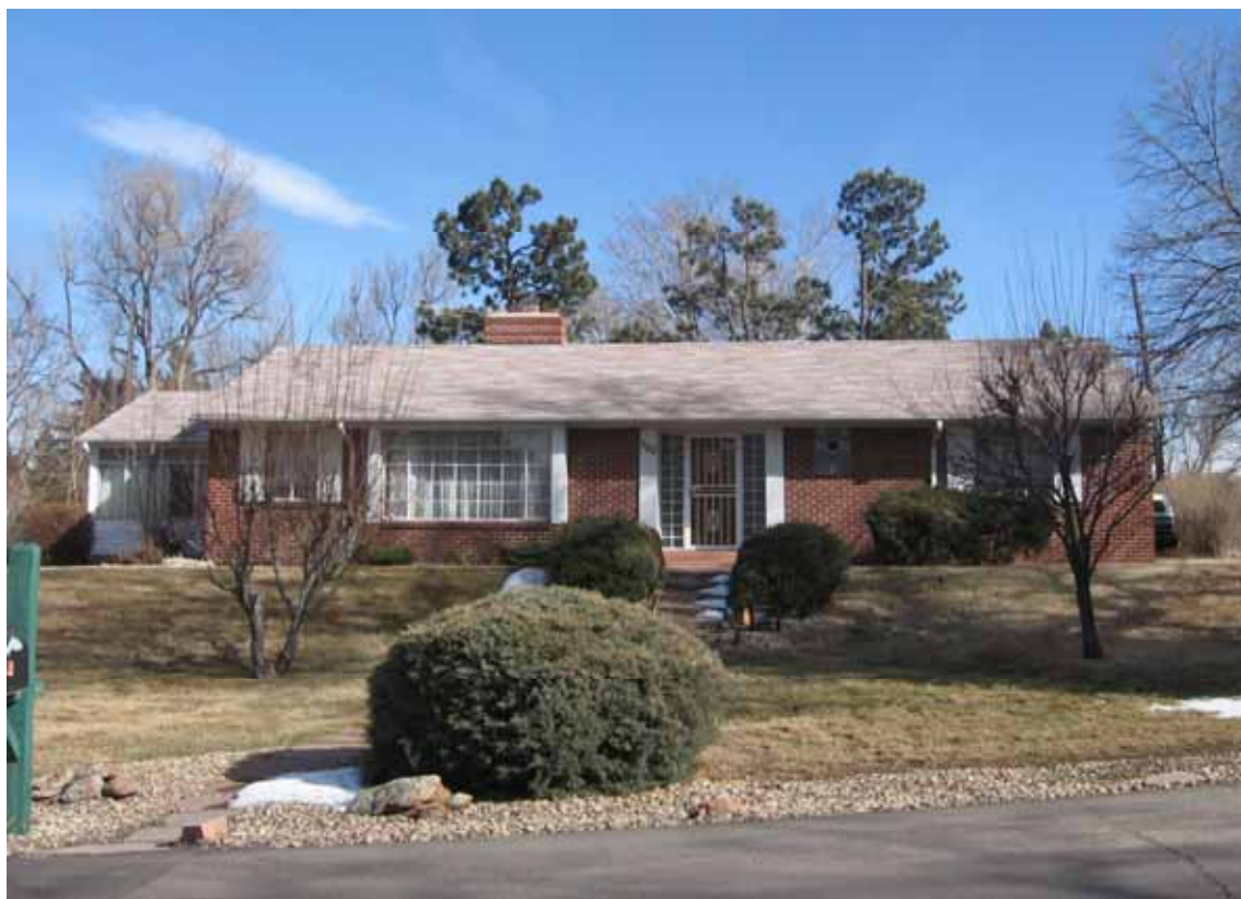
Photograph 2: West façade, view to the East
