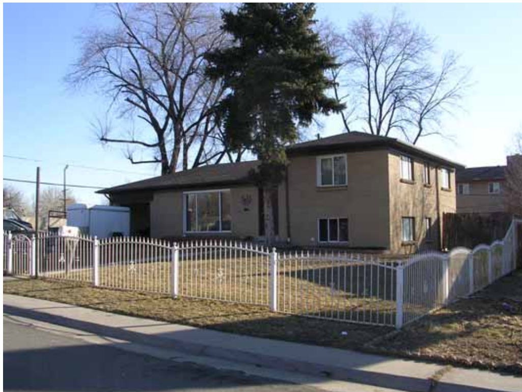
Photograph 1: West and South façades, view looking Northeast
