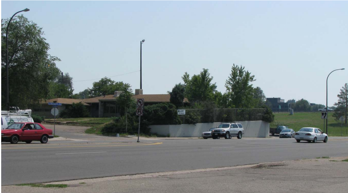
EXHIBIT 18 700 Wadsworth Blvd., view to the southeast across Wadsworth Boulevard
