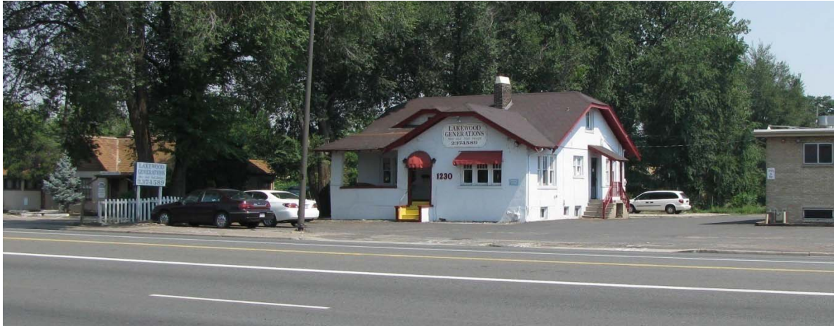
EXHIBIT 30 1230 Wadsworth Blvd., view to the northeast from across Wadsworth Boulevard
