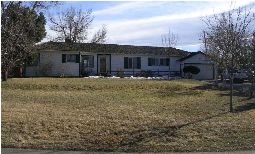
EXHIBIT 48 7500 Broadview Drive, view to the south from Broadview Drive
