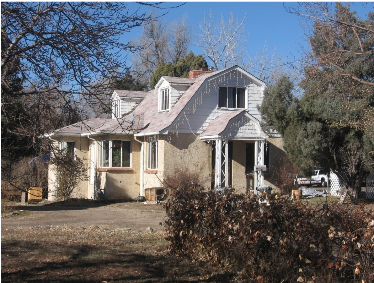
EXHIBIT 22 1215 Wadsworth Blvd., view to the northwest
