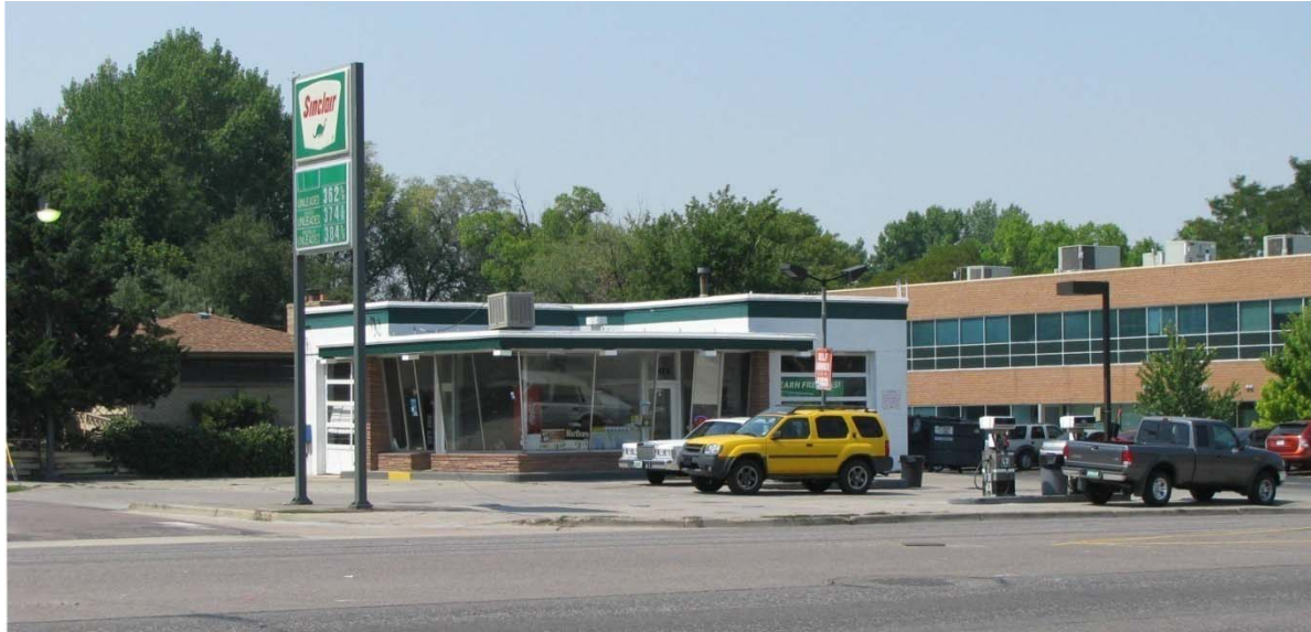
EXHIBIT 36 401 Wadsworth Blvd., view to the northeast from across Wadsworth Boulevard
