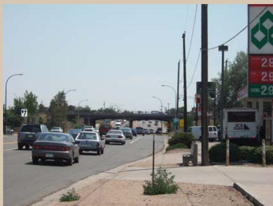
Traffic congestion, inefficient roadway operations, and poor pedestrian and bicycle facilities characterize the US 6/Wadsworth project area.
