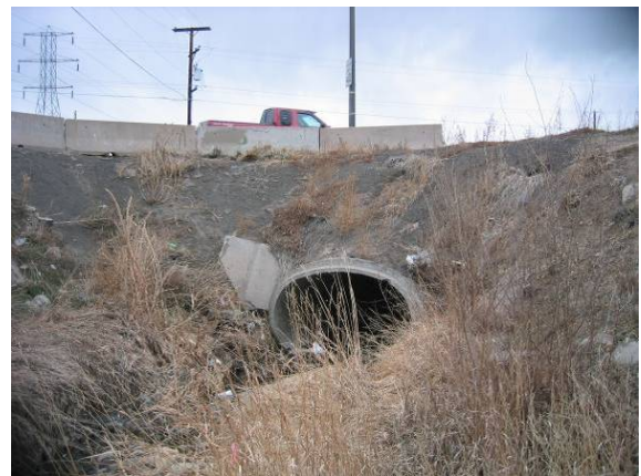
48 EXHIBIT 4-4: DRY GULCH CULVERT
