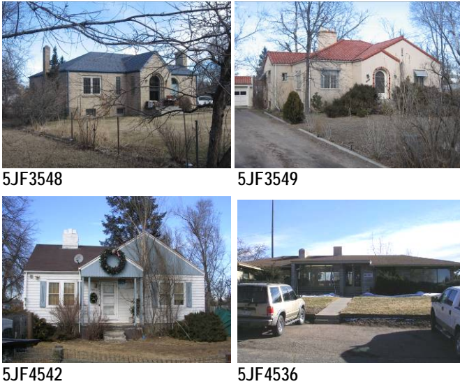
EXHIBIT 4-6: SECTION 4(F) HISTORIC PROPERTIES
