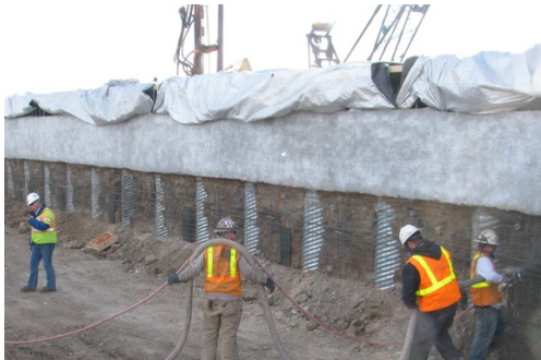
The west soil nail wall
