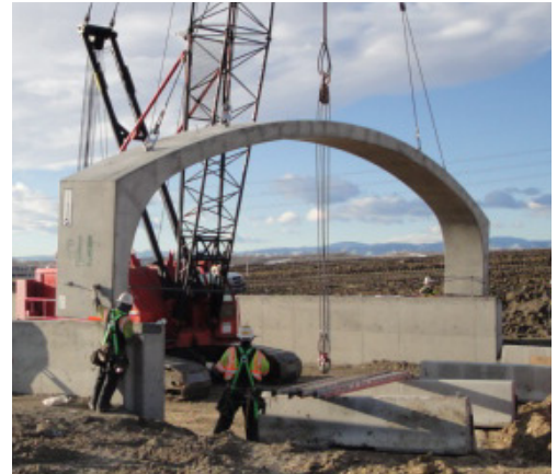
The completed pre-cast arch structure
