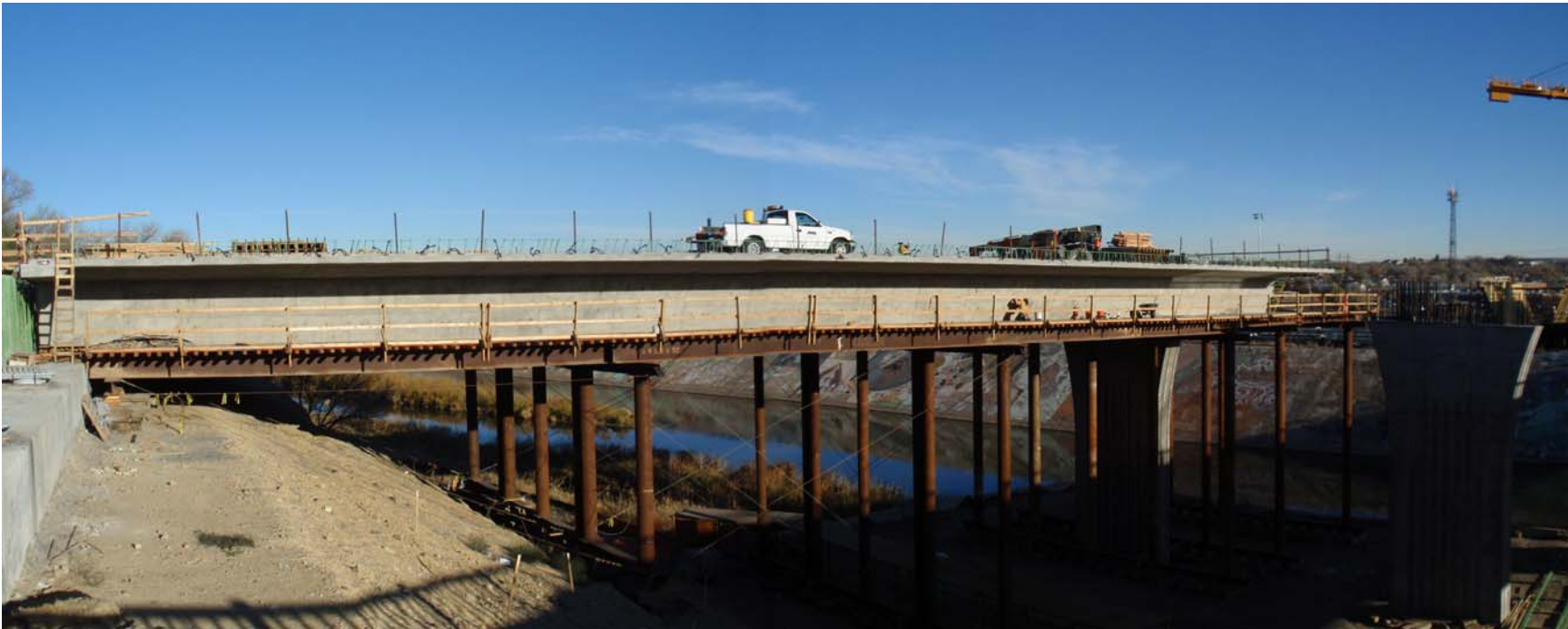
Figure 10 – Span 1 WB CIP Superstructure Construction – November 7, 2008:
