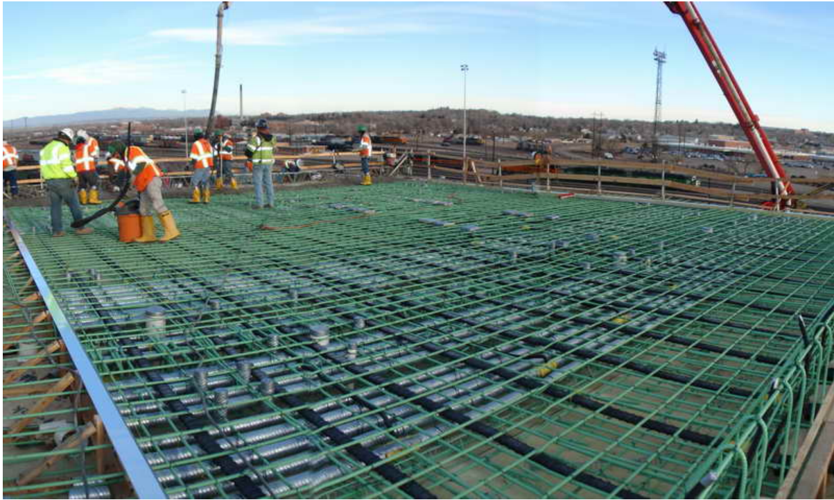
Figure 3 – Pier Table 3 WB Construction – December 31, 2008:
