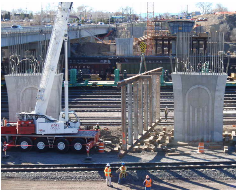
Figure 6 – Pier Table 4 WB Falsework Assembly – January 8, 2009:
