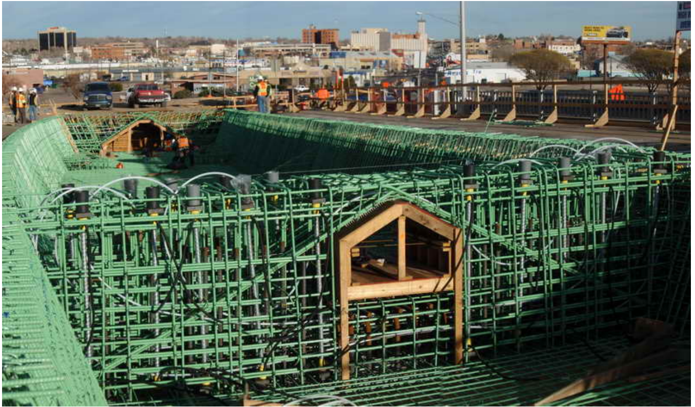
Figure 5 – Span 5 WB CIP Superstructure Construction – January 7, 2009:
