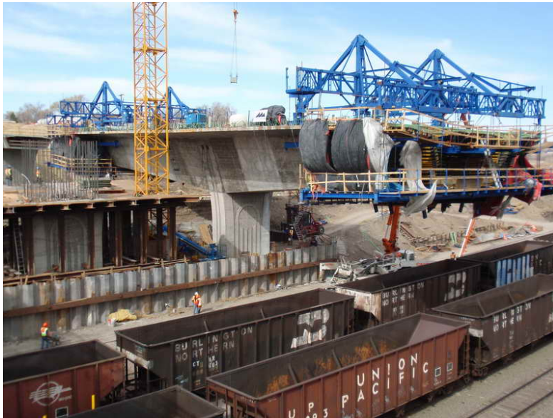
Figure 14 – Cantilever 3 WB Segmental Construction– April 9, 2009:
