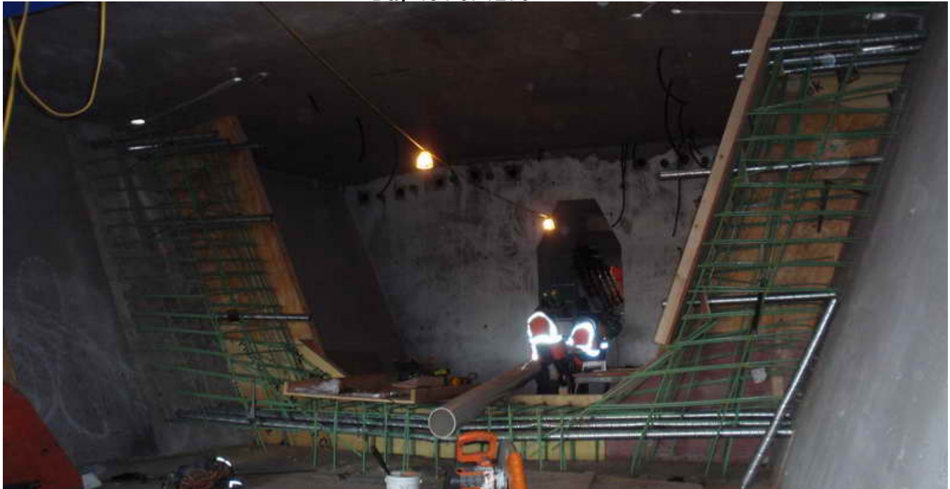
Figure 8 – Cantilever 3 WB Superstructure Construction – April 1, 2009:
