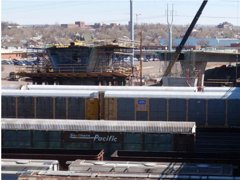
Figure 10 – Pier Table 4 WB Construction– April 6, 2009:
