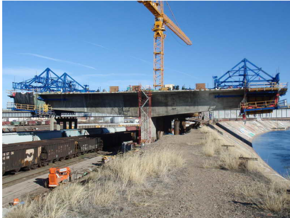
Figure 16 – Cantilever 3 WB Segmental Construction –April 13, 2009:
