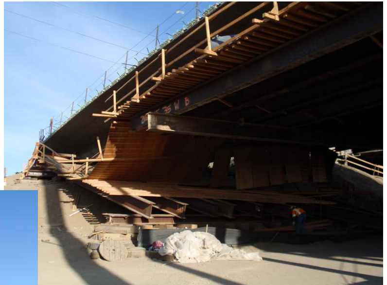
Figure 3 – Span 5 WB Falsework Removal – March 25, 2009:
