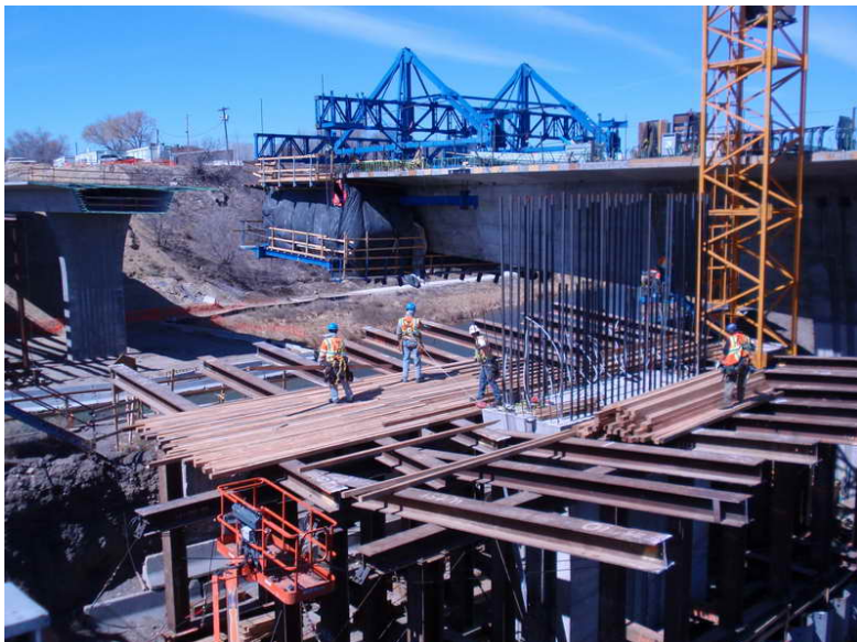
Figure 12 – Pier Table 3 EB Construction– April 7, 2009:
