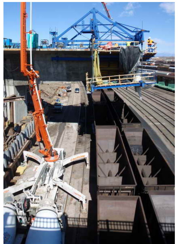
Figure 5 – Cantilever 3 WB Segmental Construction – March 31, 2009:
