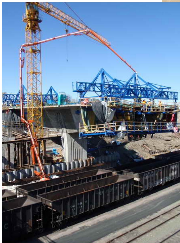
Figure 4 – Cantilever 3 WB Segmental Construction – March 31, 2009:
