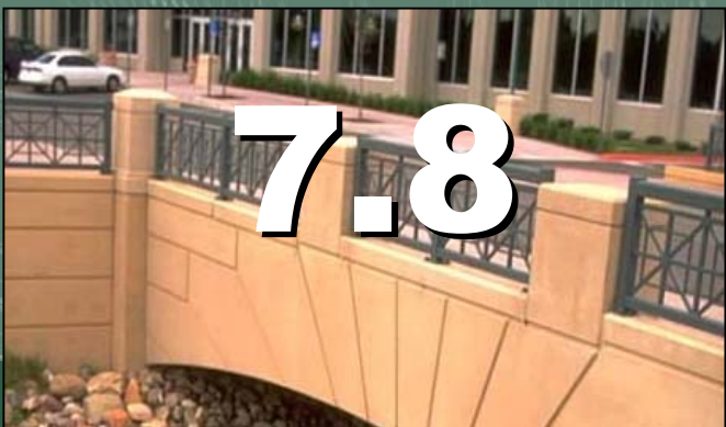
Option 3 Parapet w/ Open Railing
