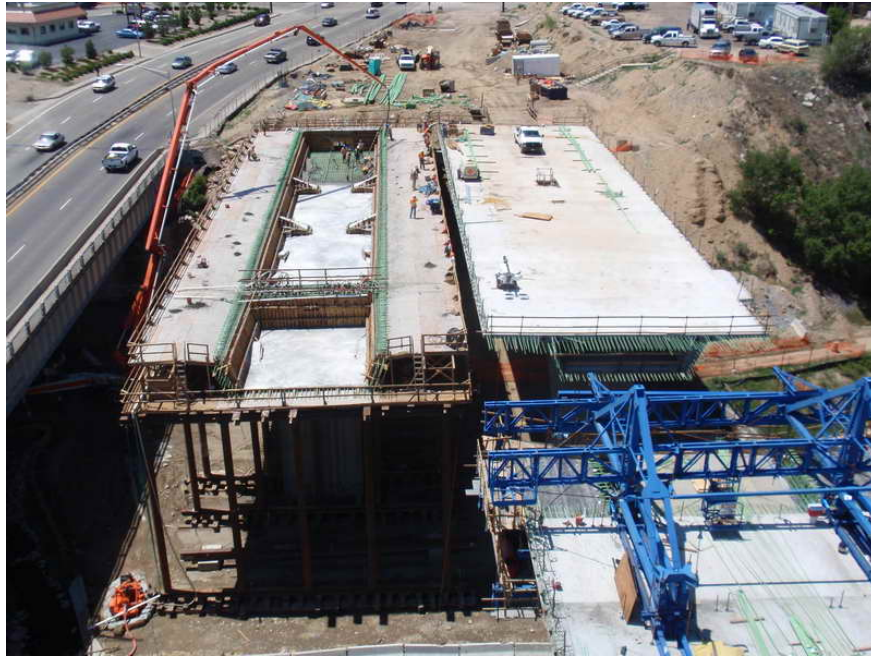
Figure 5 – Span 1 EB CIP Superstructure Construction – May 27, 2009:
