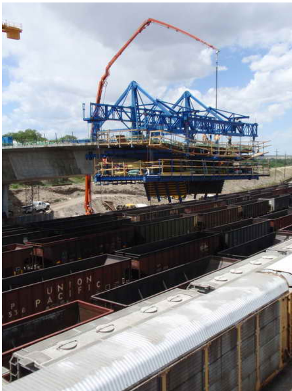
Figure 3 – Cantilever 3 WB – May 15, 2009: A 61-meter concrete pump truck delivers the concrete for Segment W3-8E, while the UPRR stores several empty coal trains under the cantilever.
