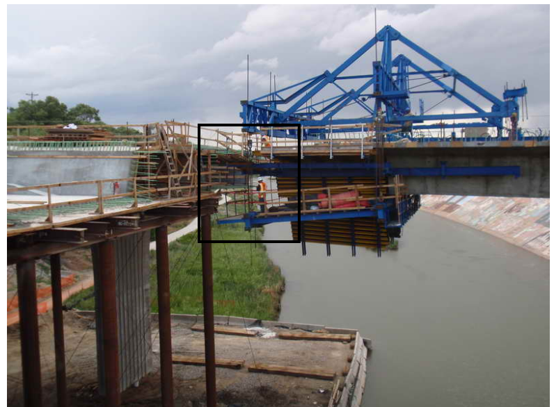
Figure 11( A & B) – Cantilever 3 WB Segmental Construction – June 11, 2009:
