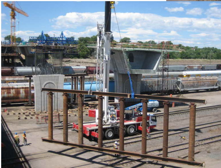
Figure 8 – Pier Table 4 EB Falsework Construction – June 5, 2009:
