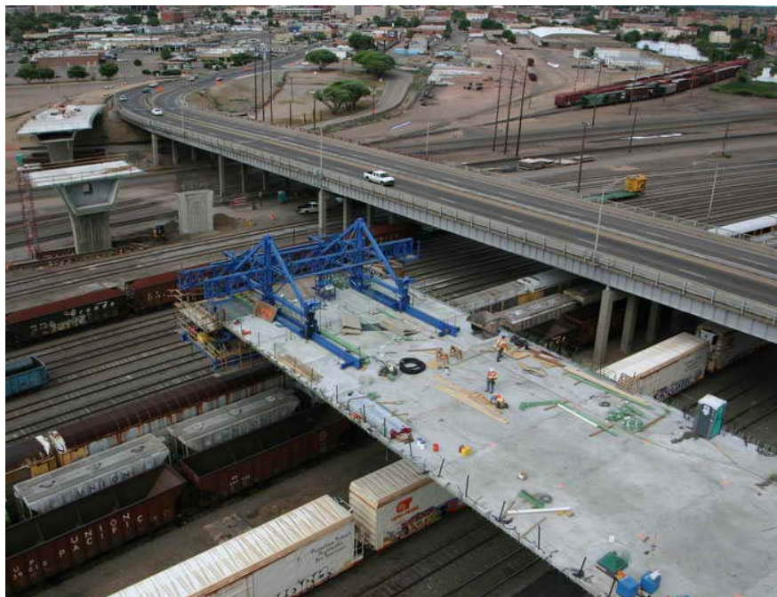
Figure 6 – Cantilever 3 WB Segmental Construction – June 1, 2009:
