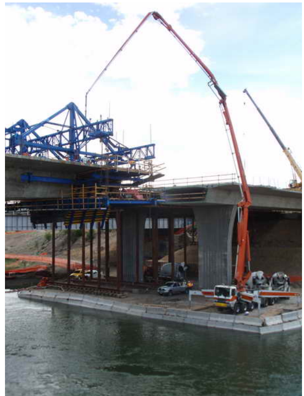
Figure 4 – Cantilever 3 WB – May 20, 2009: Segment W3-8W in the side span is placed via the 52-meter pump set up below Span 1 WB.
