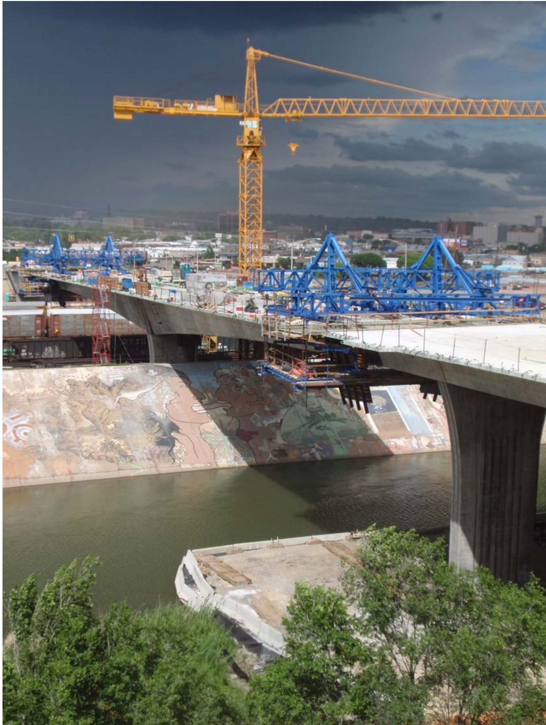
Figure 12 – Cantilever 3 WB Segmental Construction – June 11, 2009: Dark skies threaten to drop rain and hail on the jobsite, as the form traveler crew finishes launching the side-span traveler. Span 2 WB closure segment concrete is scheduled to be placed later this month.
