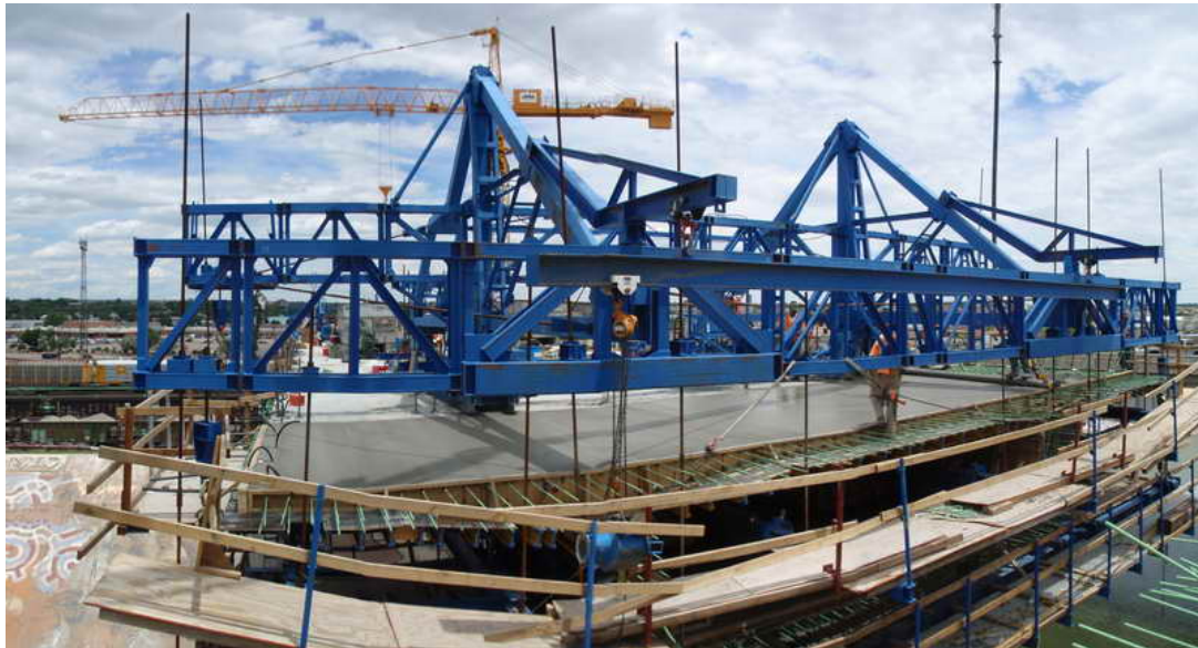
Figure 10 – Cantilever 3 WB Segmental Construction – June 9, 2009:
