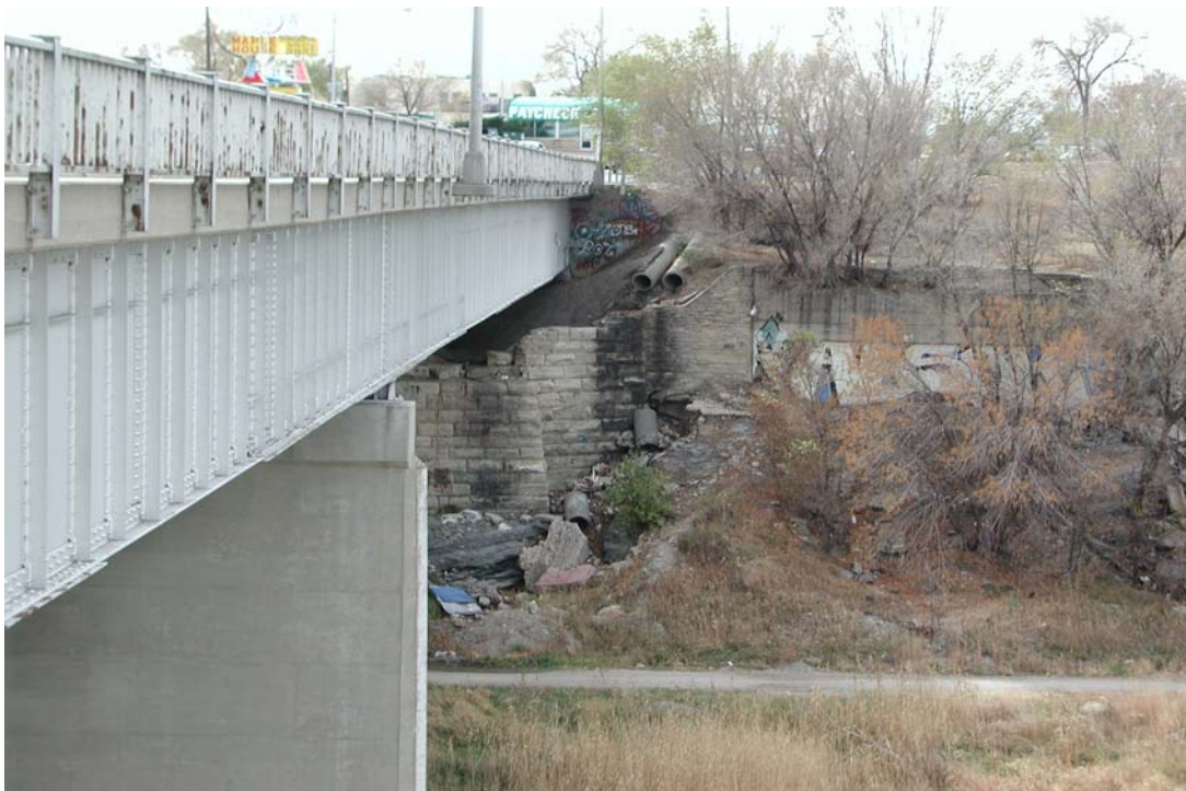
Figure 2.6 Storm Sewer Outfall at West Abutment
