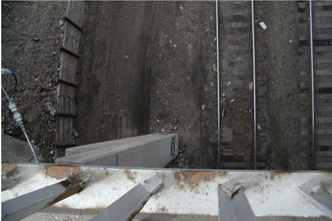
Figure 2.5 Proximity of Pier 5 to UPRR Yard Track 21 and Floodwall
