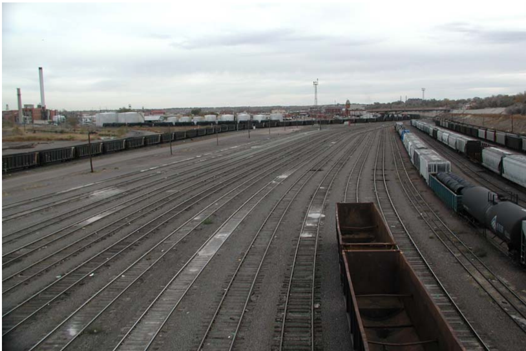
Figure 2.2 Pueblo Yard Looking South
