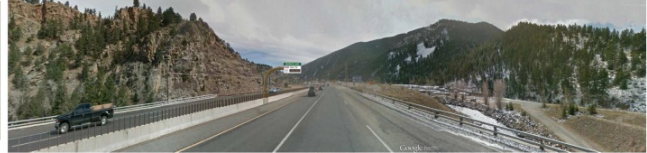
EXPRESS LANE TOLL SIGN FOR RE-ENTRY AFTER IDAHO SPRINGS
