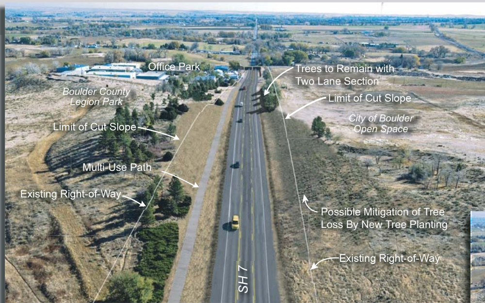
View Over the Hill With Cut Slopes
