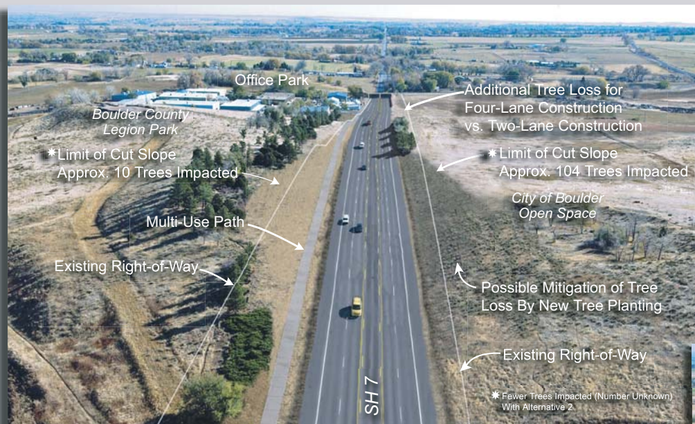
View Over the Hill With Cut Slopes
