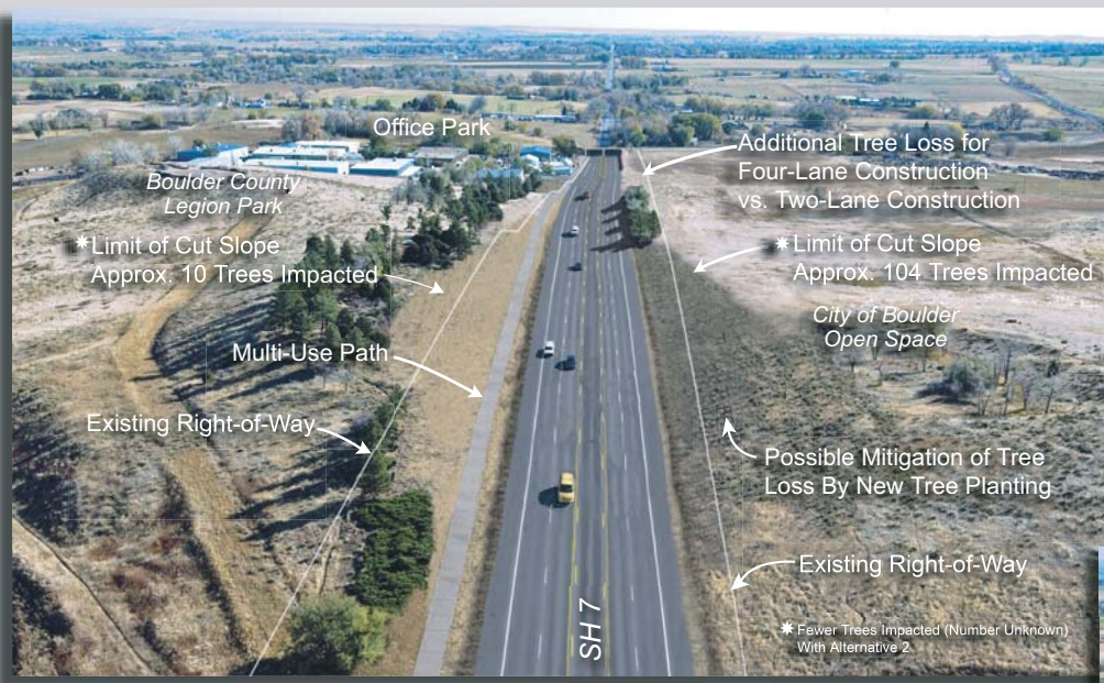
View Over the Hill With Cut Slopes
