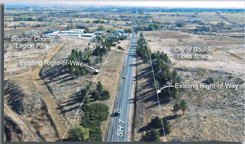
Existing View of SH 7 From Westview Looking East
