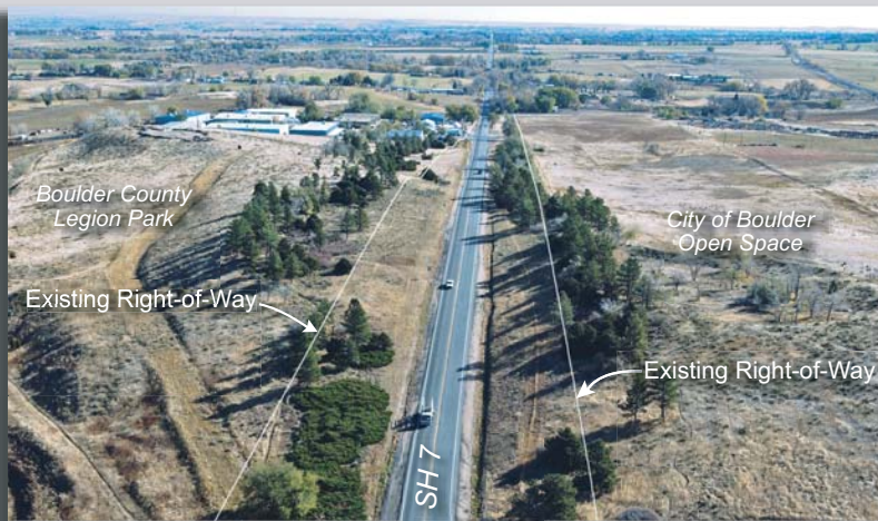
Existing View of SH 7 From Westview Looking East
