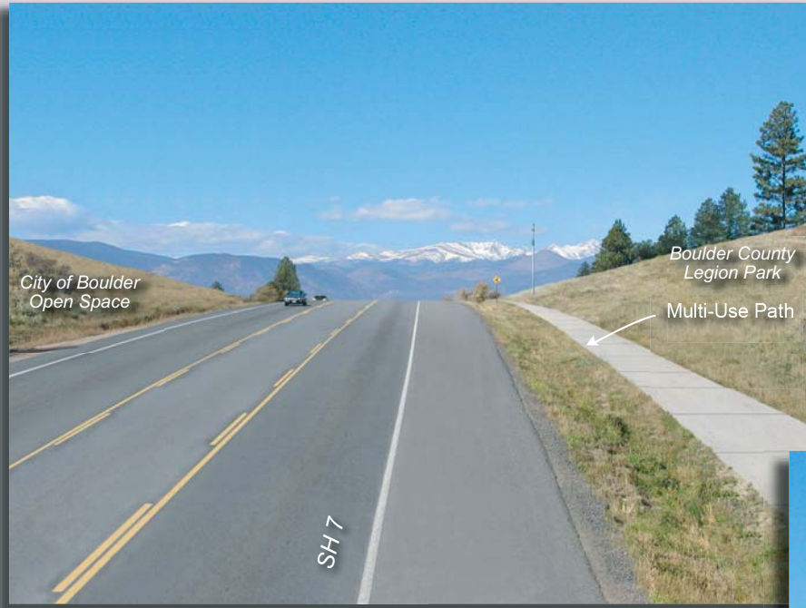
View Over the Hill With Cut Slopes
