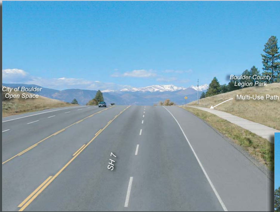
View Over the Hill With Cut Slopes
