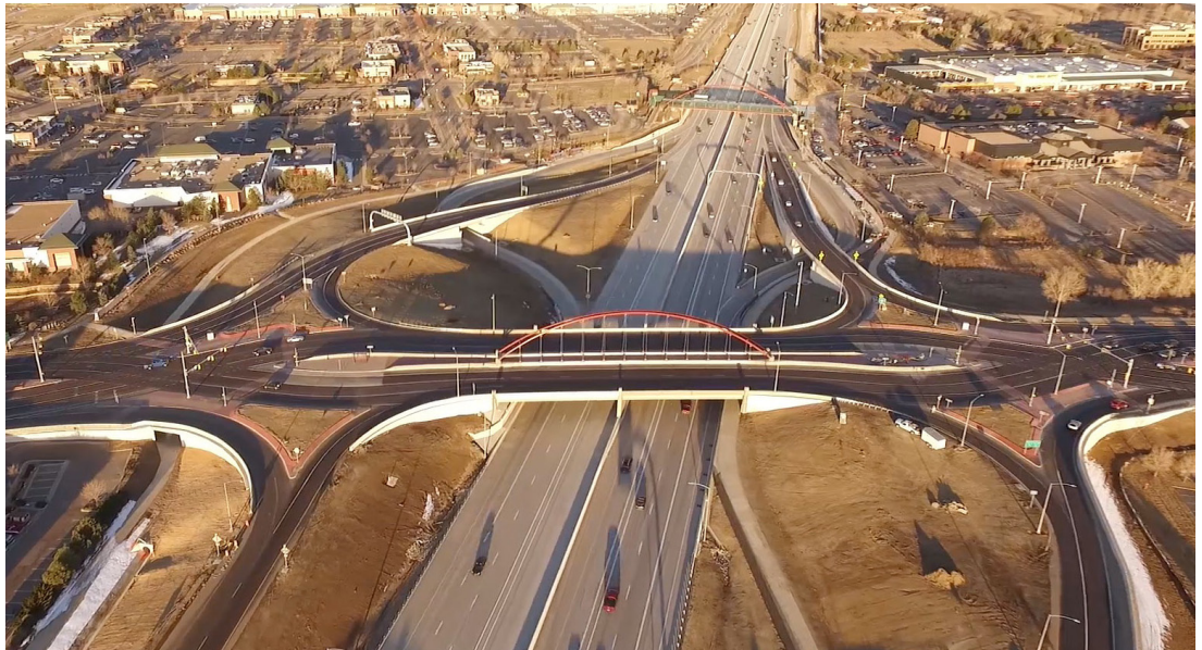
Completed Diverging Diamond Interchange at McCaslin Boulevard
