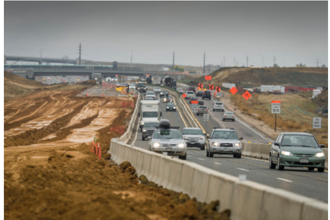
Eastbound paving preparations Photo courtesy of HDR, Inc. © 2013 Keith Philpott
