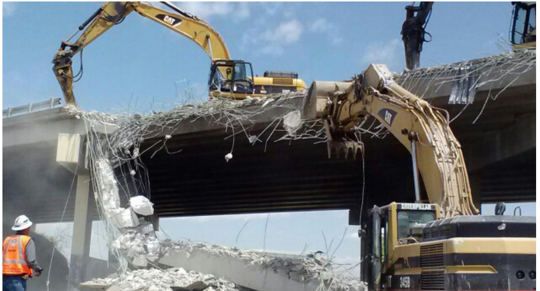
Burlington Northern Santa Fe (BNSF) bridge demolition
