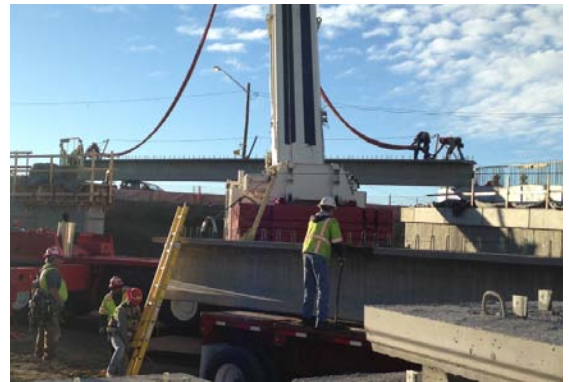
Placing girders for the new McCaslin Boulevard Diverging Diamond Interchange
