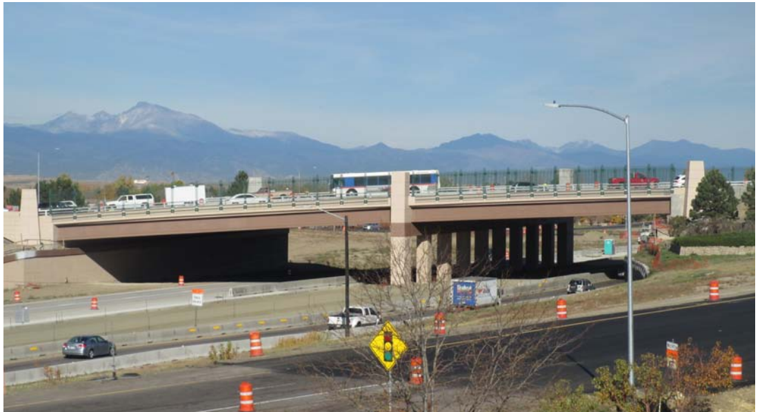
The newly reconstructed Sheridan Boulevard bridge
