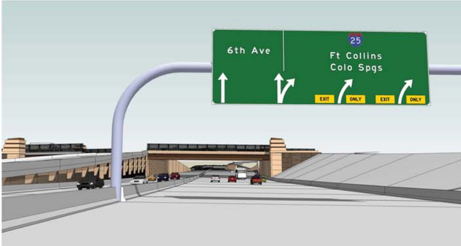
View of Federal Bridge Looking Eastbound from US 6
