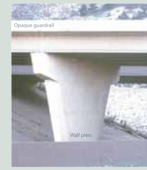
C-470 @ S.H. 285 overpass
