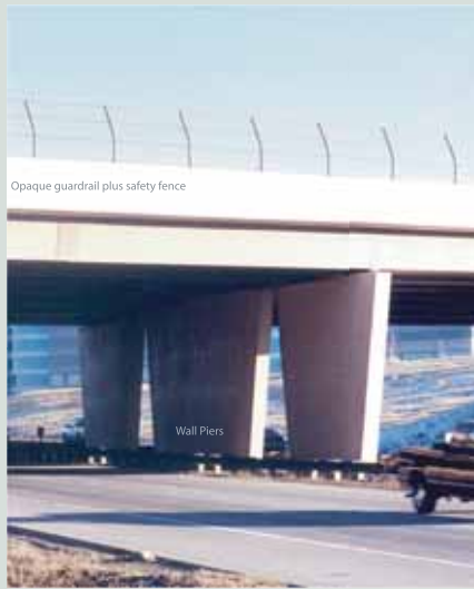
C-470 @ Lucent overpass
