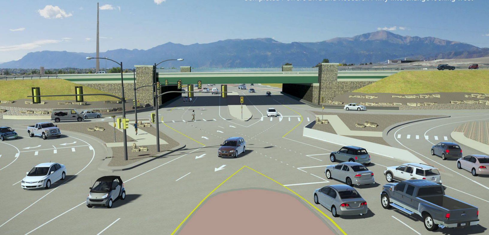
Completed Powers Blvd and Research Pkwy Interchange looking west
