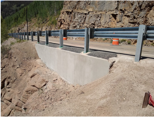
CO 145 - Retaining wall, guardrail and highway repairs at two sites near mile point 49.5 are now complete.
