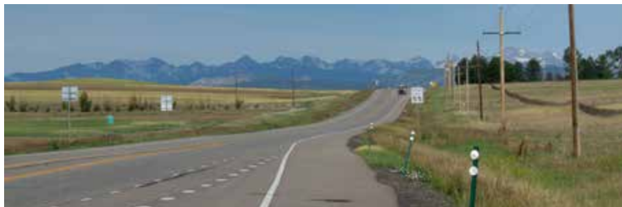
CO 52 (MP 3) looking west along corridor
