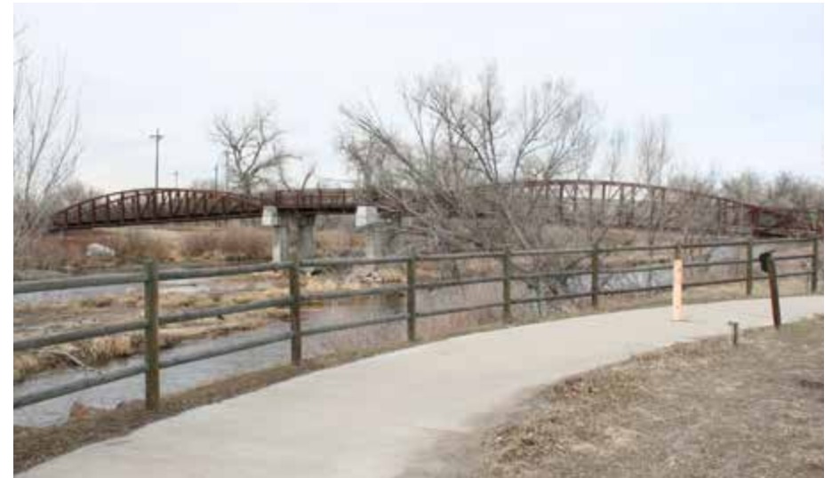
Looking northwest at pedestrian bridge over South Platte River in Fort Lupton
