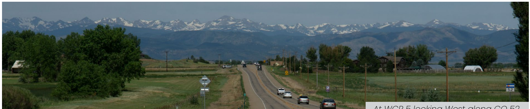
At WCR 5 looking West along CO 52
