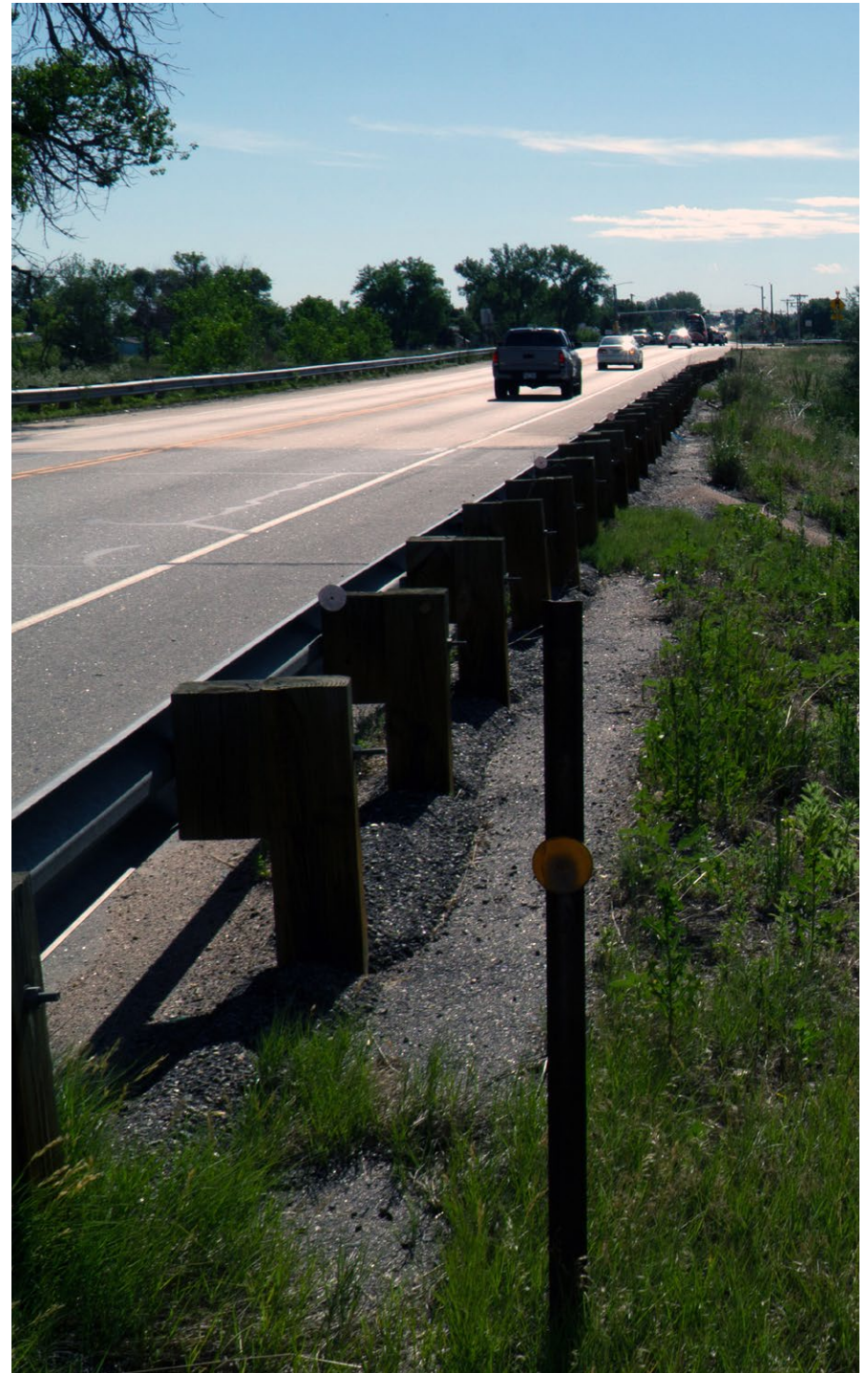
Existing Guardrail along CO 52 , West of County Line Road
