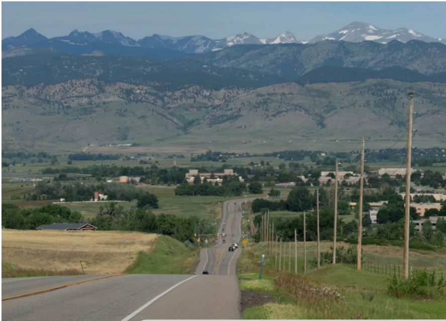
CO 52 East of 79th Street Looking West
