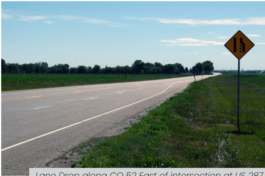
Lane Drop along CO 52 East of intersection at US 287
