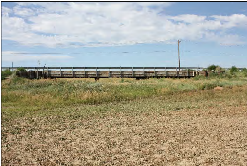
Photograph 8. Downstream Bridge Face Looking Southwest
