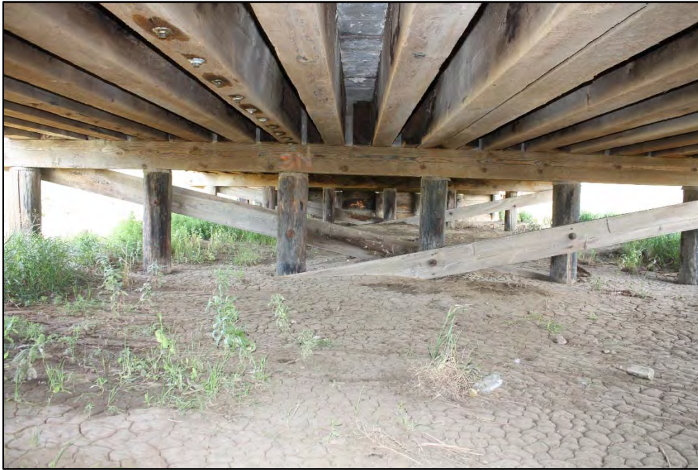
Photograph 17. Bridge Stringers and Bents Looking Northwest
