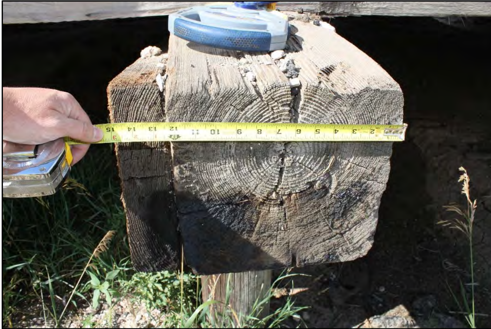
Photograph 19. Typical Pier Cap and Pier
