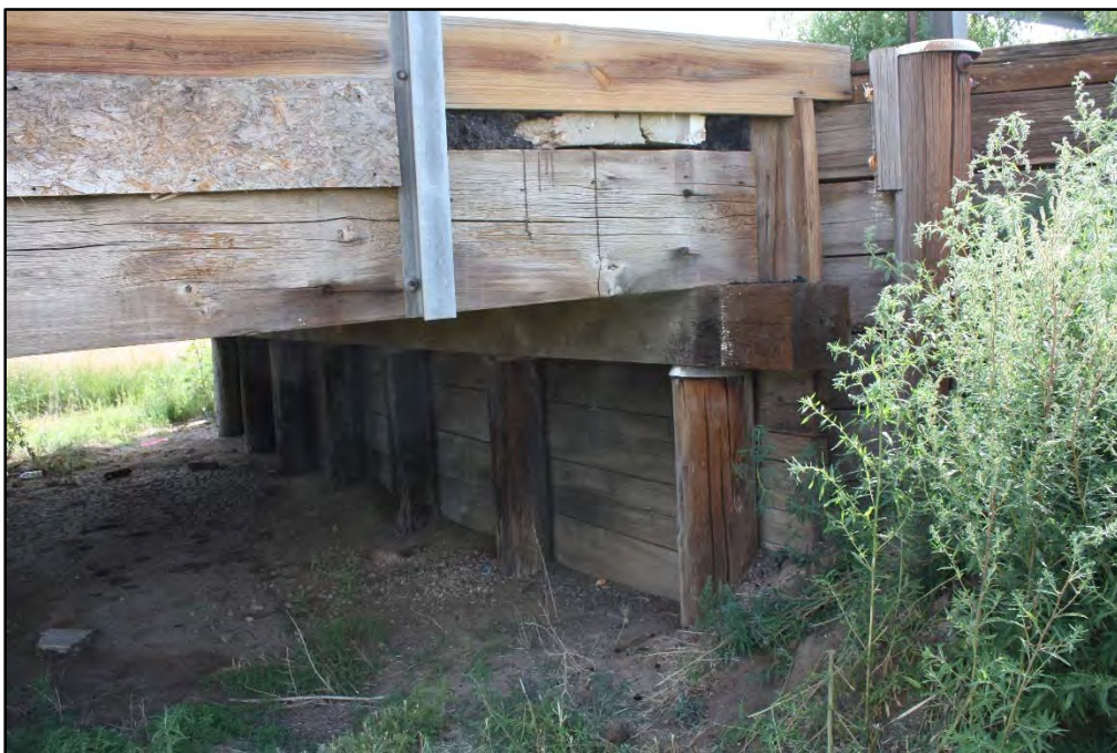
Photograph 14. East Abutment Backwall (Upstream) Looking East
