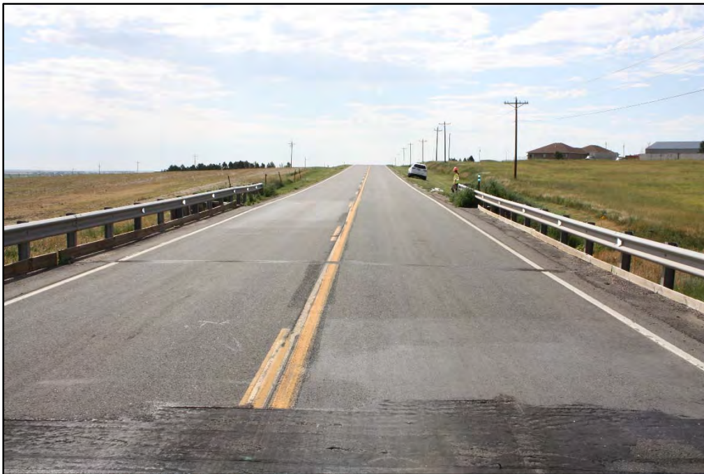
Photograph 6. Bridge Deck Looking Southeast
