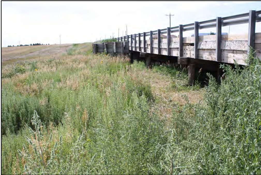
Photograph 11. Downstream Bridge Face Looking South
