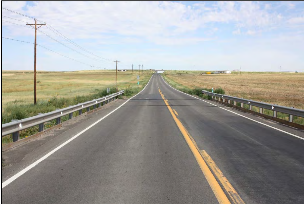
Photograph 5. Bridge Deck Looking Northwest
