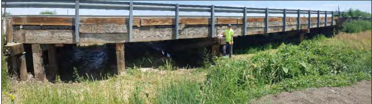
Figure 3. View looking downstream at US36 Bridge F-19-E near Strasburg, CO.
