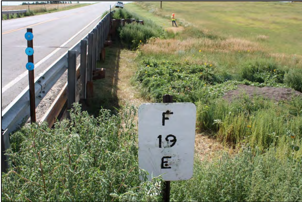
Photograph 3. Upstream Embankment Looking Southeast
