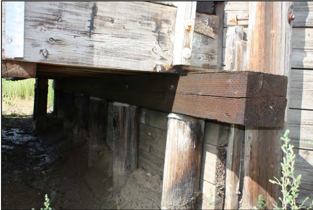
Photograph 15. West Abutment Backwall (Downstream) Looking West
