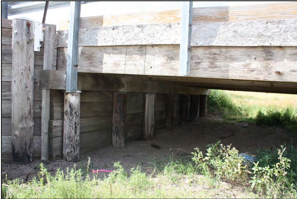
Photograph 13. East Abutment Backwall (Downstream) Looking South
