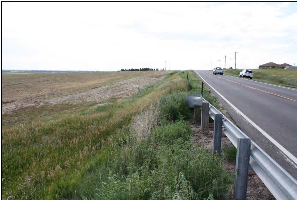
Photograph 4. Downstream Embankment Looking Southeast
