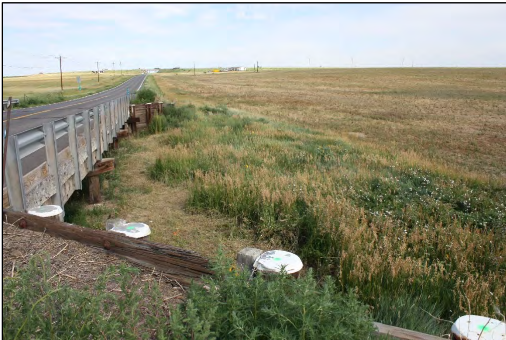
Photograph 2. Downstream Embankment Looking Northwest
