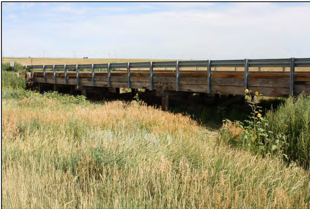
Photograph 10. Upstream Bridge Face Looking North
