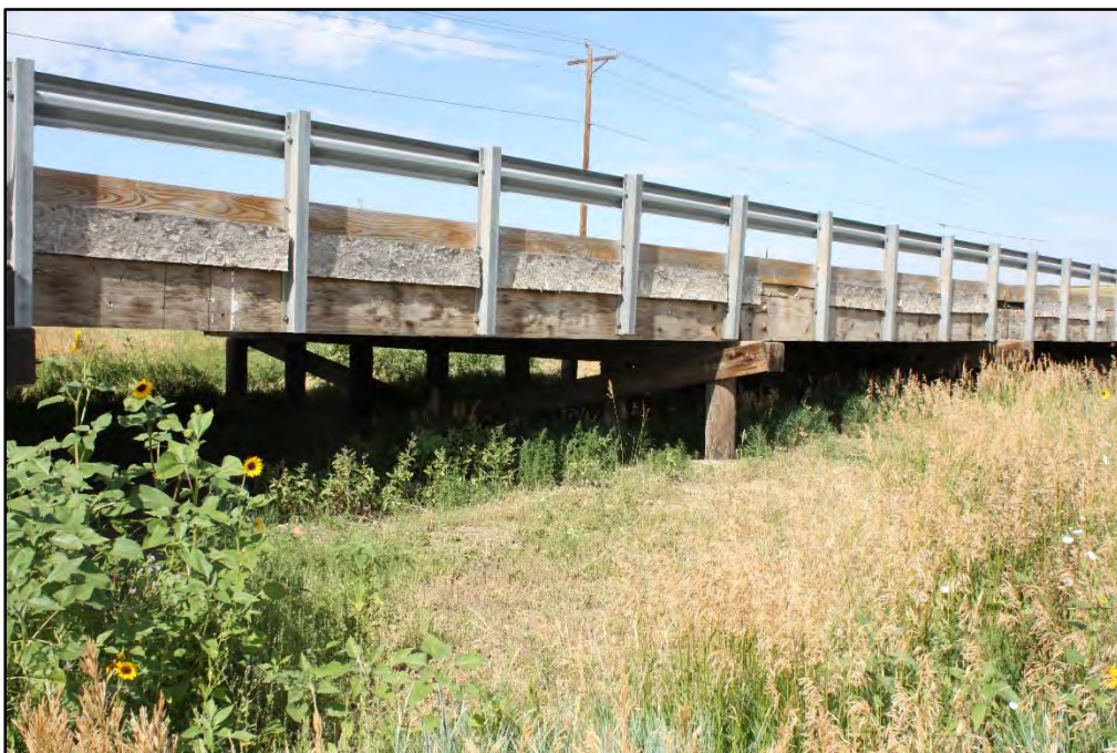
Photograph 12. Downstream Bridge Face Looking West
