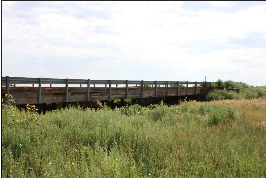
Photograph 9. Upstream Bridge Face Looking East
