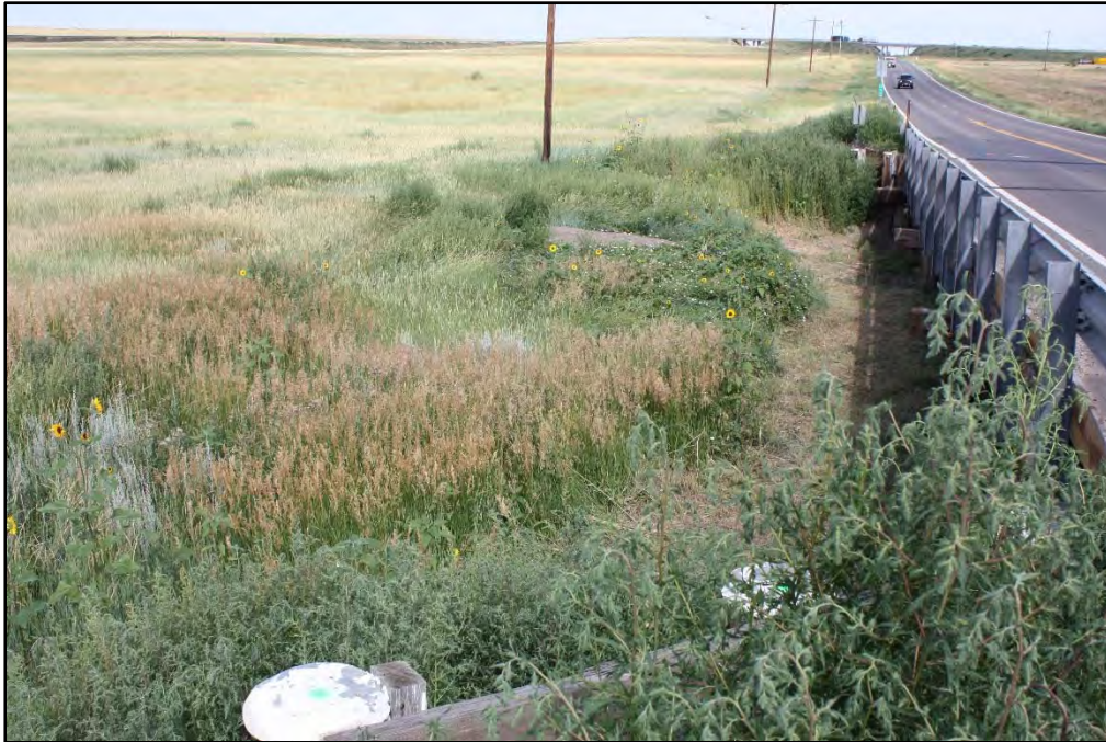
Photograph 1. Upstream Embankment Looking Northwest
