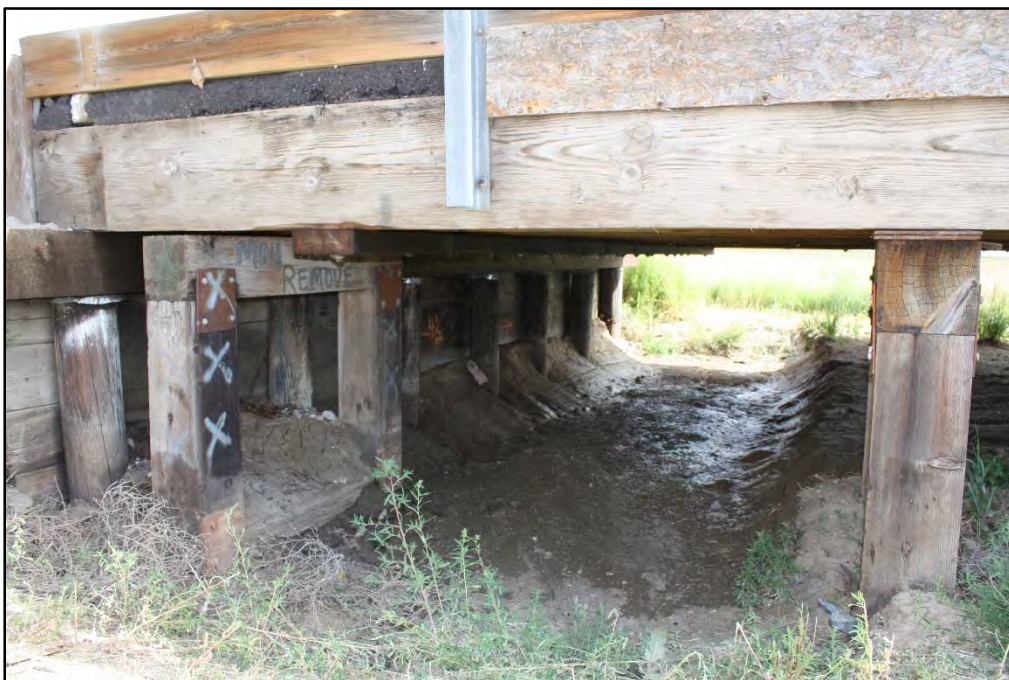
Photograph 16. West Abutment Backwall (Upstream) and Excavation Looking North
