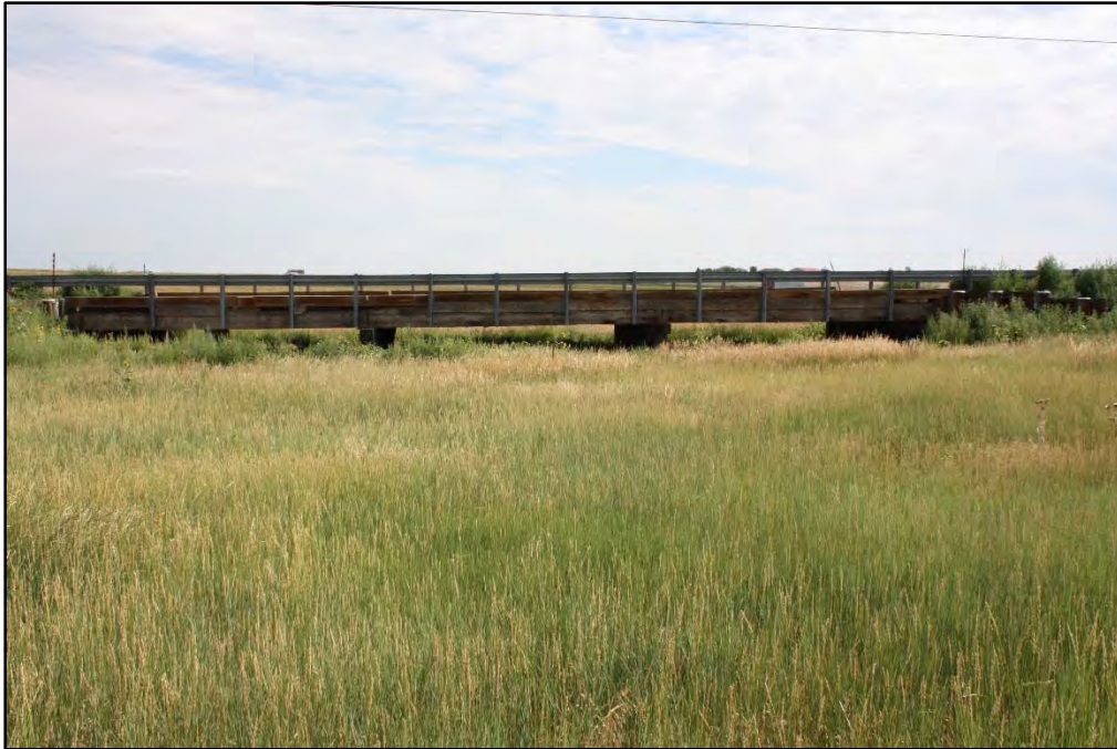
Photograph 7. Upstream Bridge Face Looking Northeast
