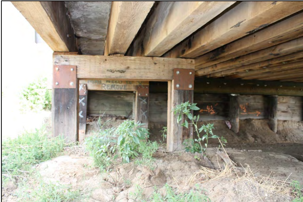
Photograph 18. Helper Bents Looking Northwest
