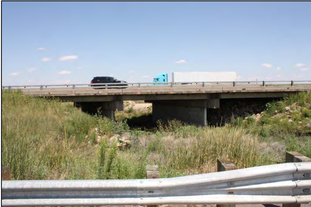
Photograph 14. Upstream Face of Downstream East Bound I-70 Bridge Looking Northeast
