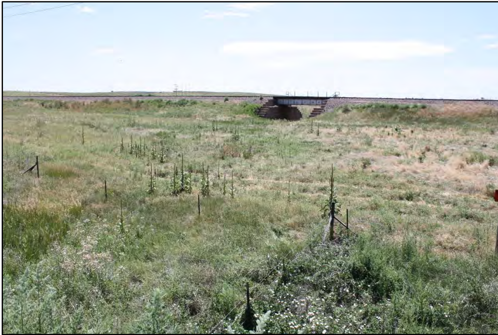
Photograph 15. Upstream UPRR Embankment and Floodplain Looking Southeast
