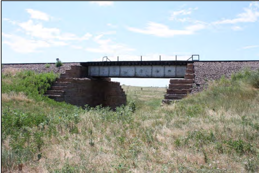
Photograph 12. Upstream UPRR Bridge Looking Southwest
