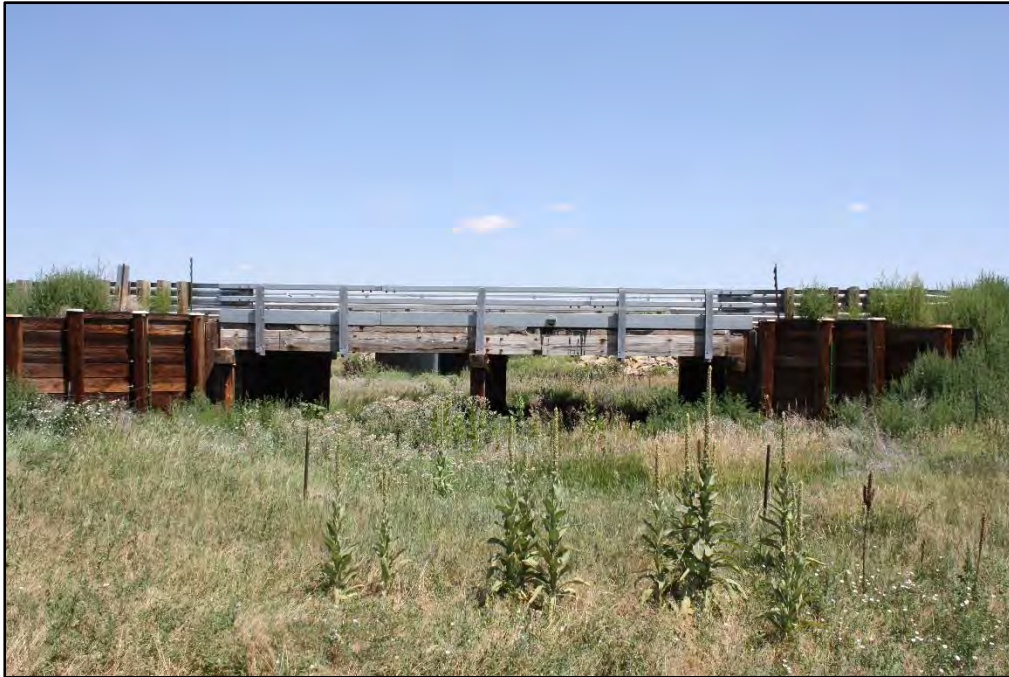
Photograph 7. Upstream Bridge Face Looking Northeast
