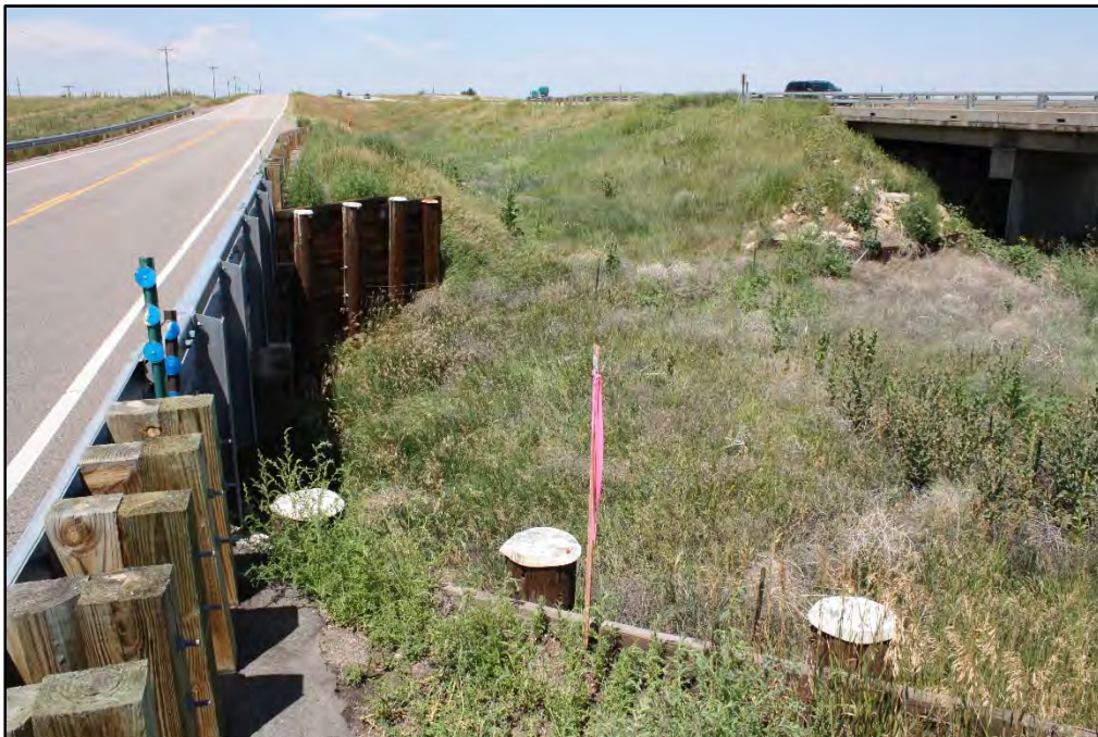
Photograph 2. Downstream Embankment Looking Northwest
