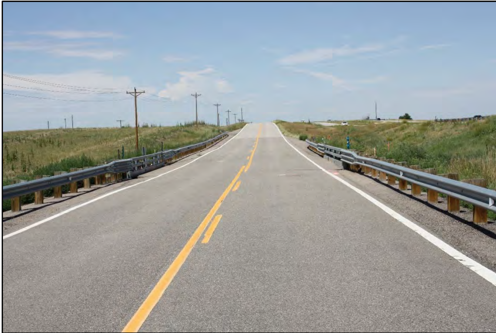
Photograph 5. Bridge Deck Looking Northwest
