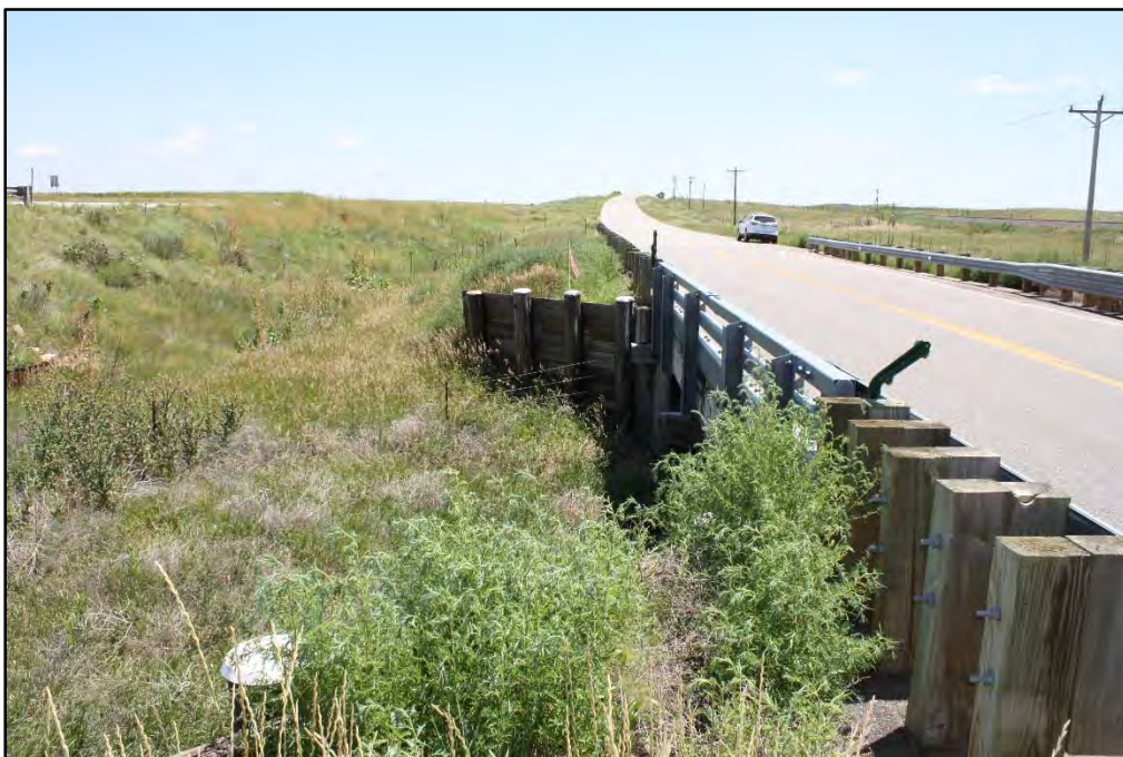
Photograph 4. Downstream Embankment Looking Southeast
