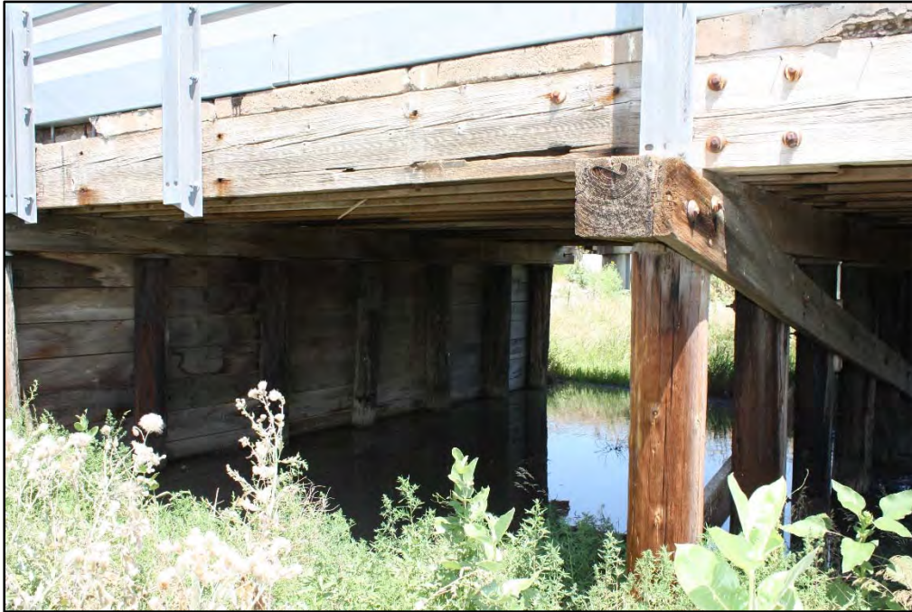
Photograph 9. West Abutment Backwall (Upstream) Looking North
