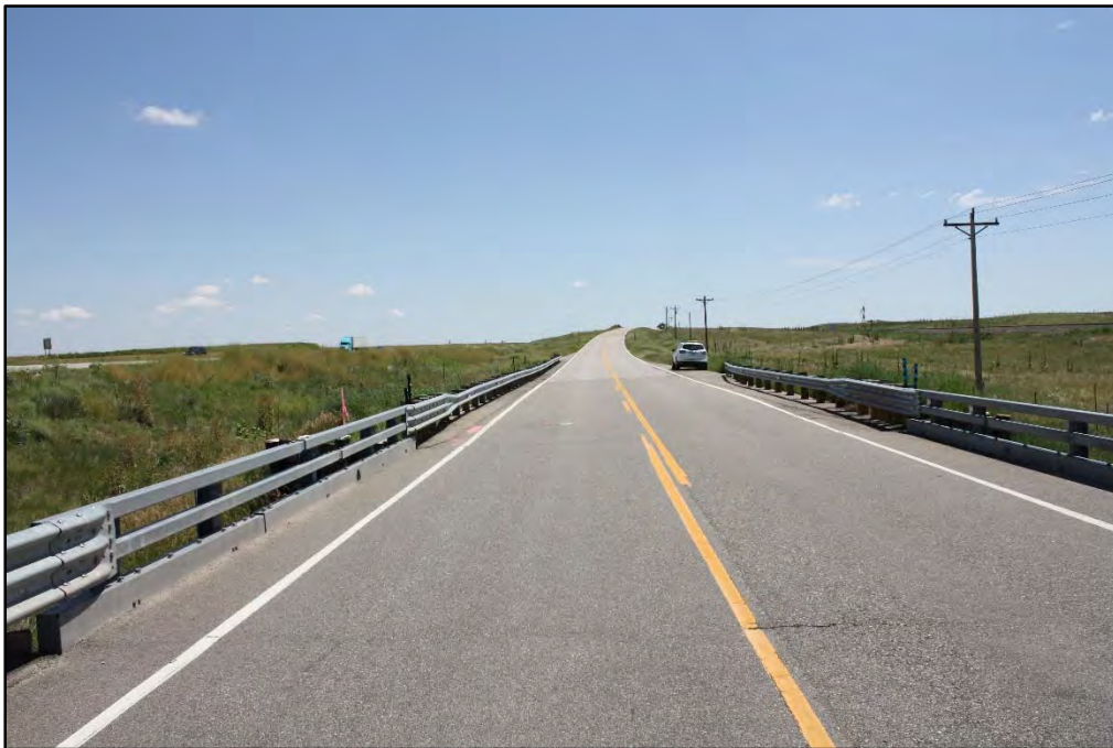
Photograph 6. Bridge Deck Looking Southeast
