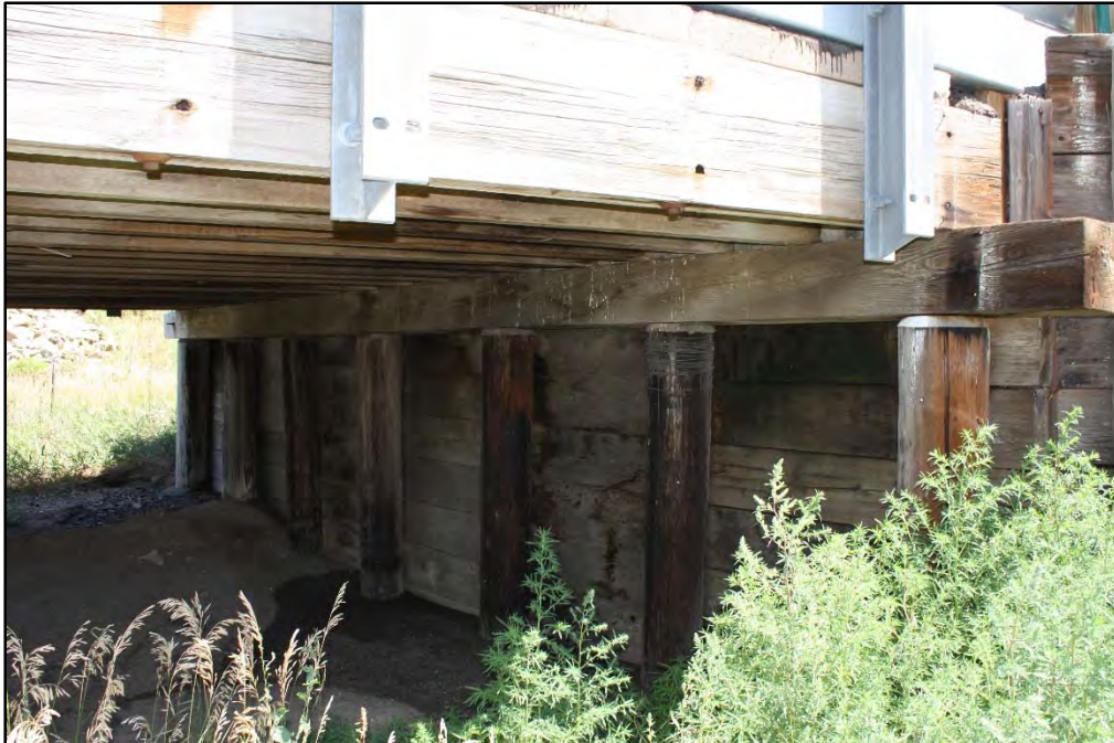
Photograph 10. East Abutment Backwall (Upstream) Looking East
