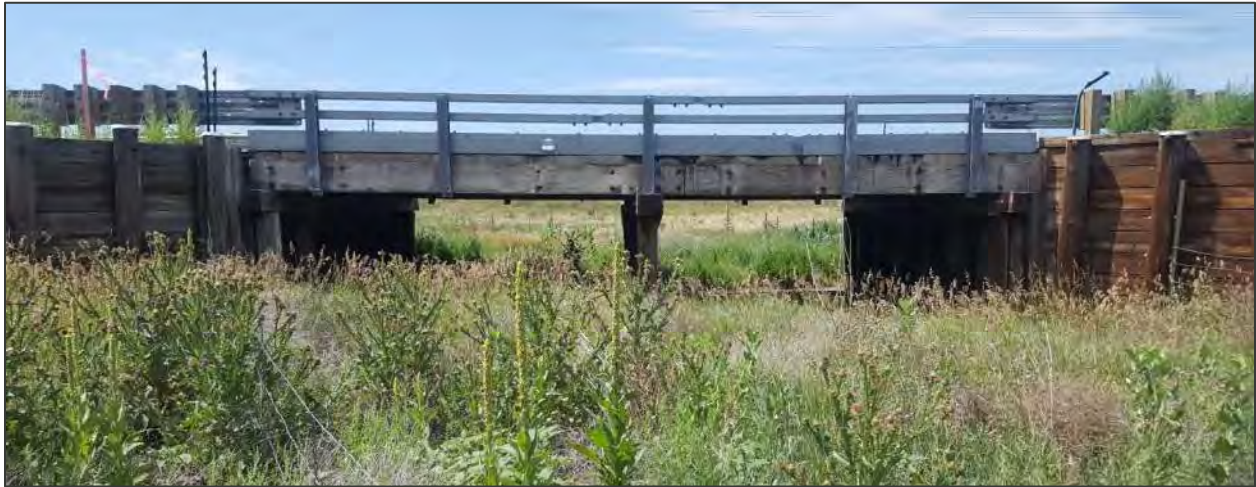
Figure 3. View looking upstream at US36 Bridge F-20-L near Peoria, CO.
