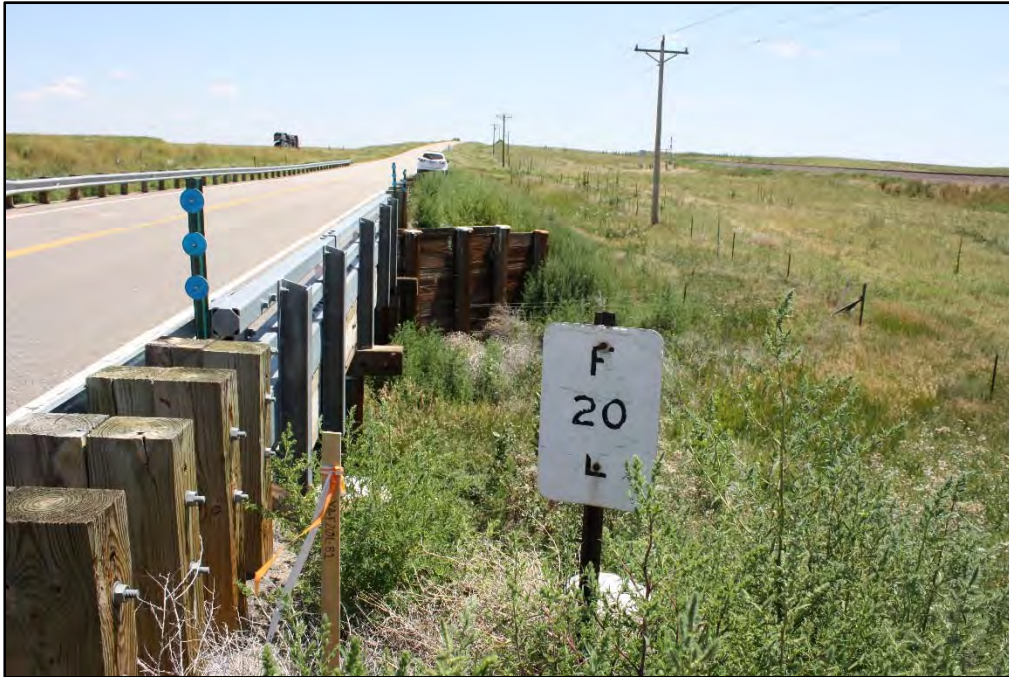
Photograph 3. Upstream Embankment Looking Southeast
