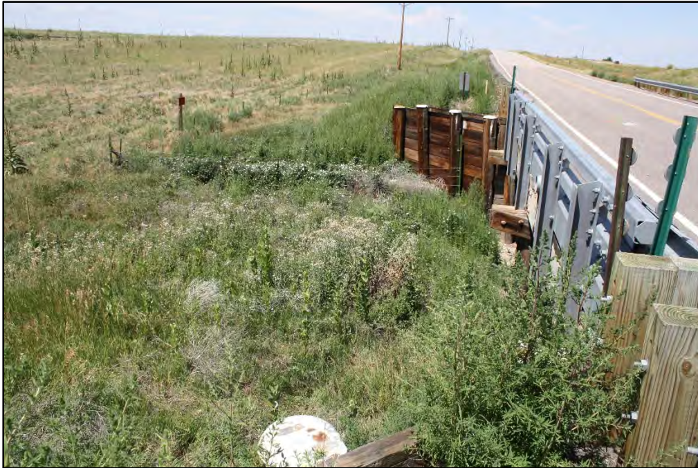
Photograph 1. Upstream Embankment Looking Northwest
