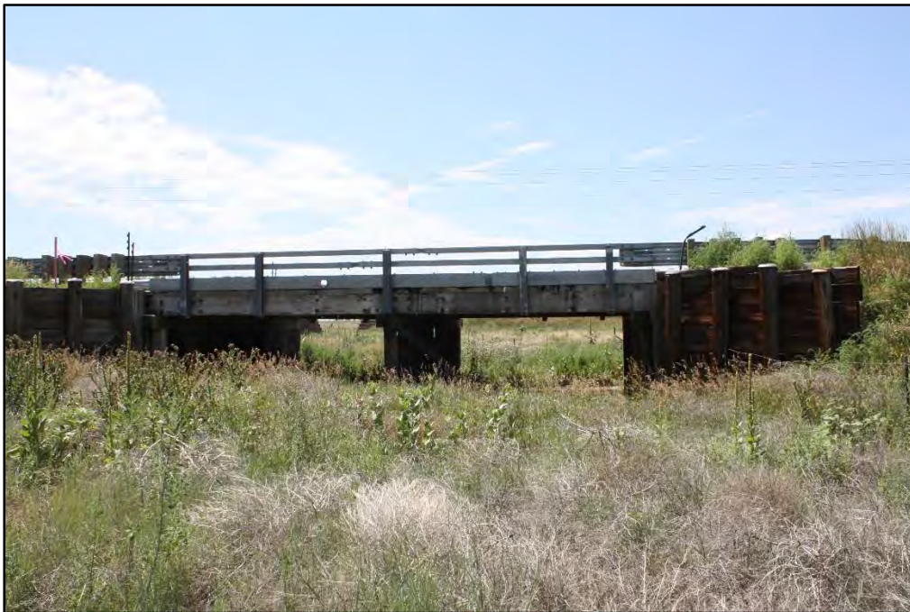
Photograph 8. Downstream Bridge Face Looking Southwest
