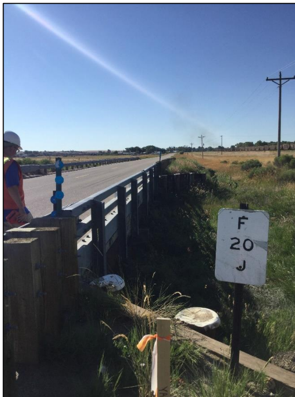
Figure 4: Upstream face of Bridge F-20-J, looking northwest along roadway
