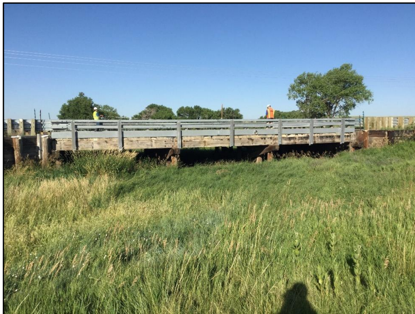
Figure 2: Upstream face of Bridge F-20-J
