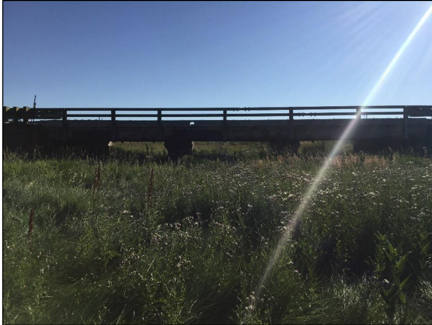
Figure 3: Downstream face of Bridge F-20-J
