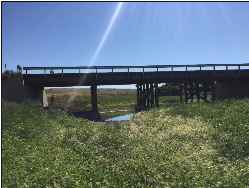
Figure 3: Downstream face of Bridge G-21-A
