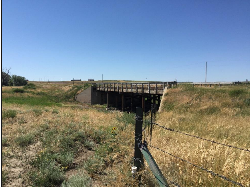
Figure 4: Upstream face of Bridge G-21-A, looking south along roadway
