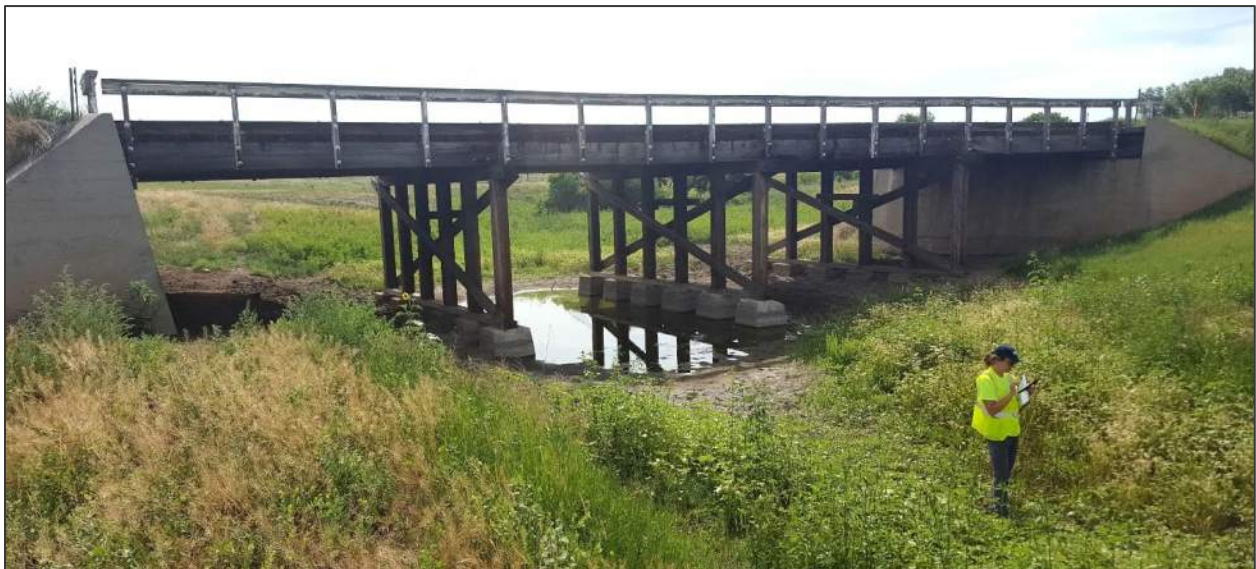
Figure 3. View looking downstream at US36 Bridge G-21-A over Agate Creek.
