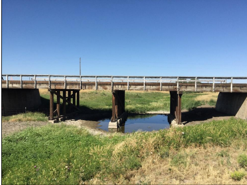
Figure 2: Upstream face of Bridge G-21-A
