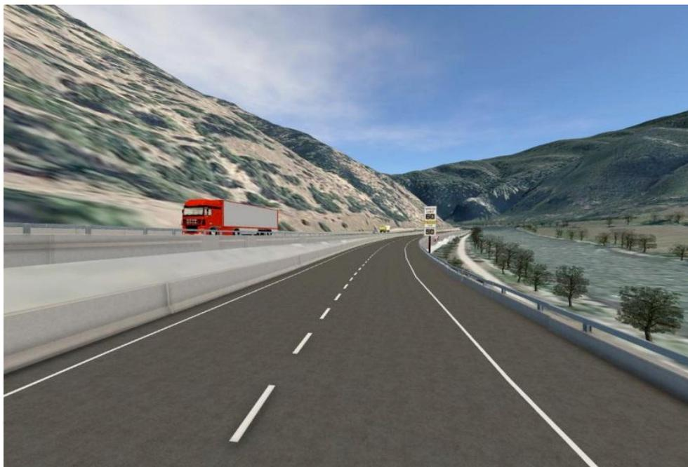
This 3d model image was used to evaluate the sign location from multiple vantage points and shows the approximate location of the relocated sign.
