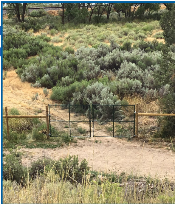
Double drive access gates along wildlife fencing.
