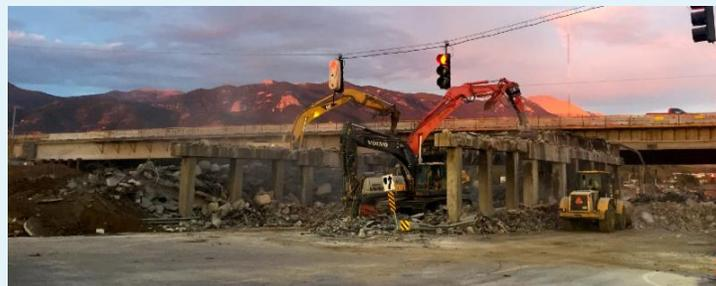
The I-25 bridge crossing over Cimarron Street/US 24 is the largest bridge demolished on the I-25/Cimarron Interchange Design-Build project. The ability to temporarily close Cimarron Street/US 24 under the interstate for quick demolition saved what would otherwise have required several weeks (2-3) of overnight closures had the old bridge been removed in pieces. Not only that, but implementing a full weekend closure resulted in a much safer operation and guaranteed quality work.
