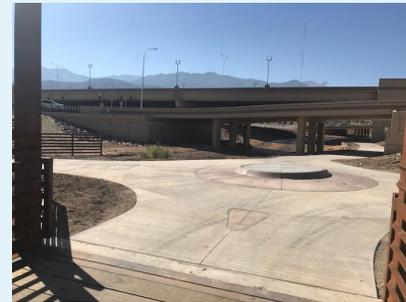
Concrete retaining wall panels with designs reflecting native fish in their habitat were installed along the new Midland Trail directly under I-25 bridges and along the Pikes Peak Greenway Trail under the Cimarron Bridge.
