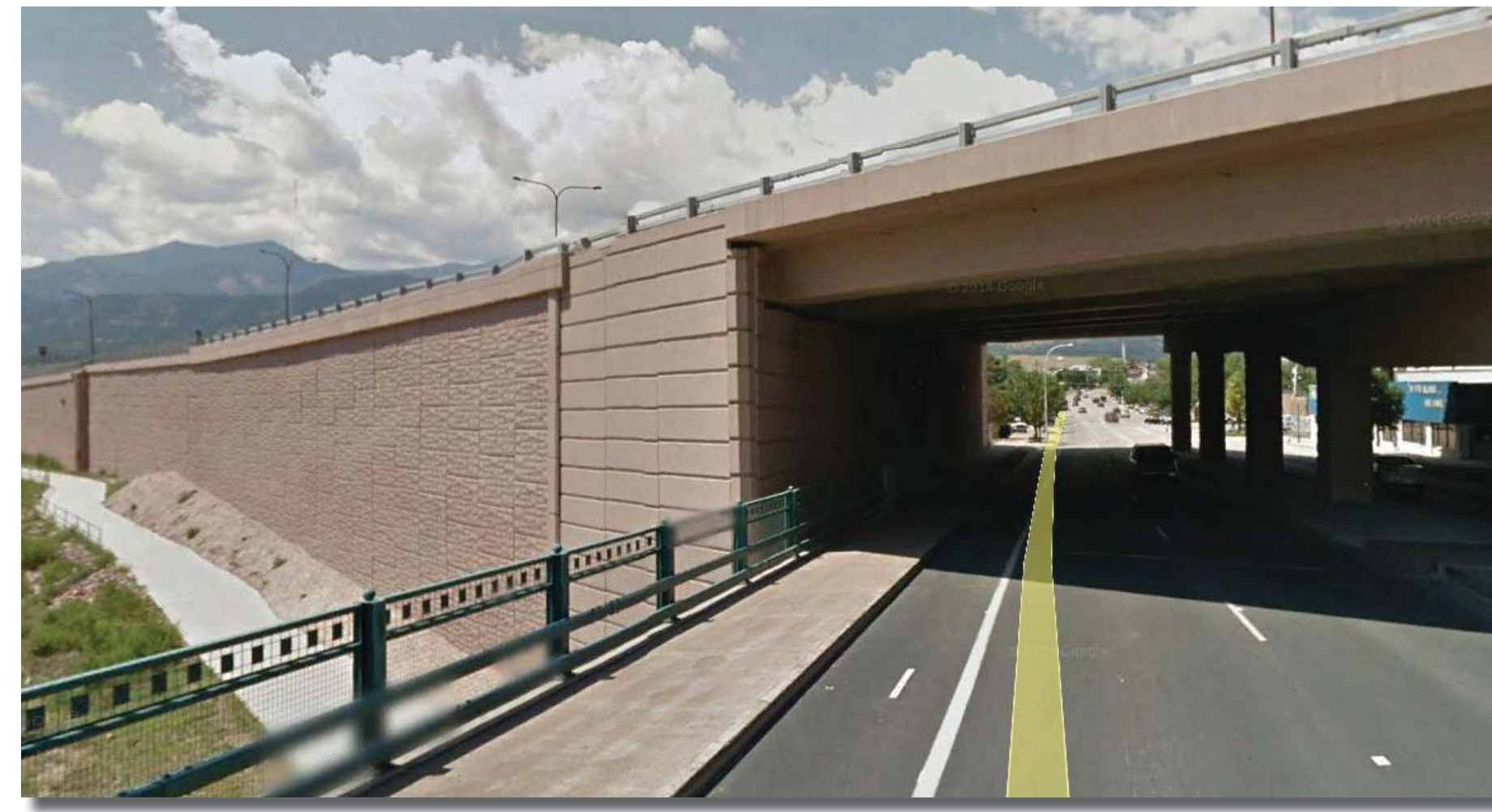
WALL TEXTURE/DESIGN ON EAST SIDE OF I-25 EXISTING WALLS NORTH OF PROJECT. I-25 WALLS WILL MATCH THESE, EXCEPT FOR ENHANCEMENTS AS SHOWN ON THIS BOARD
