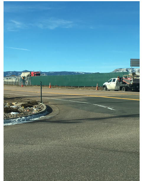
Headlight glare mitigation devices were set up on northern section frontage roads.
