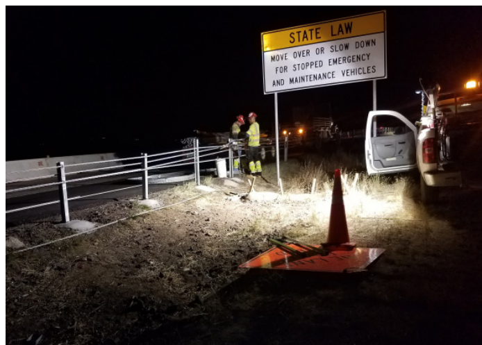
Crews performing overnight repairs of guardrail following vehicle crash
