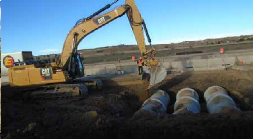
Drainage work in the north section
