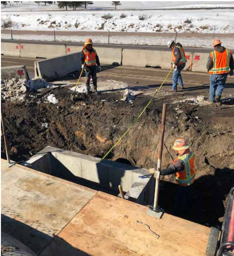
Crews install drainage inlets.
