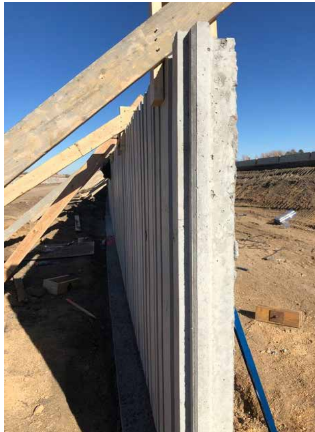
Median walls in the north section
