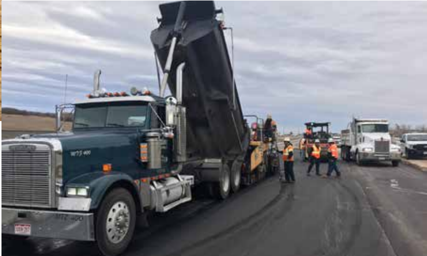
Paving in the north section
