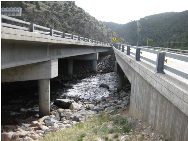
Figure 20. I-70 and eastbound ramp bridges
