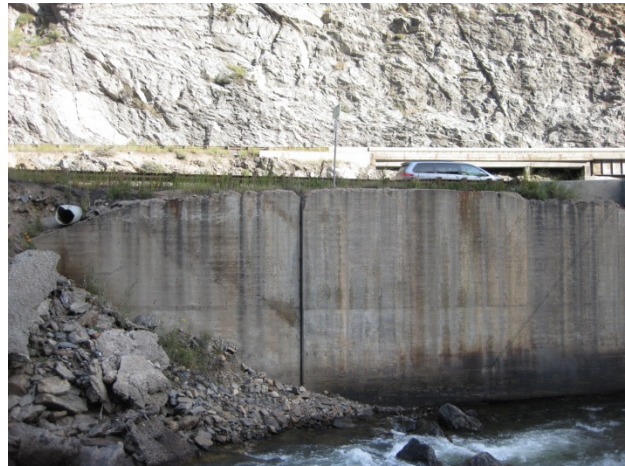
Figure 27. North abutment wing-wall
