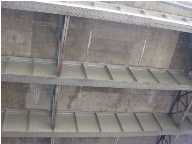
Figure 36. Bottom of bridge deck
