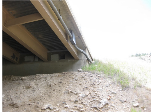
Figure 6. Girders and cross bracing
