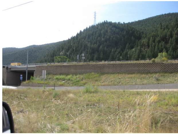
Figure 15. MSE wall on northwest corner
