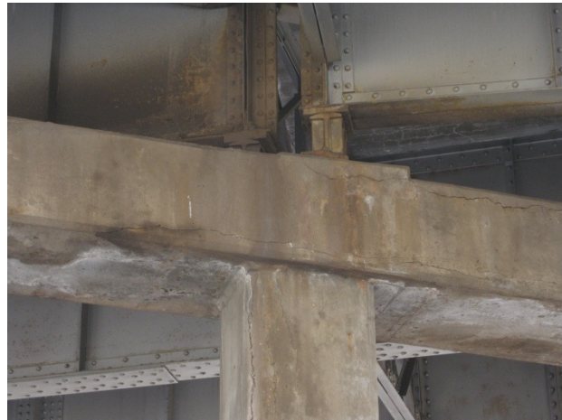
Figure 37. Pier below expansion device
