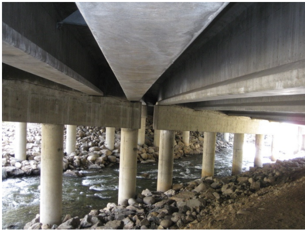
Figure 18. Pier bent looking east
