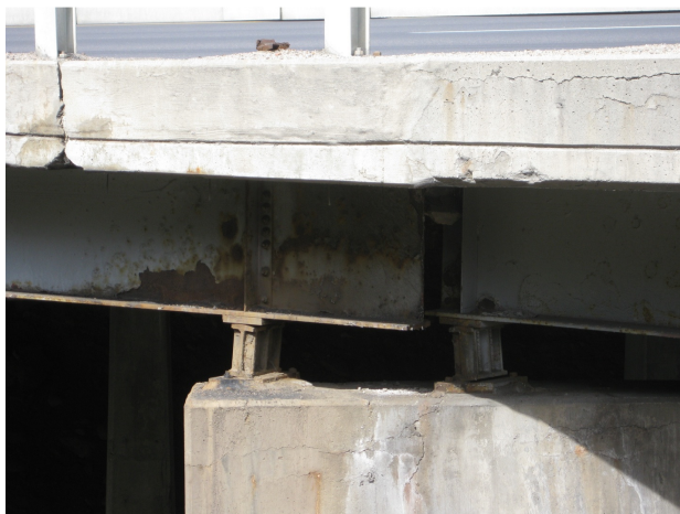
Figure 12. Bearings in pier
