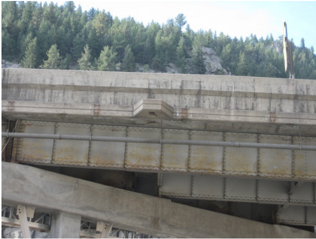
Figure 38. North side bridge rail and deck
