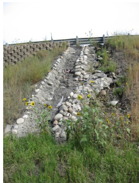
Figure 17. Southwest riprap rundown
