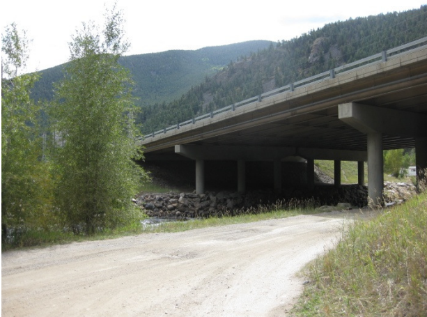
Figure 5. Access road below the bridge
