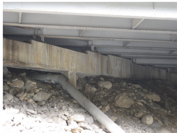
Figure 13. Drain pipe near west abutment
