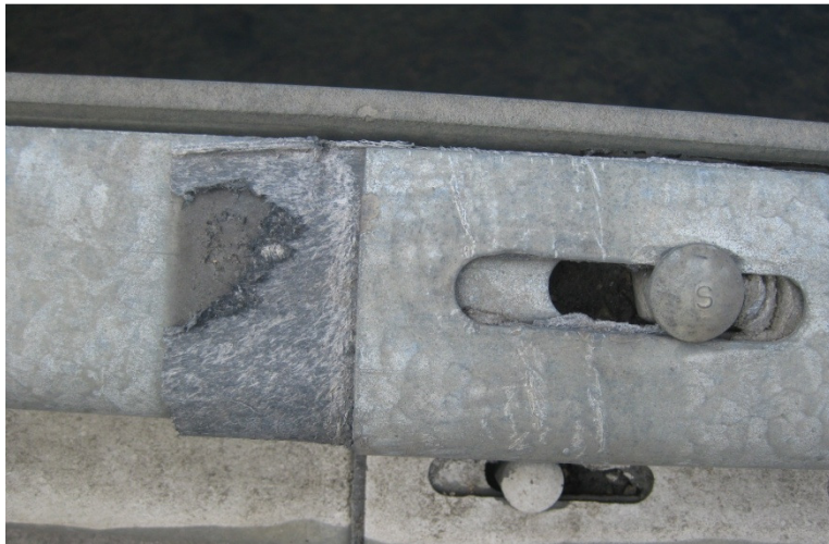
Figure 9. Bridge rail expansion joint
