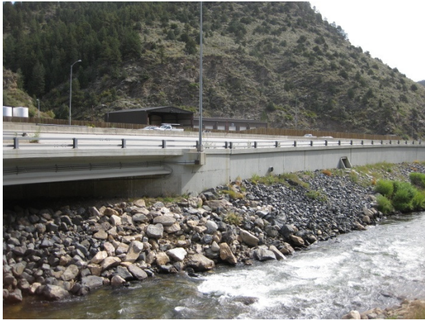
Figure 22. Retaining wall with box culvert
