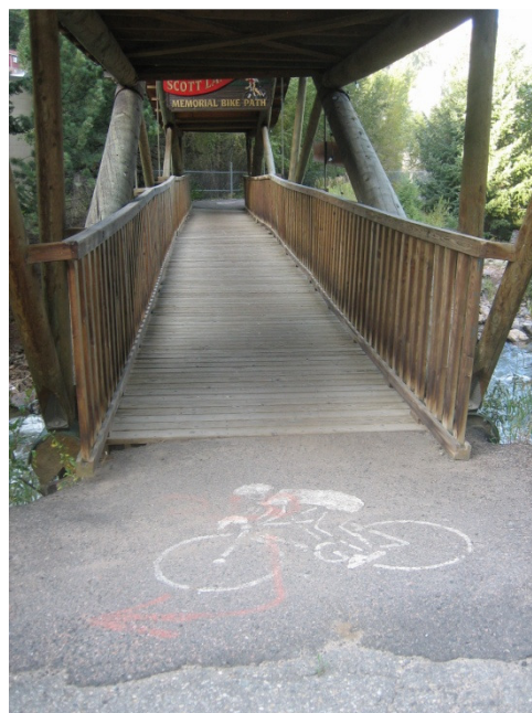
Figure 49. Bicycle path pavement markings
