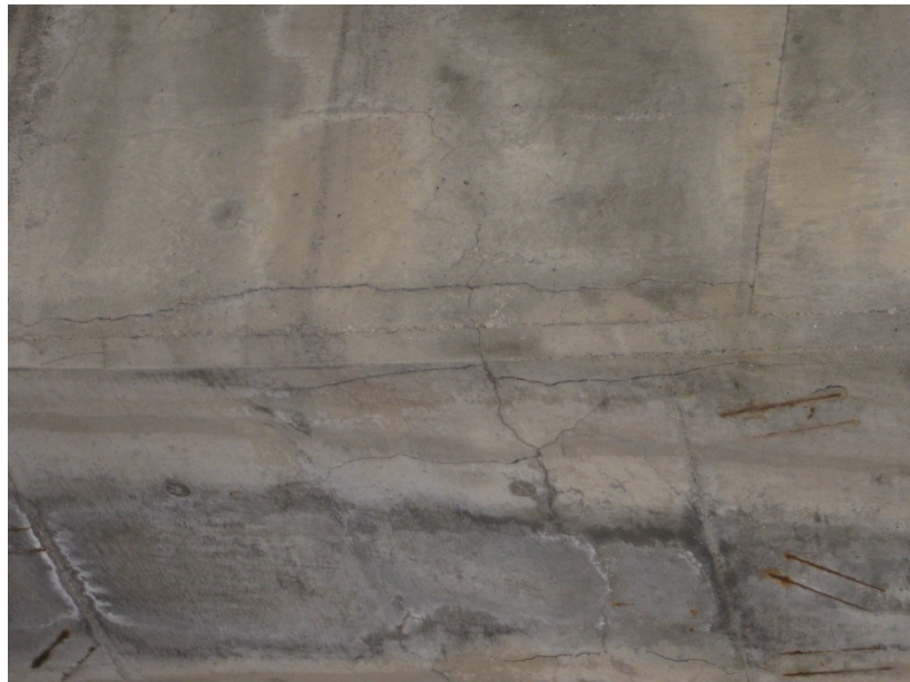
Figure 31. Bottom of pier cap
