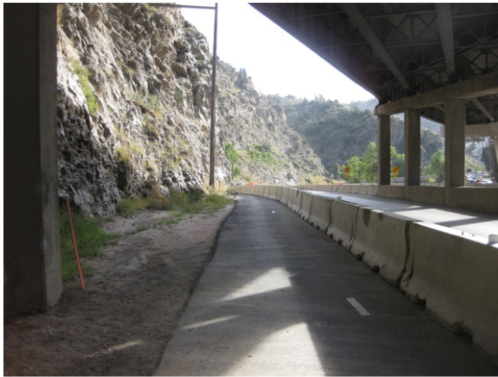
Figure 41.US 6 ramp below I-70
