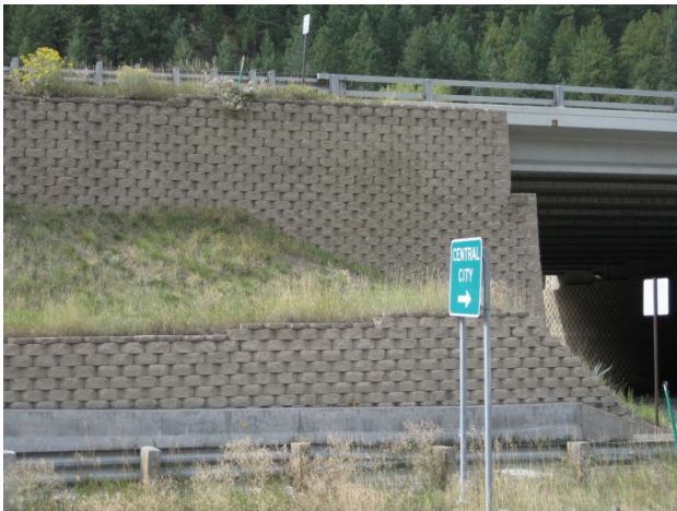
Figure 14. Tiered MSE wall on northeast corner
