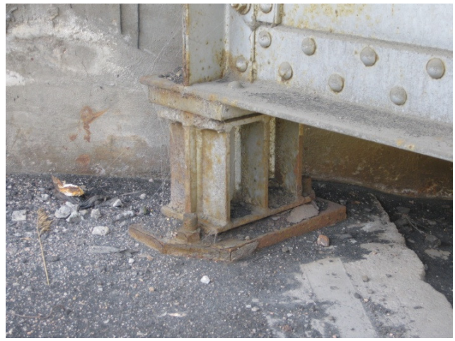
Figure 39. South abutment bearing
