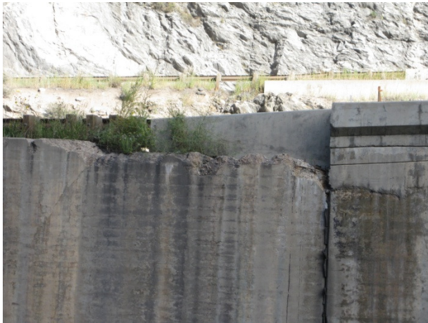
Figure 26. Top of pier wall
