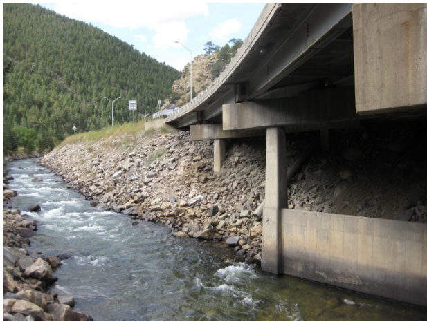
Figure 7. Bridge looking west
