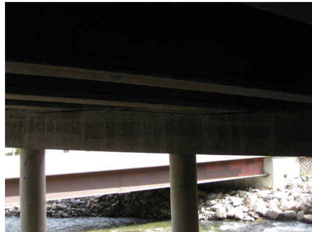
Figure 21. Westbound ramp bridge
