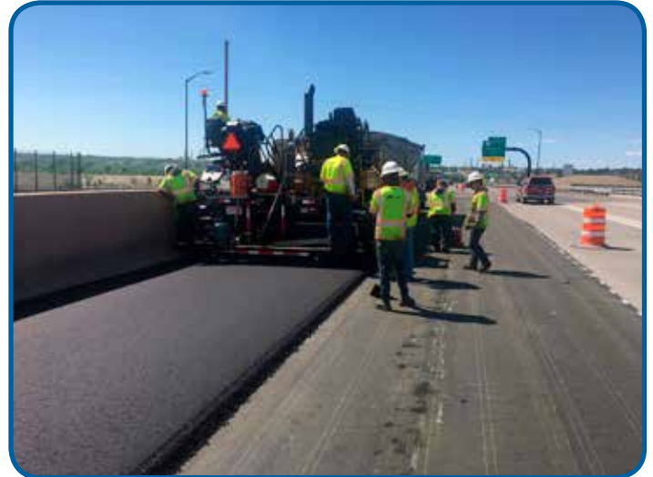
Asphalt crews lay down the final top mat
