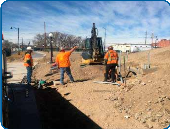
Installing permanent lighting services on D Street
