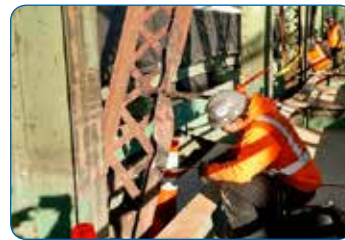
US 50 C Green Truss Bridge heat straightening before and after
