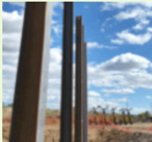
Steel H pilings installed to support D Street walls
